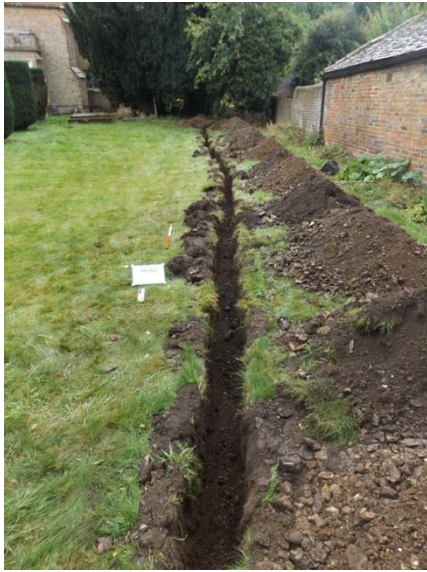
Plate 1: Pipe trench, facing south
