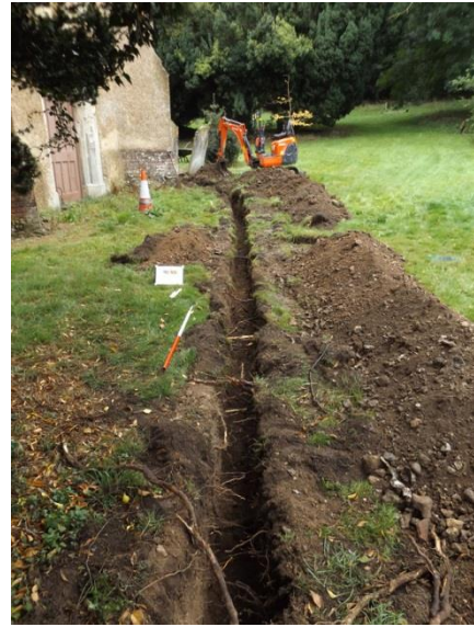
Plate 2: Pipe trench, at western end of church
