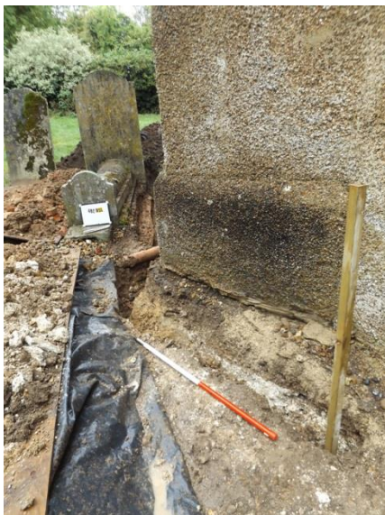
Plate 3: Pipe trench, rear of church tower
