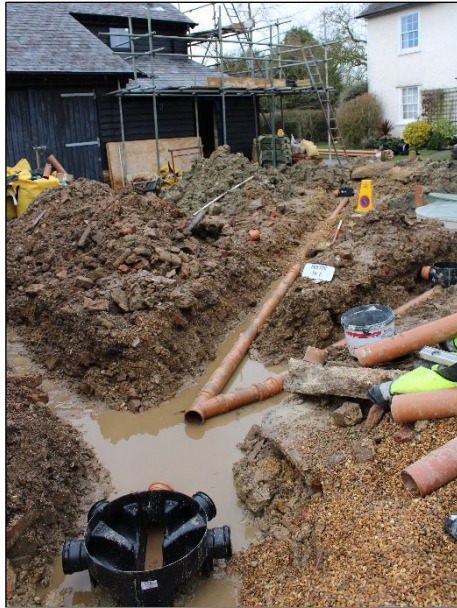
Plate 5: Trench 2 layout B, looking north
