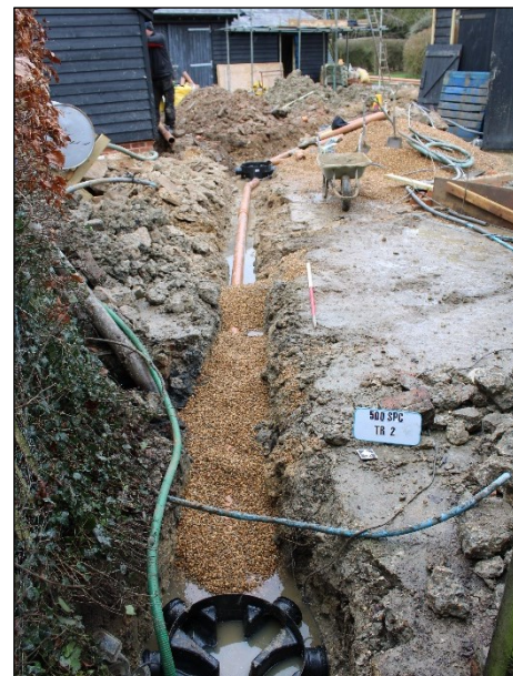
Plate 3: Trench 2 layout A, looking north
