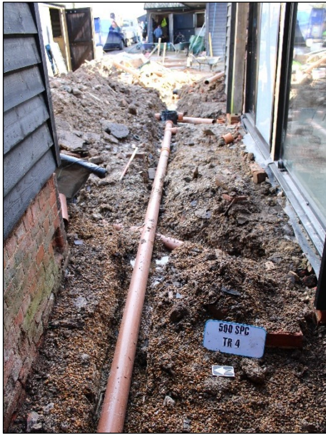
Plate 9: Trench 4 layout, looking east
