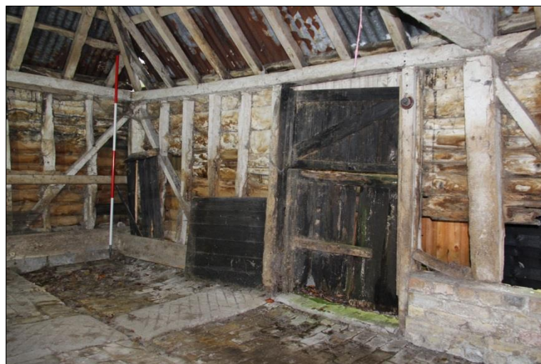
Plate 15: West end: northwest corner
