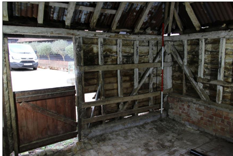
Plate 5: East end: northeast corner
