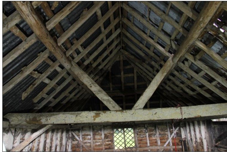
Plate 13: West end: truss
