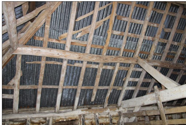
Plate 10: East end: view of the roof from the northeast
