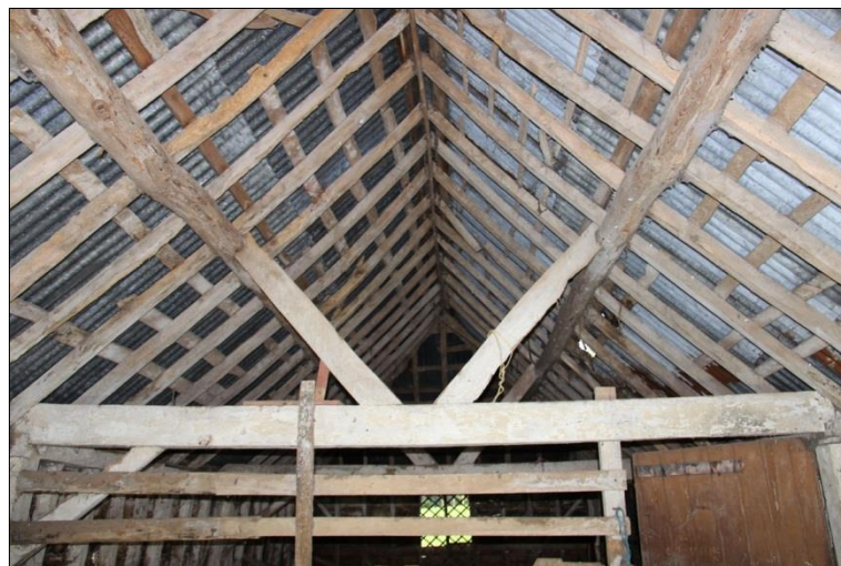
Plate 8: East end: truss over the partition
