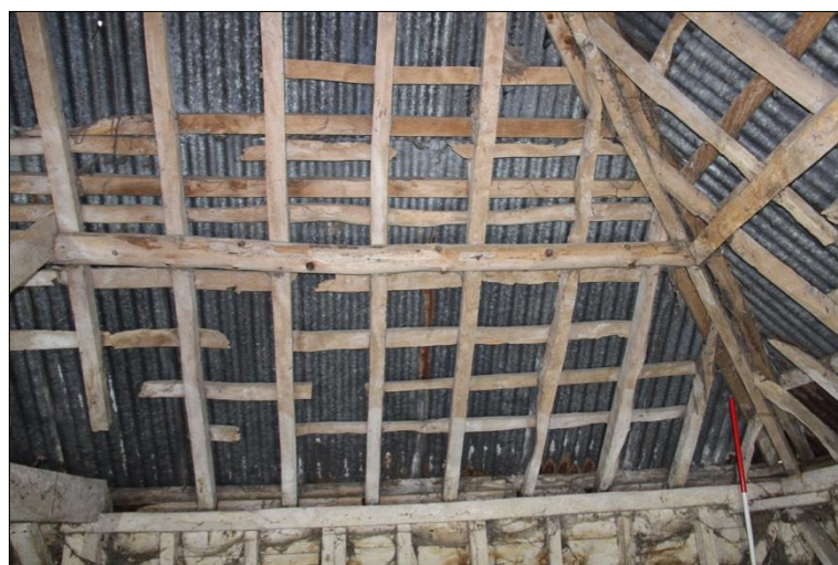
Plate 18: West end: roof above western end of the south wall
