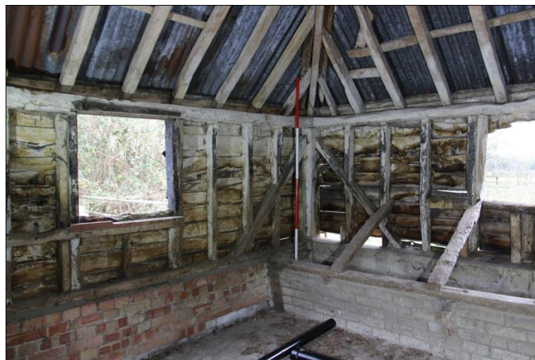
Plate 11: East end: southeast corner
