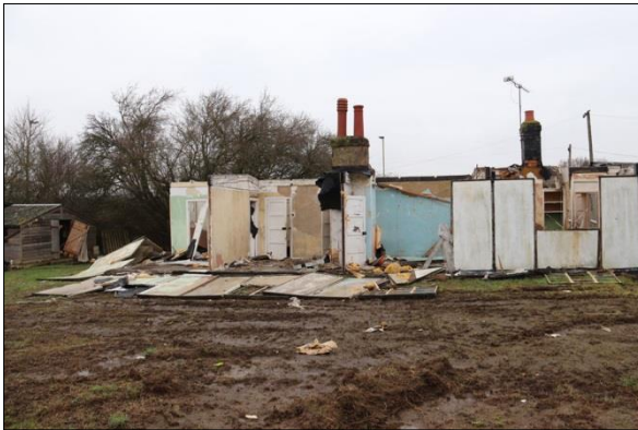
Plate 5: South elevation: west end (17)
