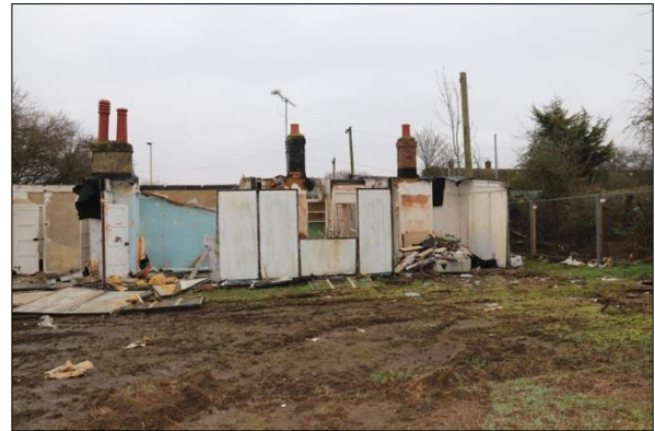
Plate 6: South elevation: east end (18)
