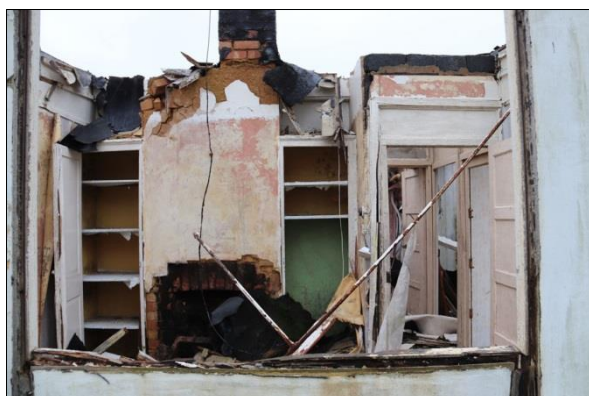
Plate 16: Room G4 from the south (12)
