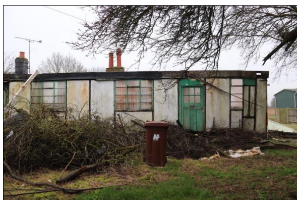
Plate 3: North elevation: west end (3)
