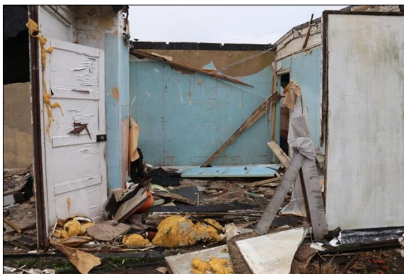
Plate 13: Room G3 from the south (9)
