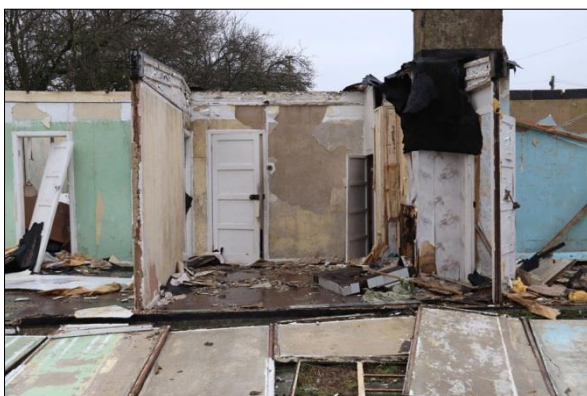
Plate 10: Room G2 from the south (6)
