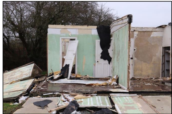
Plate 9: Room G1 from the south (5)
