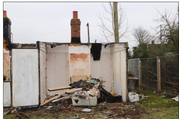
Plate 20: Room G5 from the south (15)
