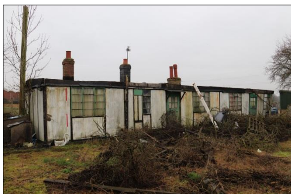
Plate 1: North elevation from the northeast (1)
