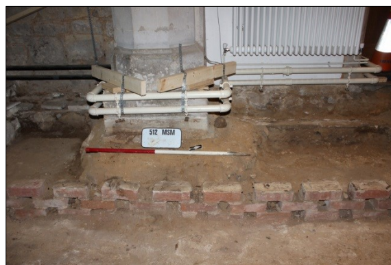
Plate 17: West column foundations, south aisle, view west
