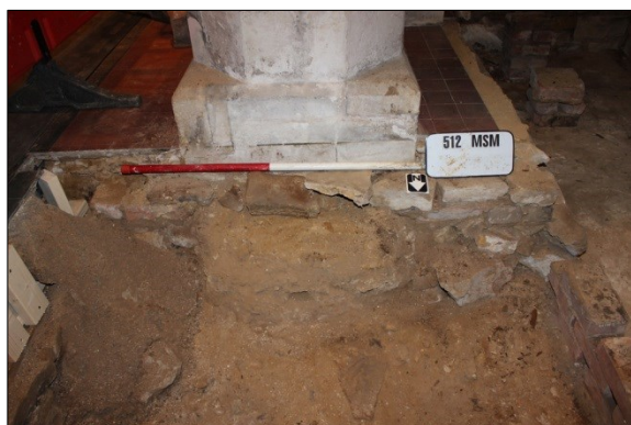
Plate 16: East column foundations, south aisle, view south
