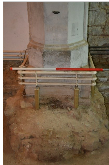
Plate 13: West column foundations, north aisle, view west
