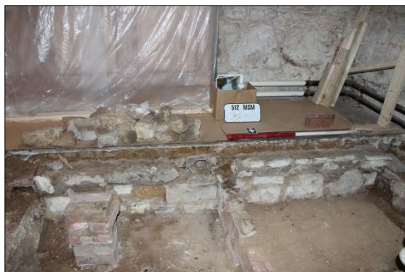
Plate 14: South section of excavation, south aisle
