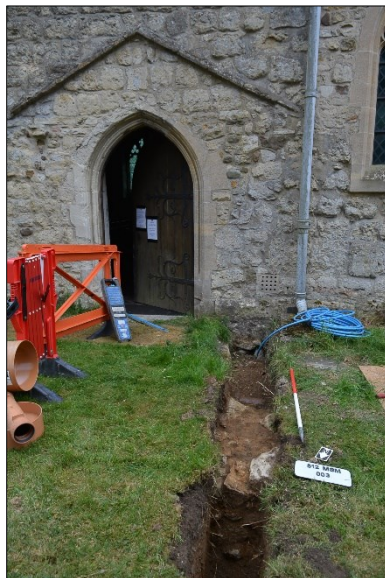
Plate 6: Foundation [003] in relation to existing entrance and roof 'scarring', view south-southeast
