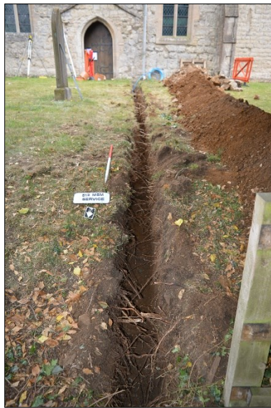
Plate 1: Service trench overall, view south-southeast
