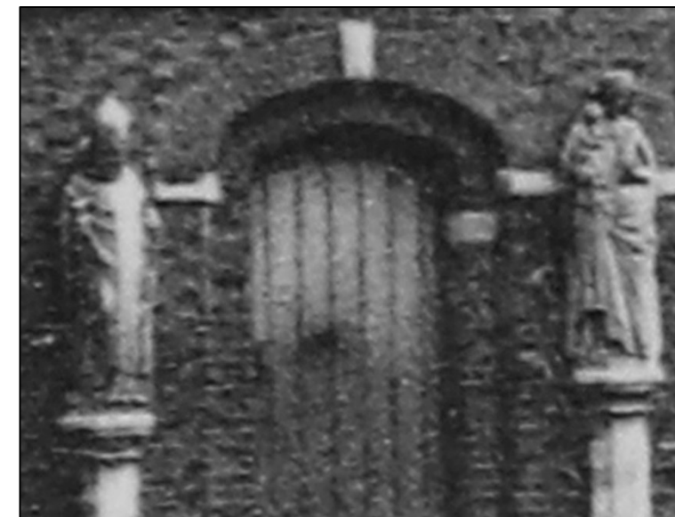
The replacement Madonna and Bishop on the Old Town Hall plinths post 1910 (21306/72/11/5)
