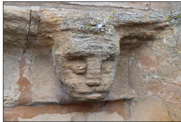
Banded weathering (Carstone)
