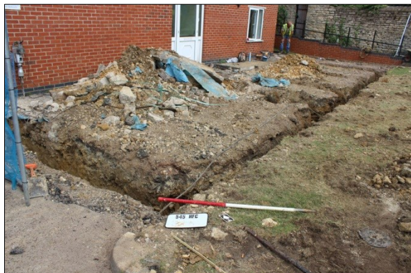
Plate 1: Trenches 1-5 overall, view NE
