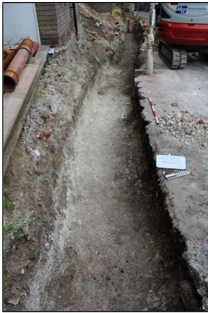
Plate 1: Trench 1, facing northwest
