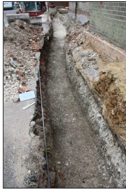
Plate 2: Trench 1, facing southeast
