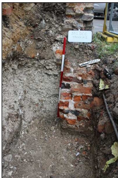
Plate 7: Trench 1, north-western end showing stub of the demolished wall, facing NW
