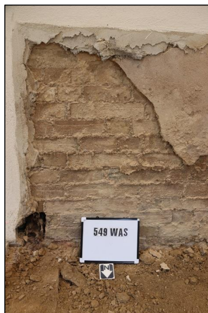
Plate 5: Detail of the brickwork in the south wall
