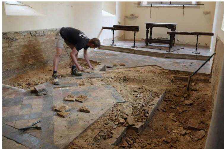
Plate 1: The tiles being removed
