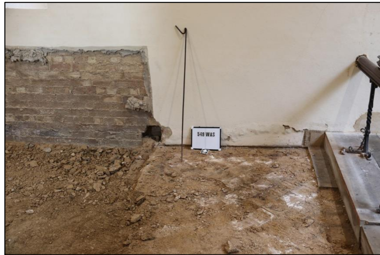
Plate 6: Floor reduction at the eastern end of the north wall
