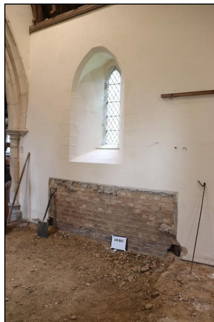
Plate 7: The lancet window and 19 th century brickwork in the north wall
