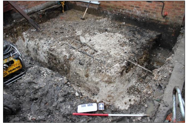
Plate 2: Rear extension - Footings trenches overall, facing north
