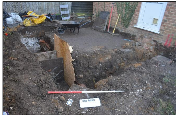
Plate 10: Front extension - Groundworks at the front of the property, facing southeast
