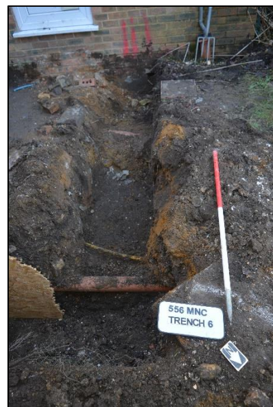
Plate 12: Front extension - Trench 6, facing southwest
