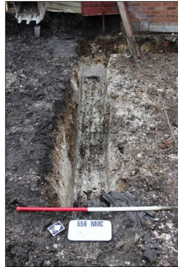
Plate 4: Rear extension - Trench 2, facing northwest
