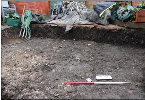
Plate 1: Rear extension - Ground reduction, facing south-southeast
