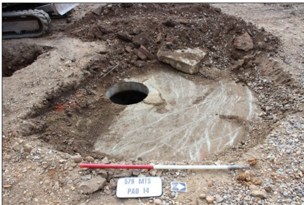
Plate 15: Concrete chamber in place of pad 14, looking west
