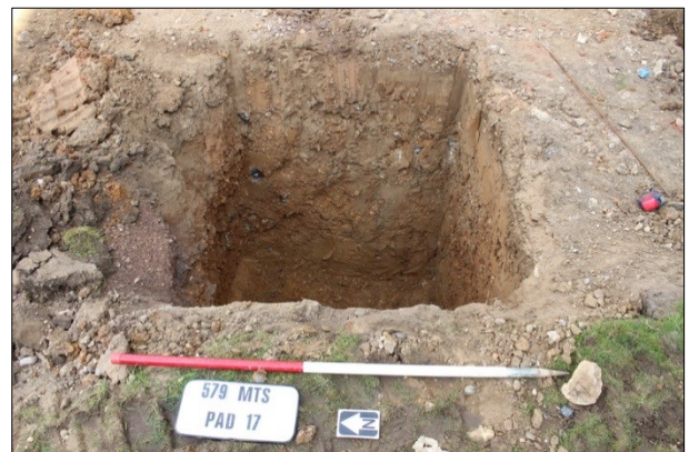
Plate 18: Pad 17, looking east
