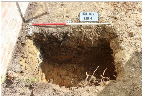
Plate 5: Pad 4, looking south
