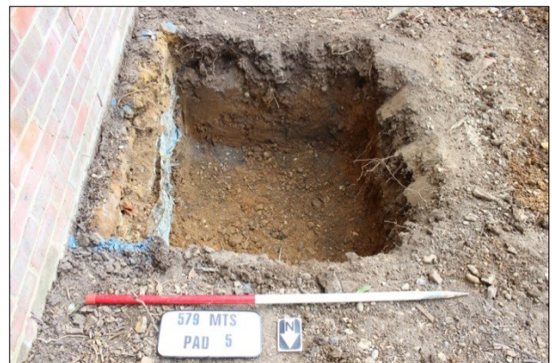
Plate 6: Pad 5, looking south
