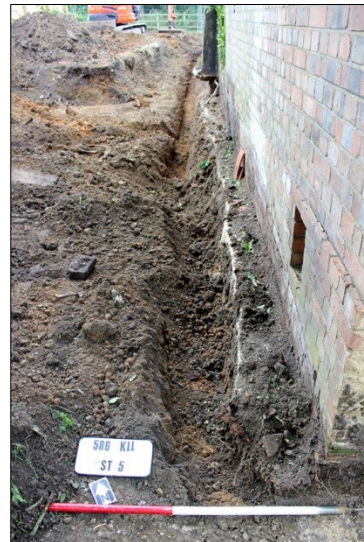
Plate 31: Service trench 5, view NE
