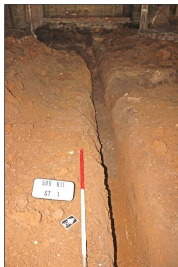
Plate 11: Service trench 1. View NW
