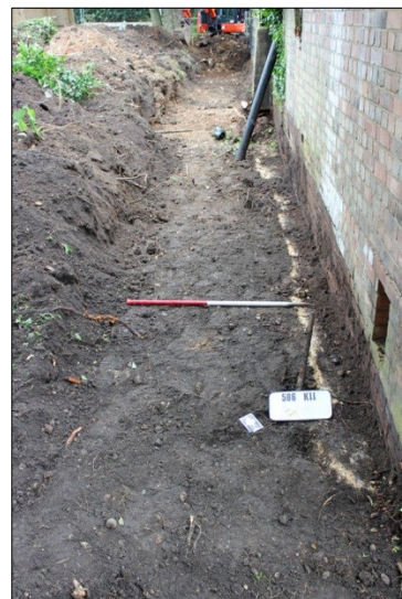
Plate 28: Exterior ground reduction along the length of the barn, view NE
