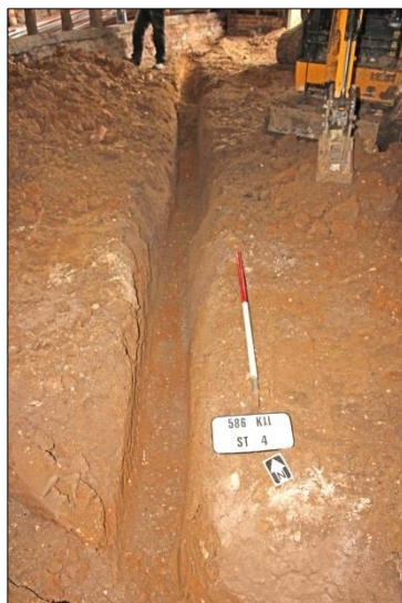
Plate 15: Service trench 4, view N
