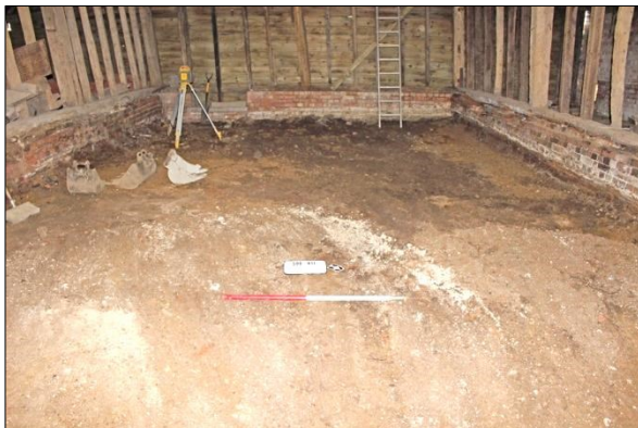
Plate 3: Main barn floor reduced, view SW
