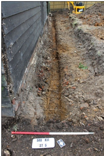
Plate 30: Service trench 5, view SW
