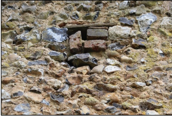
Shot 55: Putlog hole in west wall (upper level)
