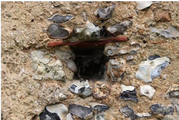
Shot 45: Putlog hole in west wall (upper level)
