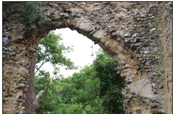
Plate 13: Voussoirs in the south wall (18)
