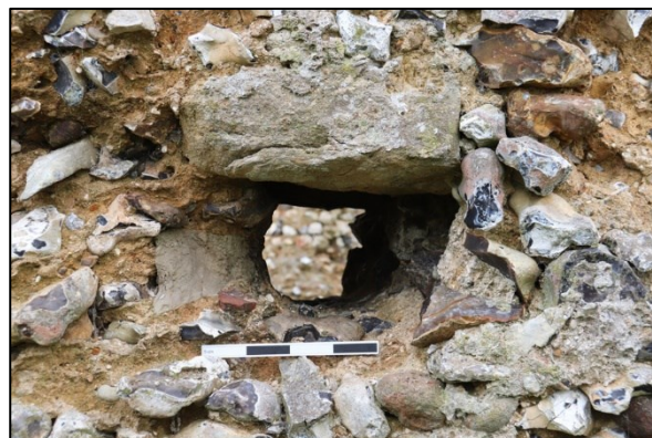
Shot 50: Putlog hole in south wall
