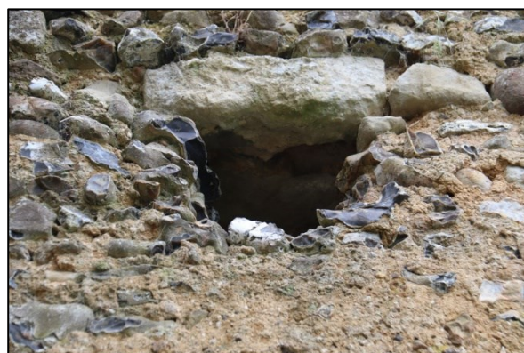
Shot 54: Putlog hole in west wall (above 52)
