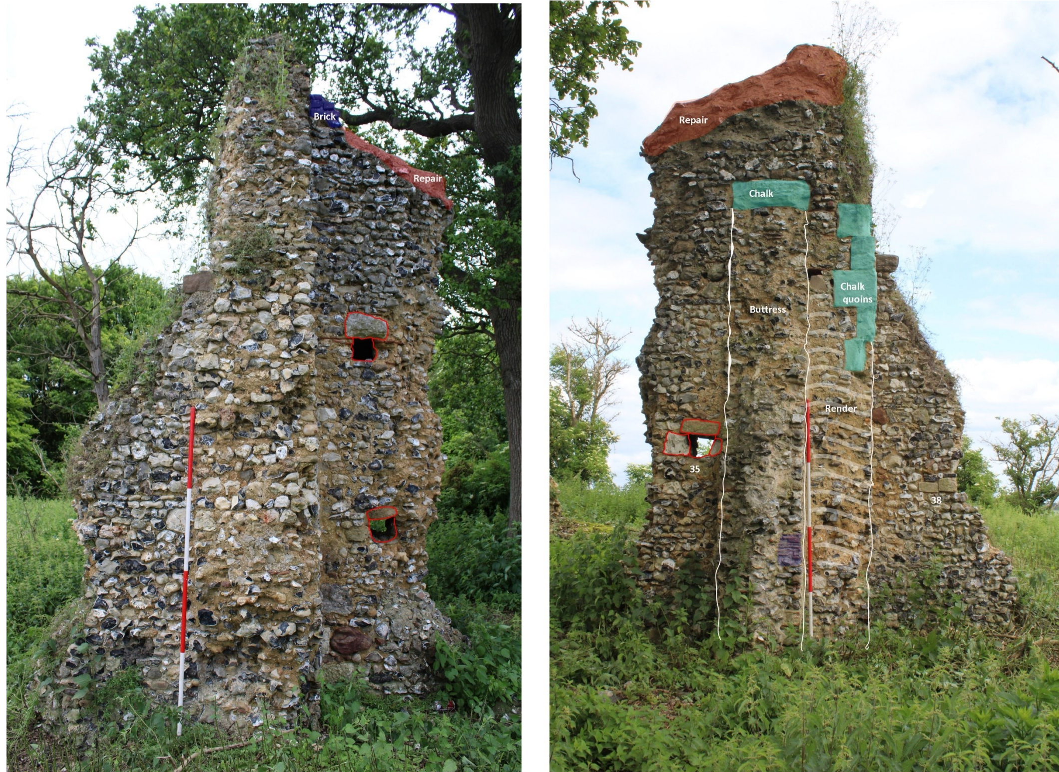
Figure 16: South wall, chancel end details (interior to left & exterior to right)
