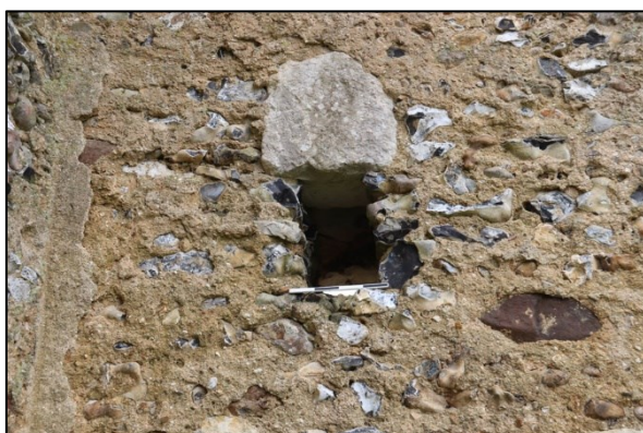
Shot 53: Putlog hole in west wall (above 51)
