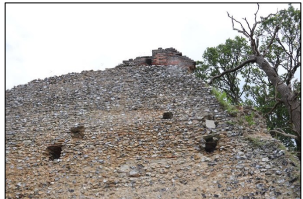
Shot 46: Top of west wall
