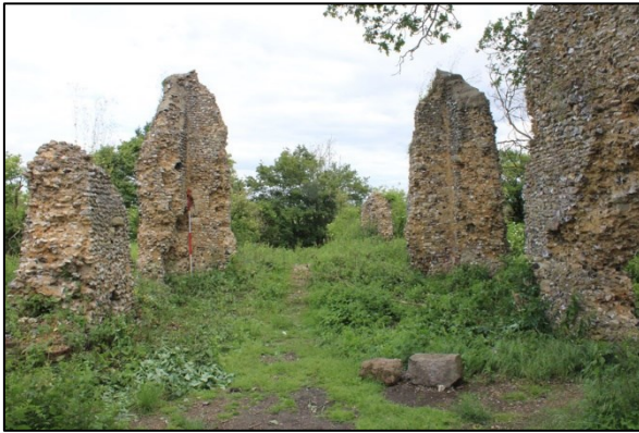
Plate 8: Interior view looking east (29)
