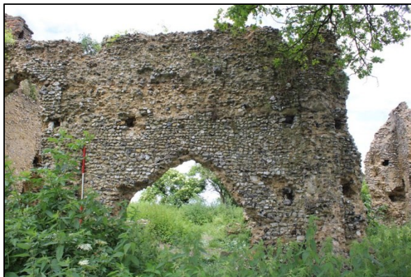
Shot 13: South nave wall
