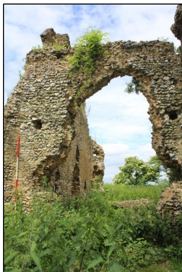
Shot 15: West end of south wall
