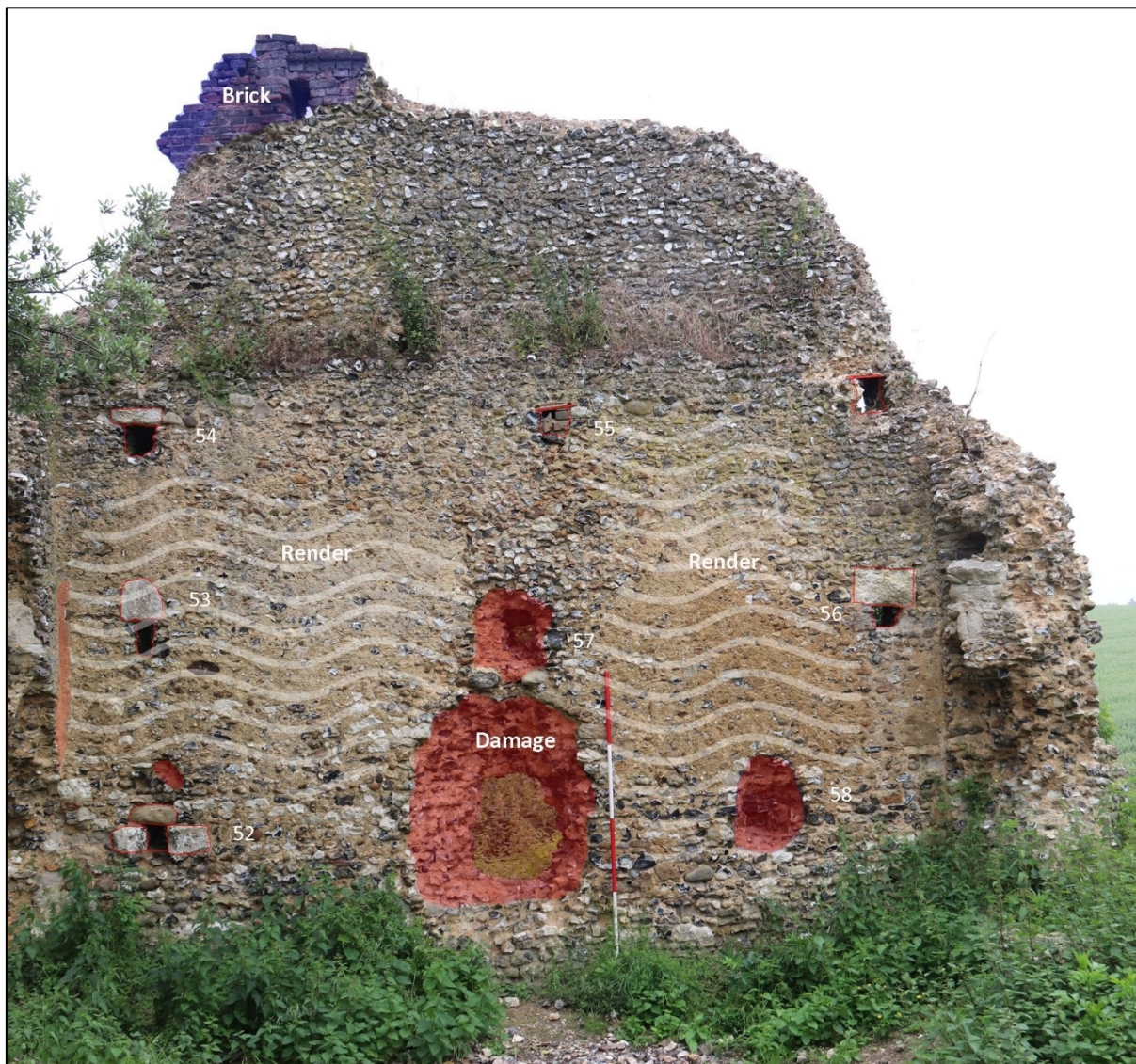
Figure 13: West wall details (interior)
