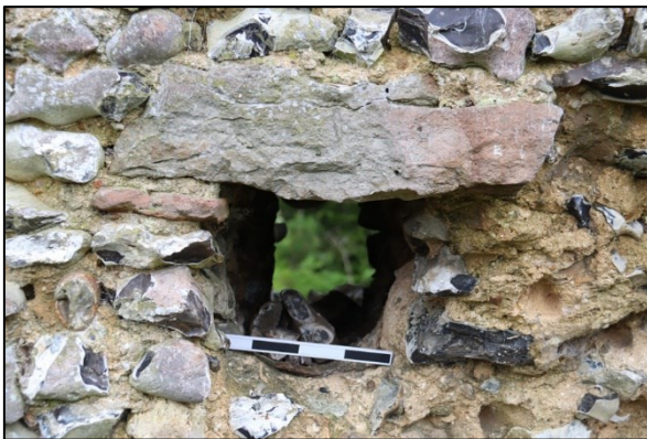
Shot 63: Lower putlog hole in freestanding section of south wall
