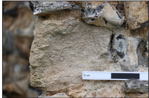
Plate 18: Detail of Barnack stone (40)
