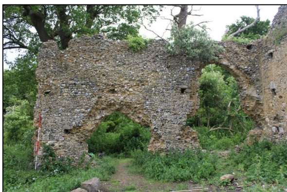
Shot 27: South nave wall
