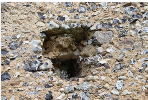
Shot 41: Putlog hole with lintel in west wall (middle level)
