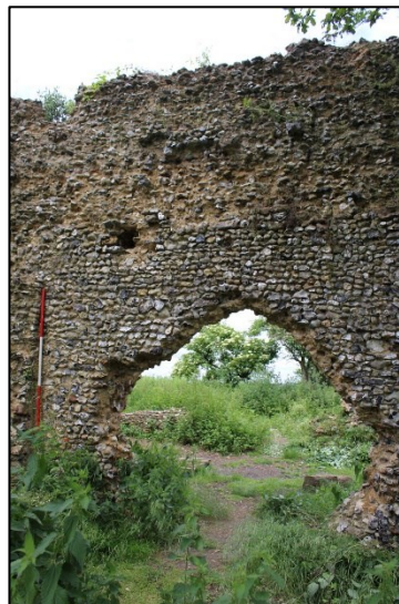
Shot 14: South nave wall
