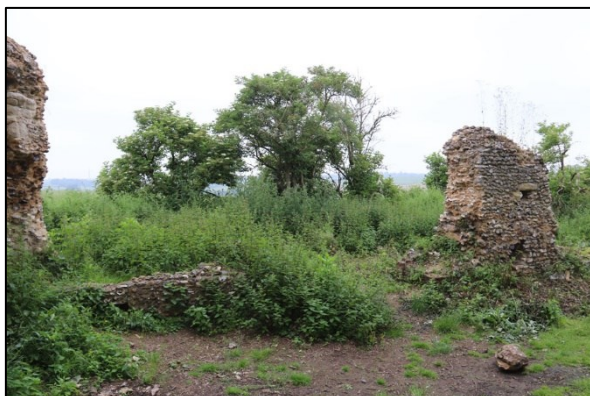
Shot 13: North wall of nave
