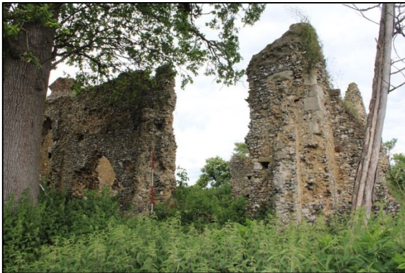
Shot 3: Southeast corner of the nave
