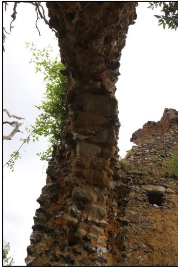
Shot 61: Stonework within window arch in south wall
