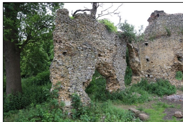
Shot 8: Southwest corner of the nave
