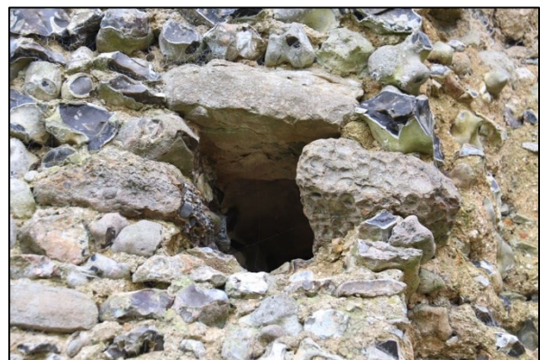
Shot 60: Putlog hole in south wall (middle level)
