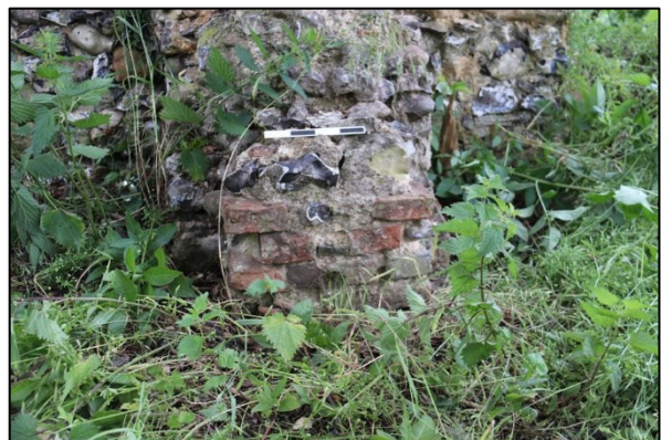
Plate 22: Floor tiles in southern buttress (32)
