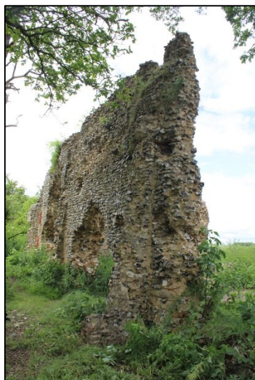
Shot 17: South wall
