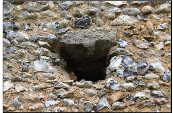
Shot 44: Putlog hole in west wall (middle level)
