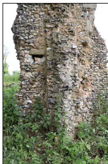
Shot 36: South chancel wall detail
