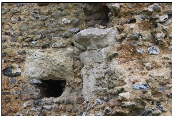
Shot 17: Remains of window tracery in north wall & putlog hole in west wall
