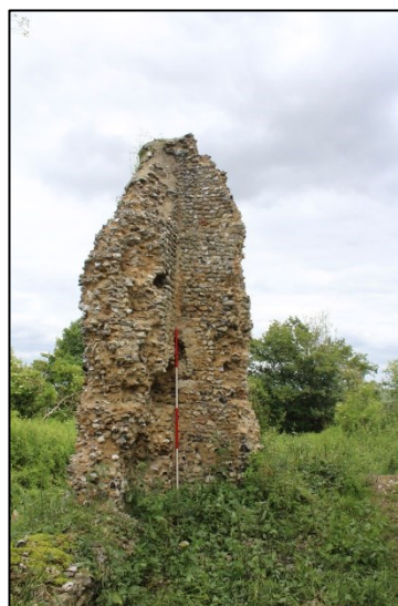
Shot 22: Northeast corner of nave
