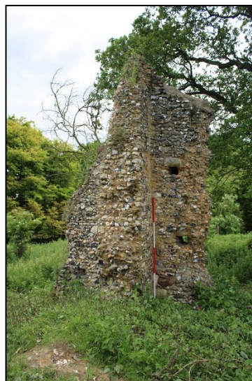
Shot 26: Southeast corner of chancel & nave
