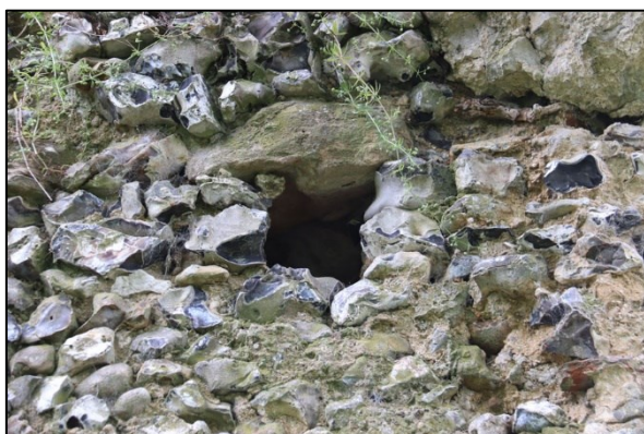
Shot 33: Putlog hole in south wall
