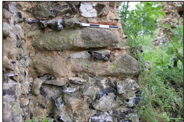
Plate 20: Sandstone in the south nave wall (34)
