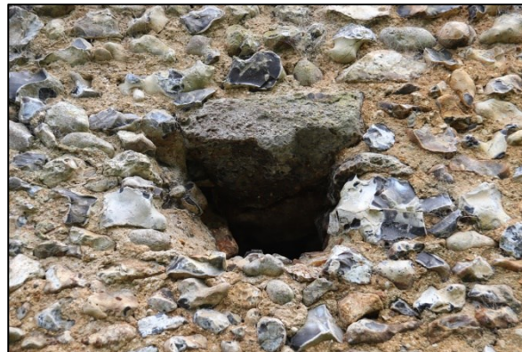
Plate 28: Moulded puddingstone lintel on exterior of west wall (44)
