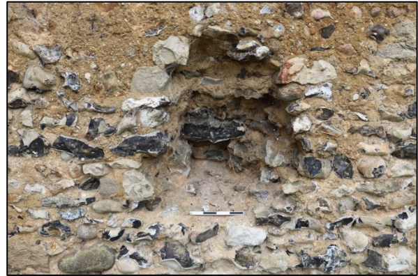
Shot 58: Recess/former putlog hole in west wall (lower level)
