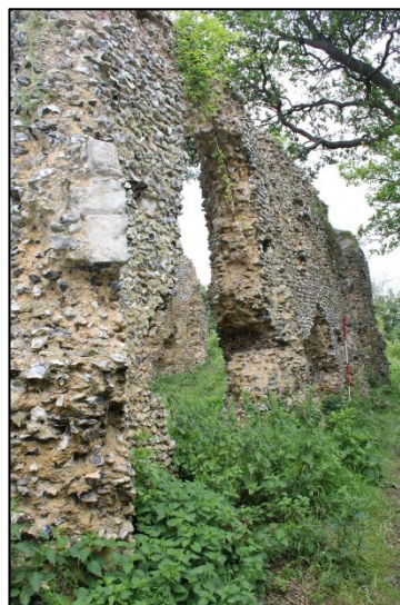
Shot 18: South wall
