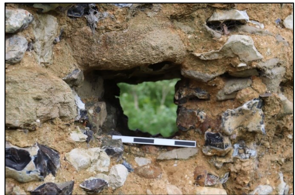
Shot 64: Upper putlog hole in freestanding section of south wall
