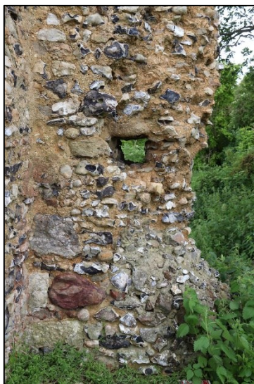
Shot 67: Detail of stonework in the freestanding section of south wall
