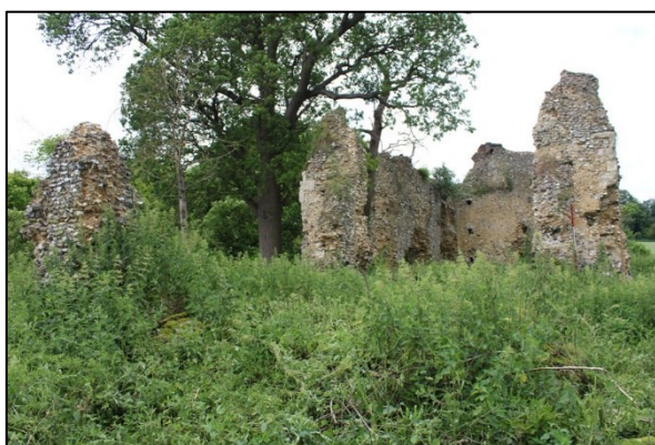
Plate 4: View from the northeast (1)
