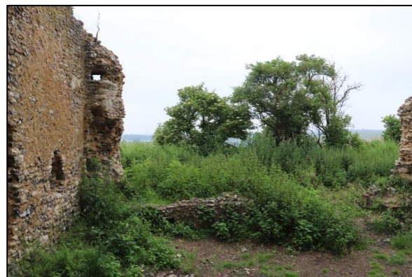
Shot 14: North wall of nave
