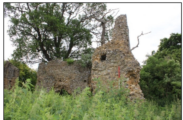
Shot 6: Northwest corner of the nave
