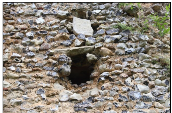
Shot 42: Putlog hole in west wall (upper level)
