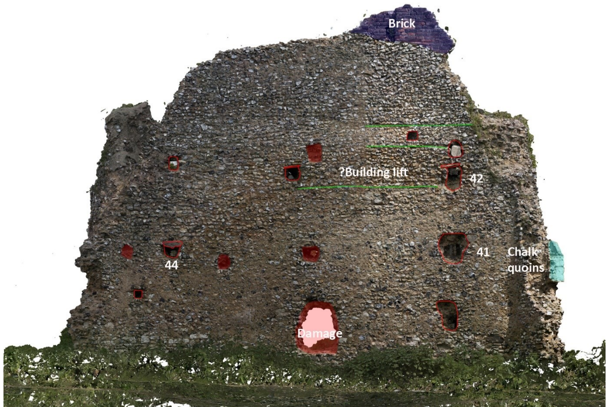
Figure 12: West wall details (exterior)
