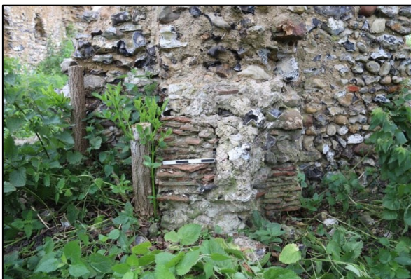
Plate 21: Tiles used in a southern buttress (31)
