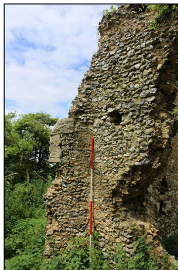
Shot 16: SE diagonal buttress
