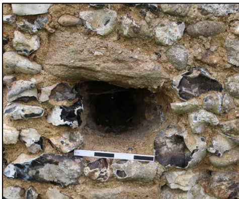
Shot 47: Putlog hole east end of south wall (lower level)
