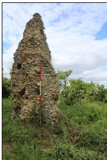
Shot 23: Northeast corner of nave
