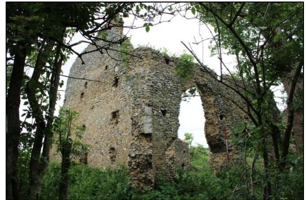
Shot 4: Southwest corner of the nave
