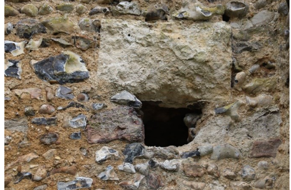
Shot 56: Putlog hole in west wall (middle level)
