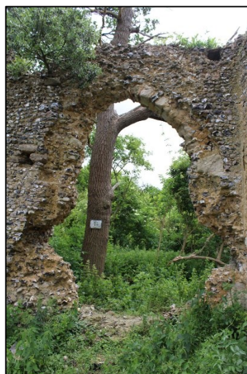
Shot 28: Window opening in south nave wall
