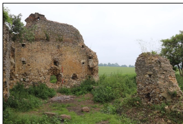
Shot 6: Northwest corner of the nave
