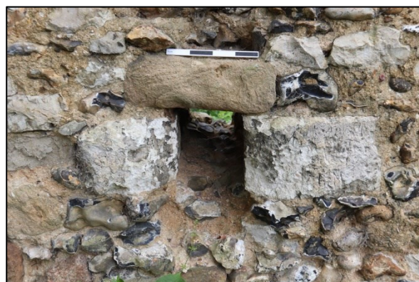
Shot 52: Putlog hole in west wall (lower level)
