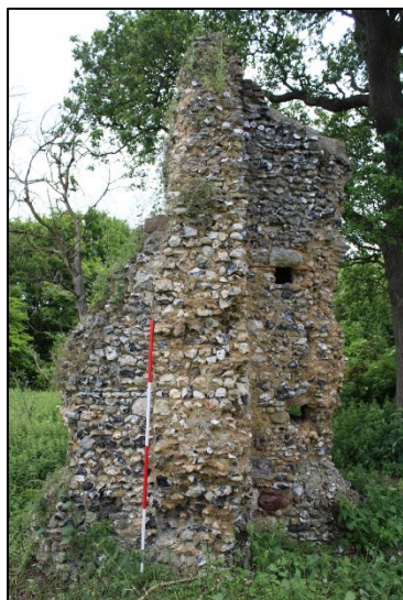
Shot 25: Southeast corner of chancel & nave
