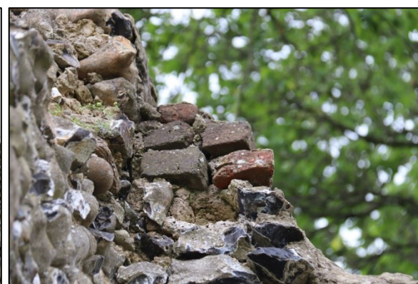
Plate 26: Brick repair work on south wall (66)
