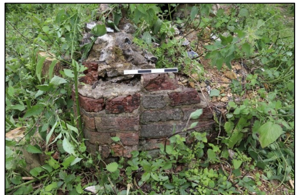
Shot 48: Brick base to door opening
