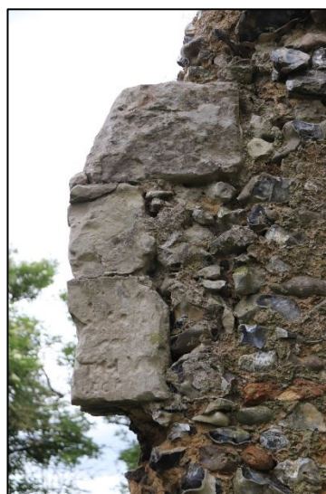
Shot 30: Southeast diagonal buttress detail
