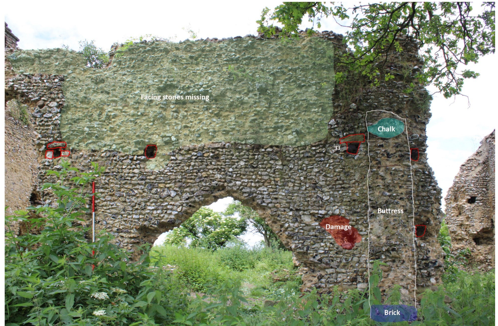
Figure 15: South wall details (exterior)
