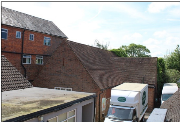
Plate 45: The Old Telephone dual pitched slated roof, facing southeast
