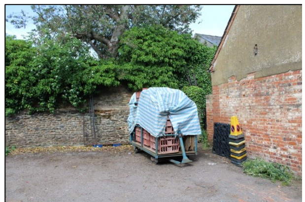
Plate 36: Western boundary wall adjacent to rear of Building 3, facing northwest
