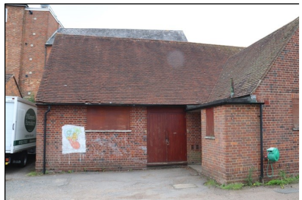
Plate 42: The Old Telephone Exchange, facing southeast
