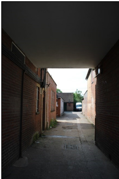
Plate 17: Carriageway arch & access road, view from the High Street, facing south. The Old Telephone Exchange is visible to the rear
