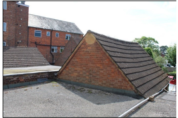
Plate 32: Former boundary wall/flat roofed section and Building 3 pitched roof, facing southeast
