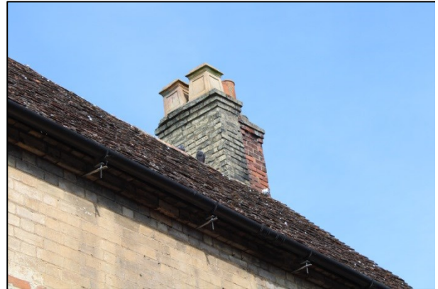
Plate 28: Building 2, detail of roof and chimney, facing northwest
