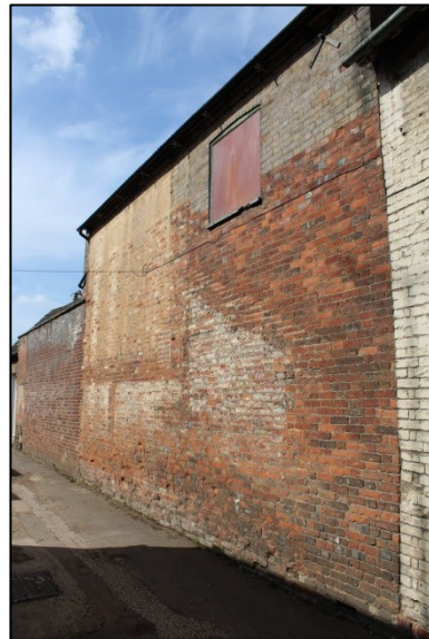
Plate 26: Building 2, facing southwest
