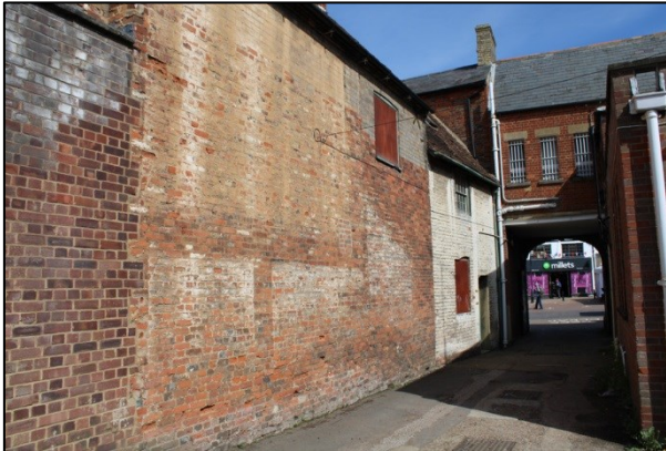
Plate 27: Building 2, facing northwest
