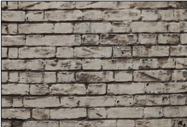
Plate 25: Building 1 (white section) detail of brickwork, facing east
