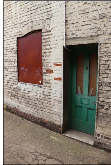
Plate 22: Building 1 (white section) detail of door & ground floor window, facing southwest
