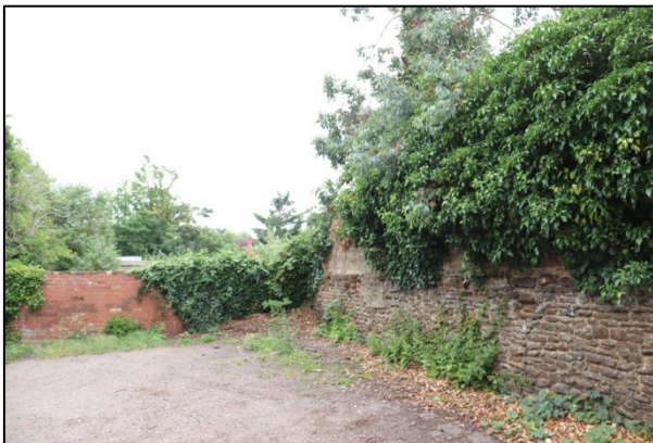
Plate 39: Western and southern boundary walls, facing southwest
