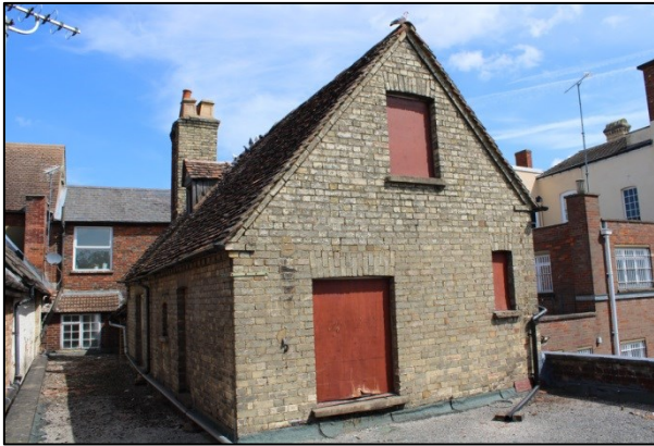
Plate 31: Building 2 and former boundary wall: pitched and flat roofs, facing northeast
