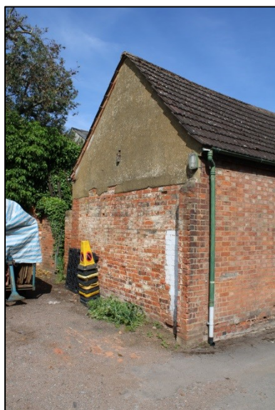
Plate 35: Building 3, gable end, facing northwest
