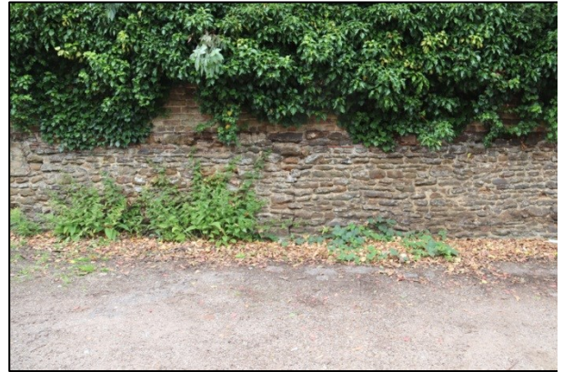
Plate 38: Western boundary wall, facing west
