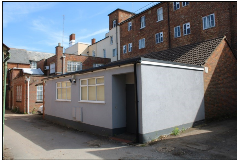
Plate 12: The Jehovah's Witnesses Kingdom Hall, facing northeast
