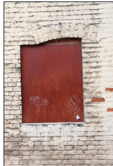
Plate 24: Building 1 (white section) detail of ground floor window, facing east
