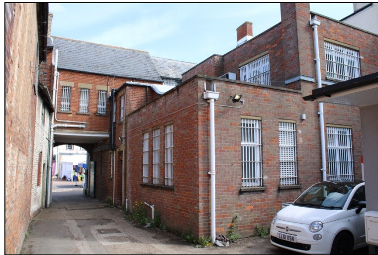
Plate 10: The west side/rear of No.48 High Street (HSBC Bank) and carriageway arch, facing northeast
