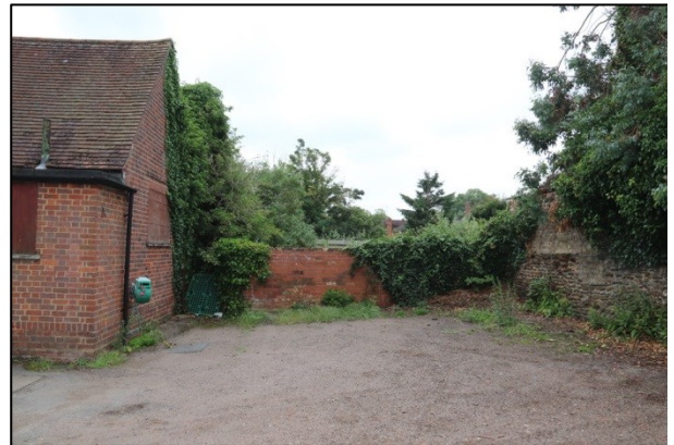
Plate 40: Boundary walls to rear of the proposed development site and western end of the Old Telephone Exchange, facing south
