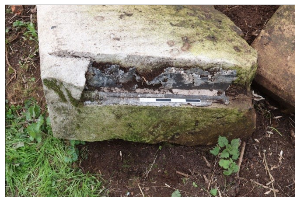
Plate 24: Stone 4 lead flashing, facing east
