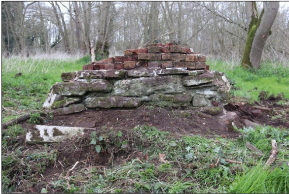
Plate 7: Stone and brick plinth, facing west
