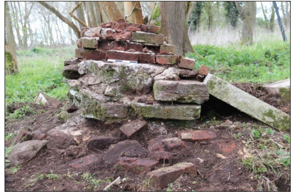
Plate 8: Stone and brick plinth, facing south
