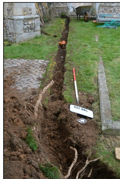
Plate 5: Service trench, looking north northeast
