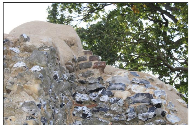
Plate 36: Northwest corner of the nave from the south
