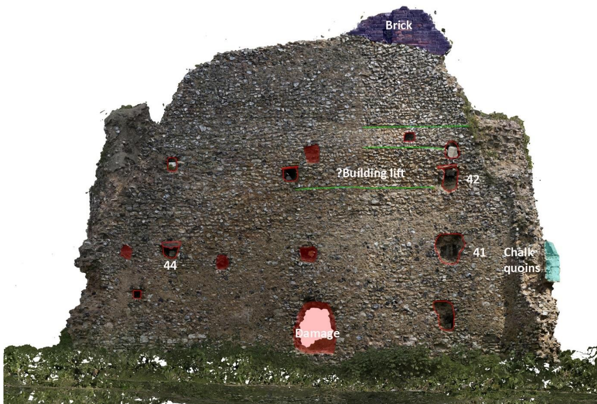
Figure 22: West wall exterior(before)
