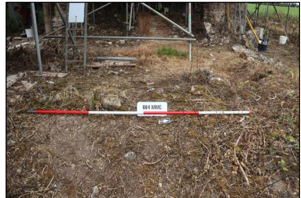
Plate 4: East wall from the east
