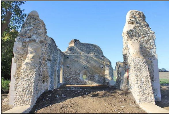
Plate 15: Internal view of the nave from the east
