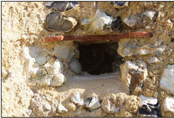
Plate 25: Detail of putlog hole in the west wall from the west
