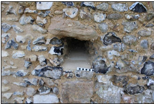
Plate 27: Detail of putlog hole in the west wall from the west
