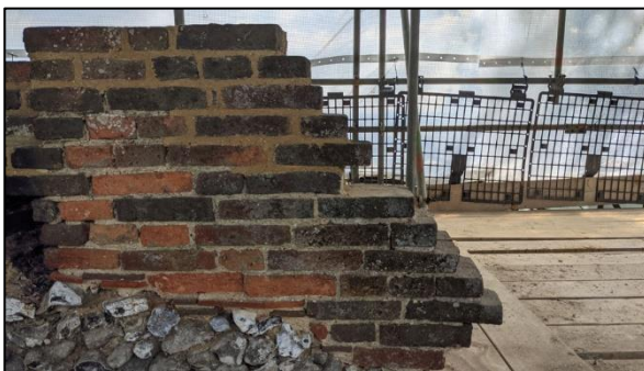
Plate 3: Detail of southern side of west wall of the bellcote
