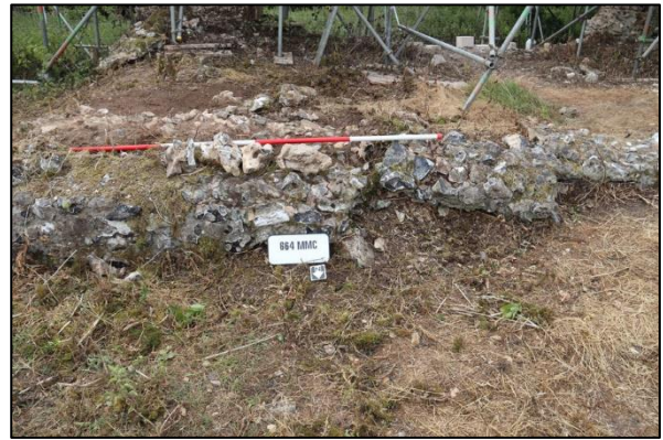
Plate 12: East end of north chancel wall from the north
