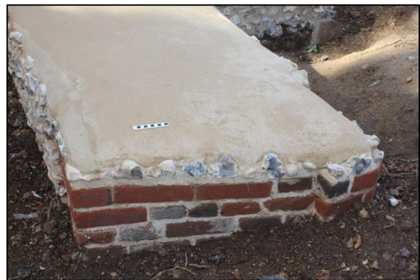
Plate 21: Door opening repaired
