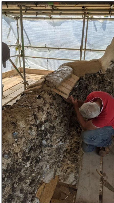
Plate 10: South nave wall under repair
