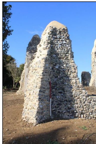
Plate 8: Southeast chancel buttress from the east
