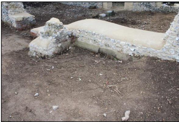
Plate 39: North nave wall from the northwest
