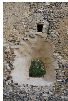
Plate 42: Detail of repaired opening in the west wall
