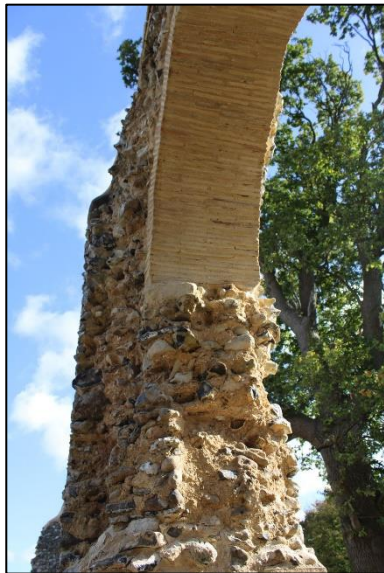
Plate 33: Detail of brick arch repair from the east
