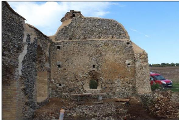
Plate 17: West wall from the east
