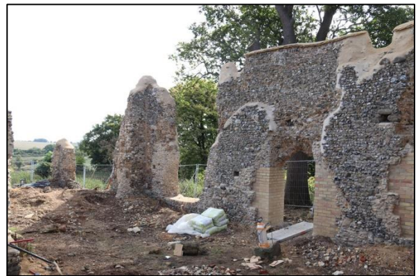
Plate 14: South nave wall from the northwest
