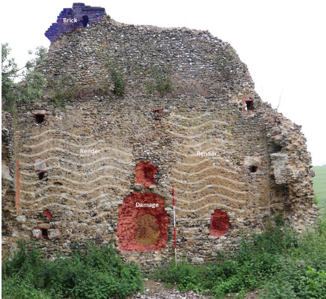
Figure 24: West wall interior(before)
