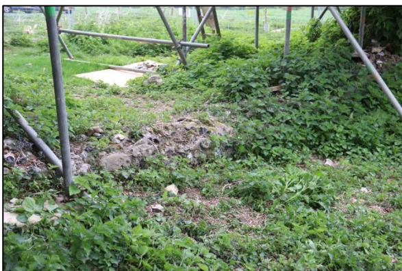
Plate 13: South chancel wall from the southwest
