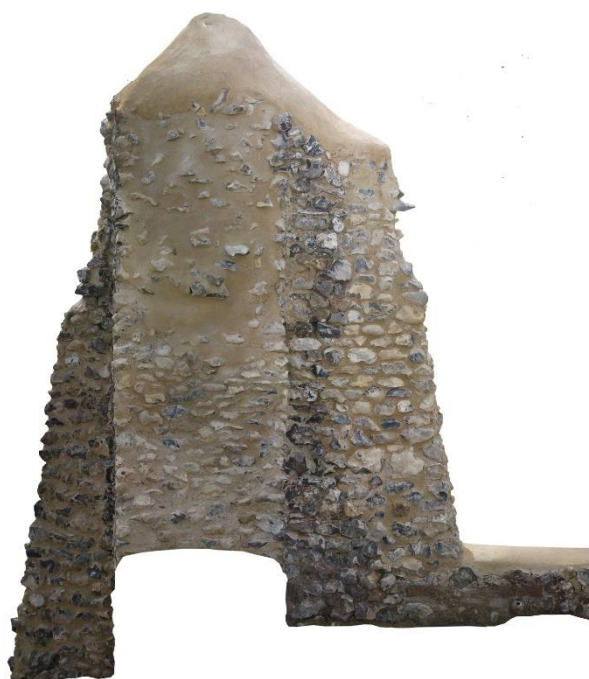
Figure 33: South chancel wall interior (after)
