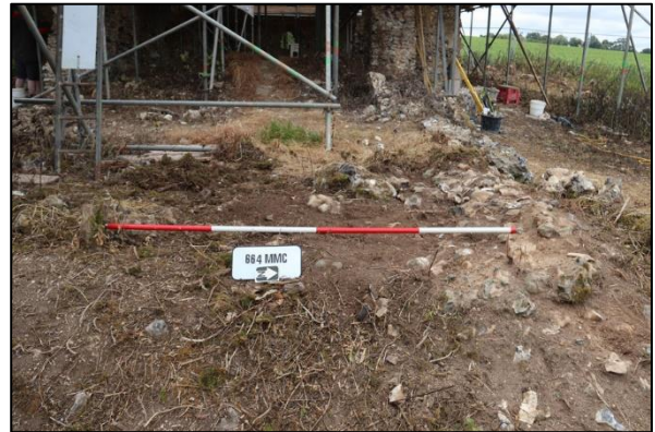
Plate 14: East end of north chancel wall from the east
