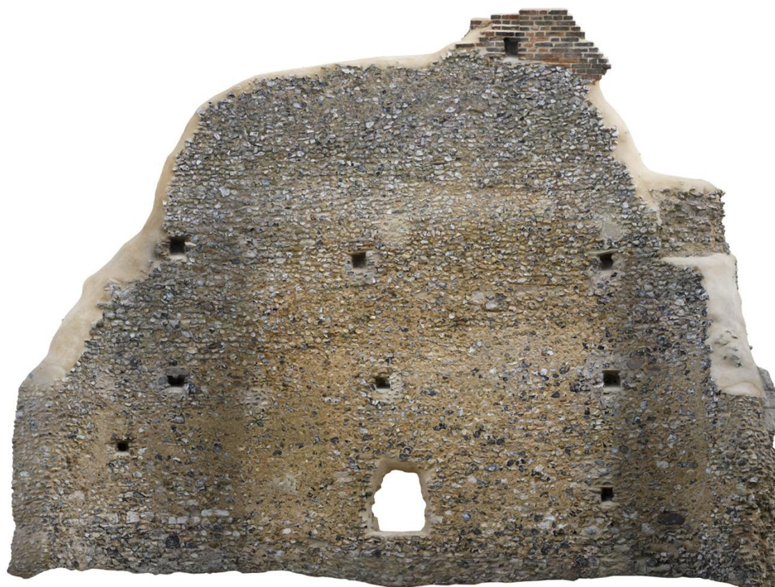
Figure 23: West wall exterior (after)
