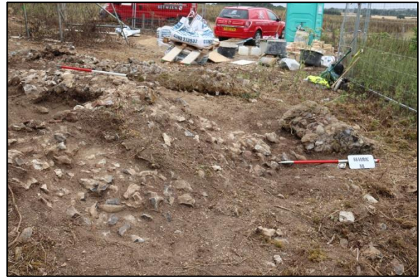
Plate 12: East chancel wall and northeast buttress from the south
