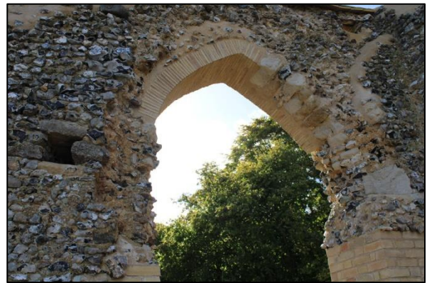
Plate 34: Detail of brick arch repair from the north
