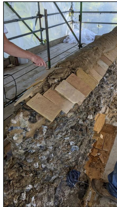
Plate 11: South nave wall under repair
