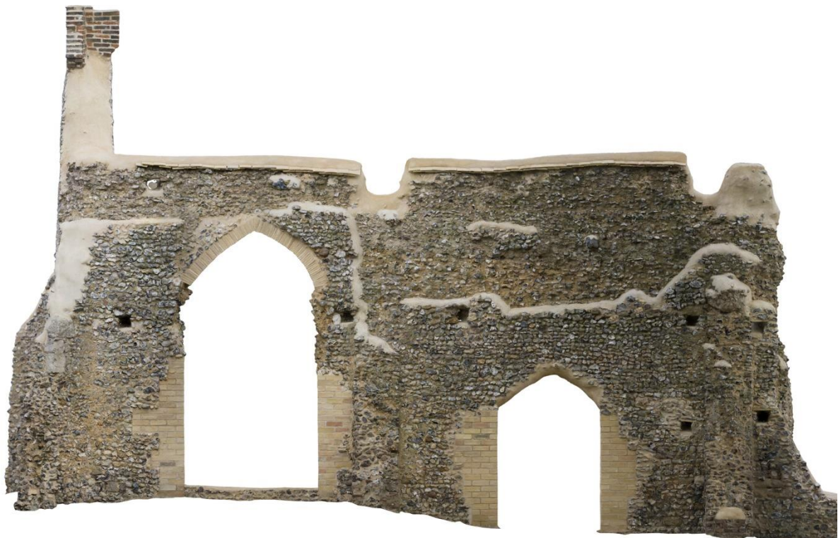
Figure 29: South nave wall exterior(before)
