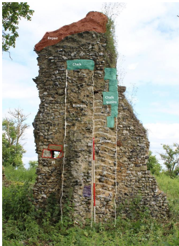
Figure 30: South chancel wall exterior (before)
