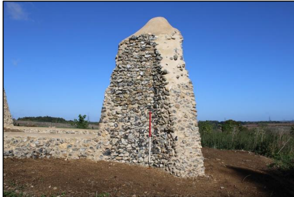
Plate 9: Southeast chancel buttress and south chancel wall from the south
