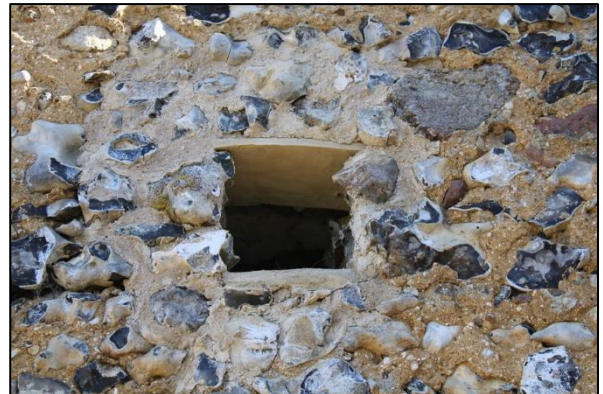
Plate 22: Detail of putlog hole in the west wall from the west
