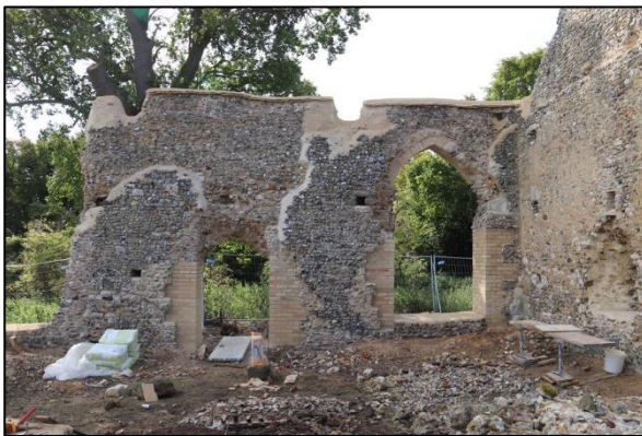
Plate 13: South nave wall from the north
