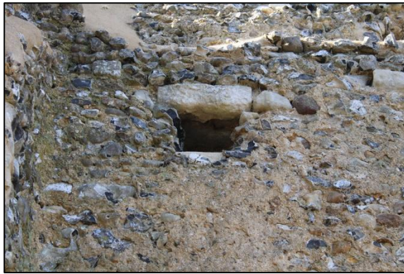
Plate 31: Detail of putlog hole in the west wall from the east
