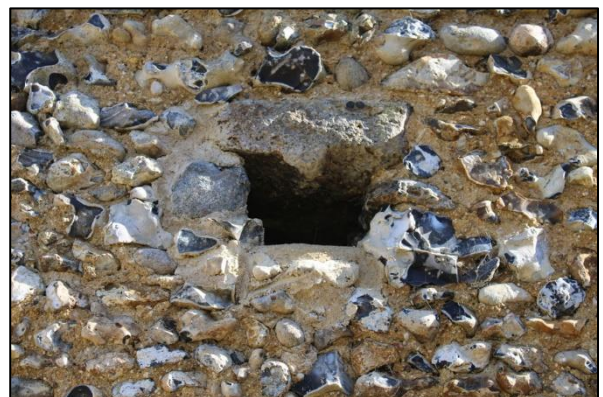
Plate 24: Detail of putlog hole in the west wall from the west
