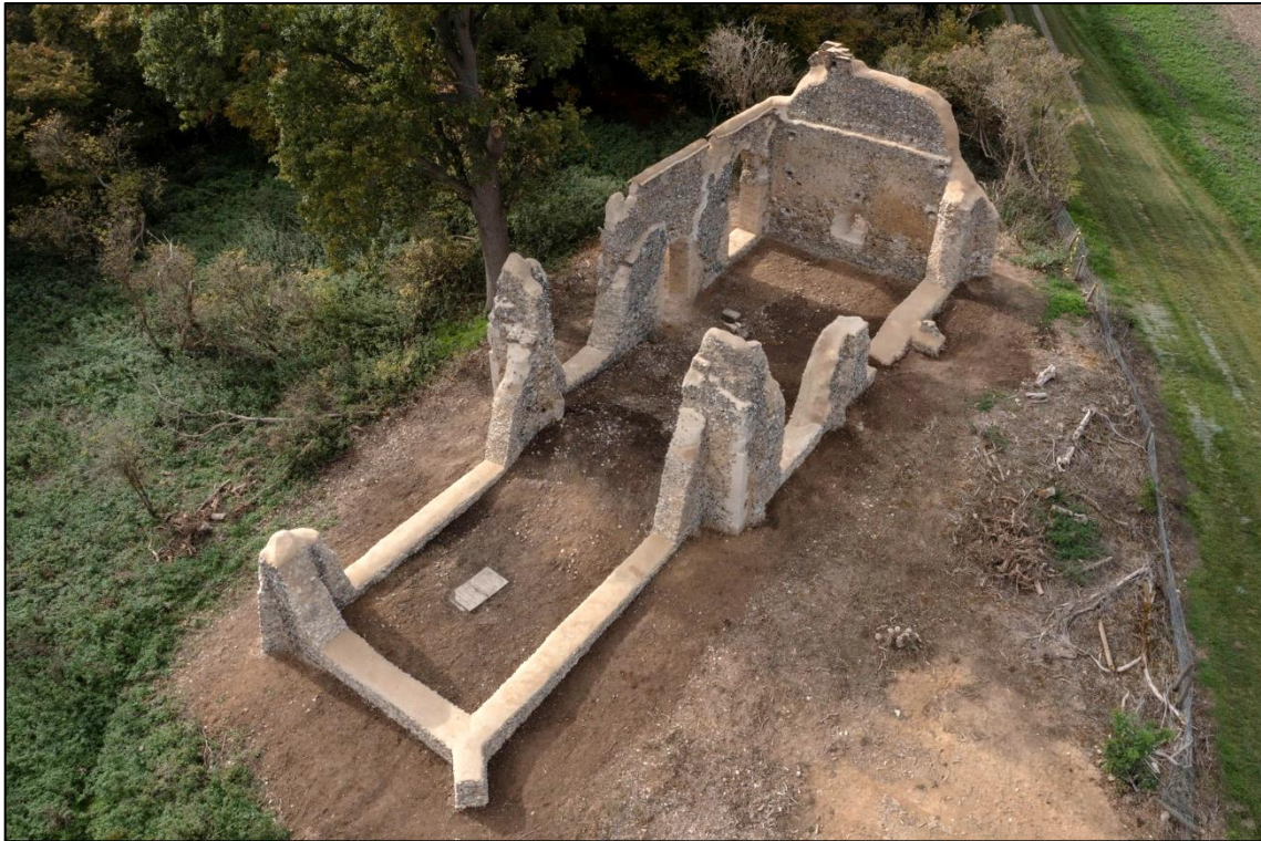
Figure 41: Minsden Chapel, the completed works (Courtesy of AerialCam)
