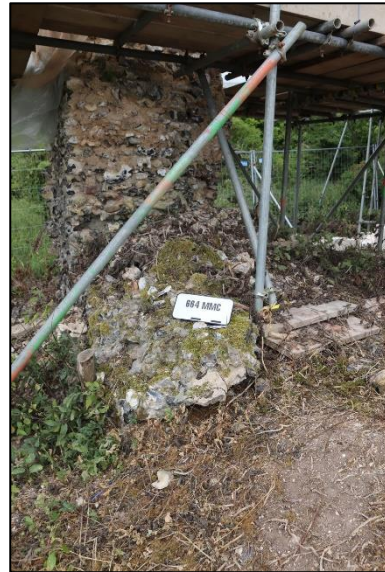
Plate 6: Southeast chancel buttress from the northwest
