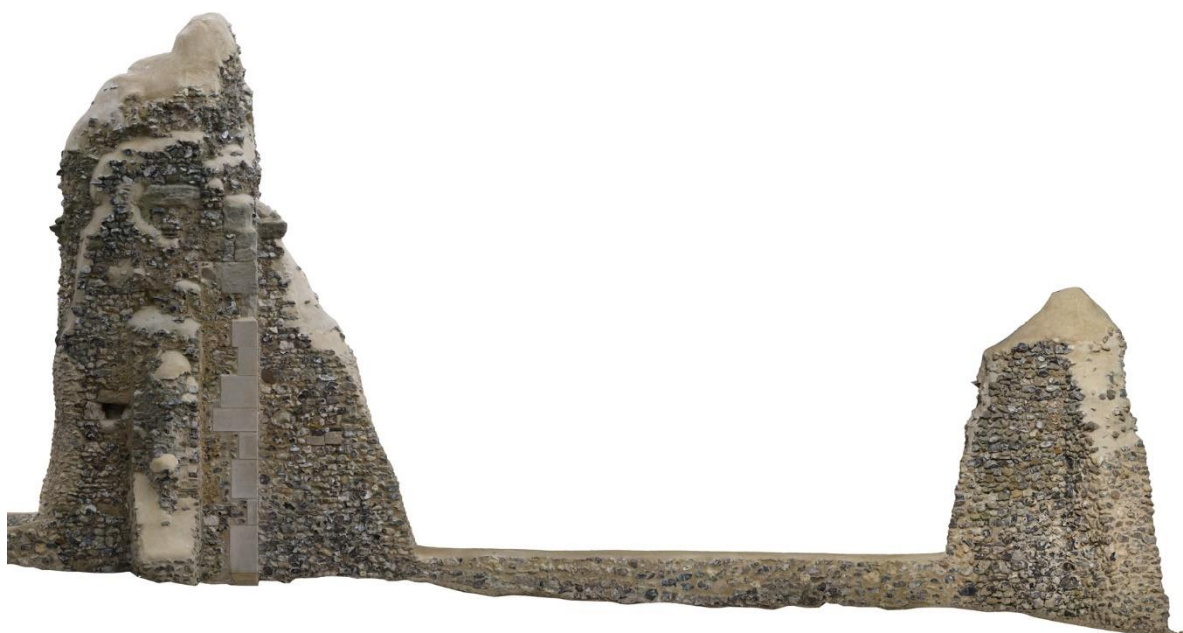
Figure 31: South chancel wall exterior(after)
