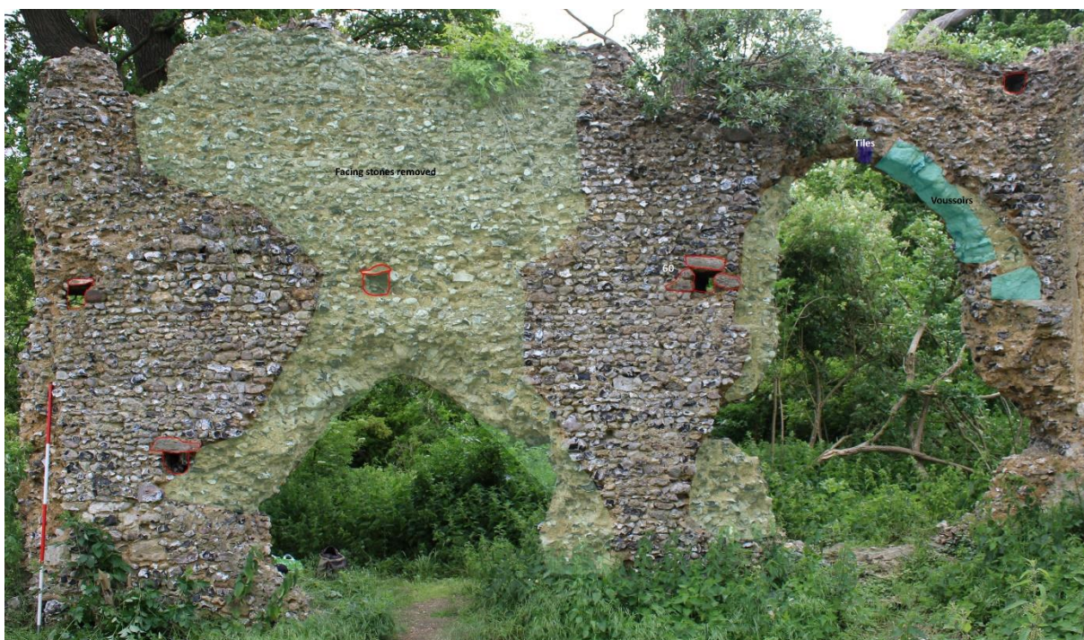
Figure 26: South nave wall interior (before)
