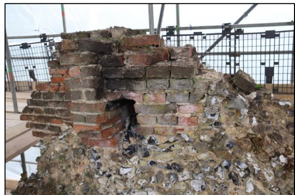
Plate 2: Bellcote from the northeast
