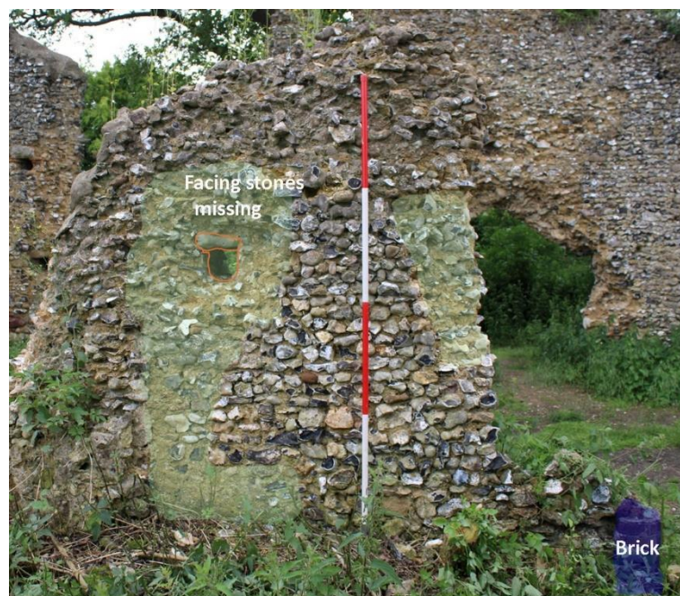
Figure 35: North nave wall exterior, centre (before)
