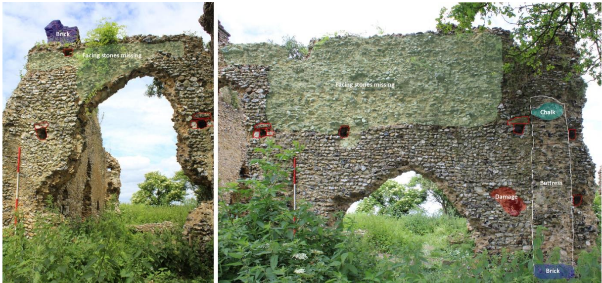
Figure 28: South nave wall exterior (before)
