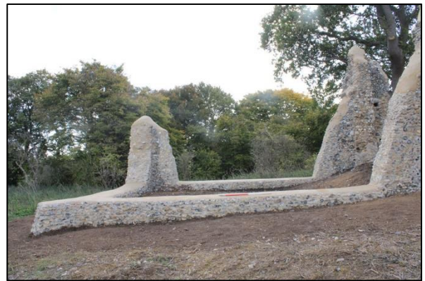
Plate 40: Chancel from the north
