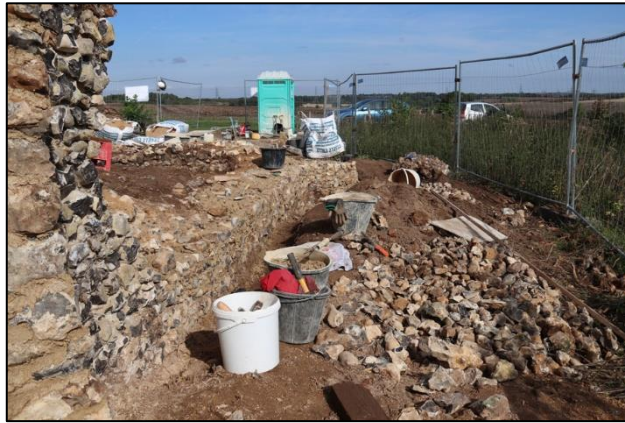
Plate 19: East chancel wall being rebuilt
