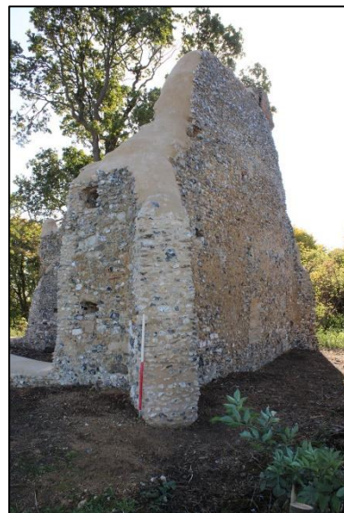
Plate 4: Northwest corner of the nave
