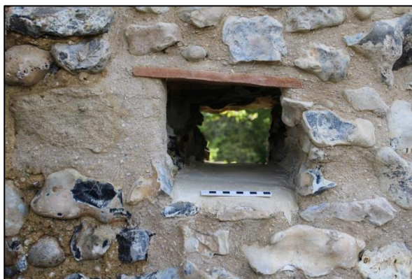
Plate 35: Detail of putlog hole in the west wall from the east
