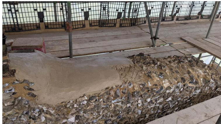
Plate 13: Example of hard capping in progress
