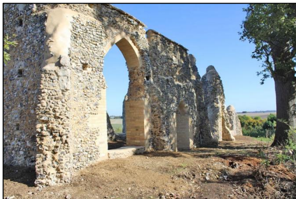
Plate 13: South wall from the southwest
