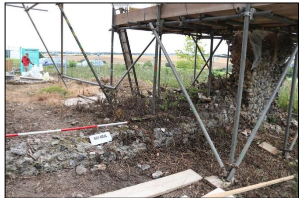
Plate 8: South chancel wall from the southwest
