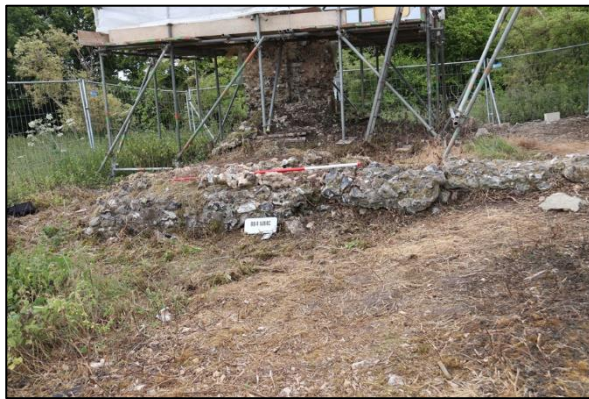
Plate 13: East end of north chancel wall from the north
