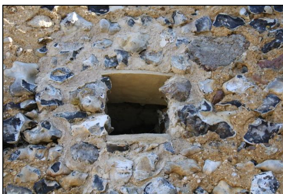
Plate 17: Example of a repaired putlog hole
