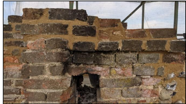
Plate 2: Detail of upper courses, looking west
