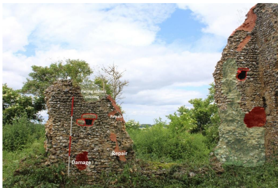
Figure 38: North nave wall interior, east (before)
