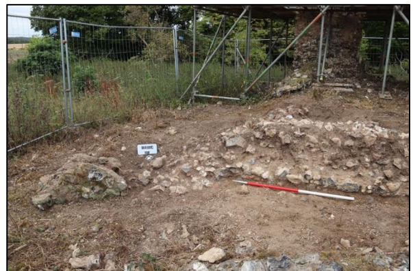
Plate 4: North chancel wall and buttress from the northeast
