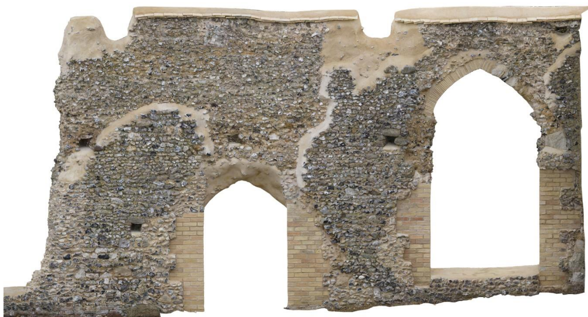
Figure 27: South nave wall interior (after)
