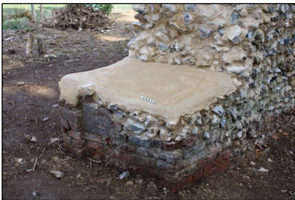
Plate 20: Door opening repaired
