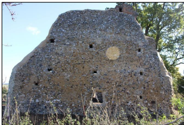
Plate 3: External face of the west wall
