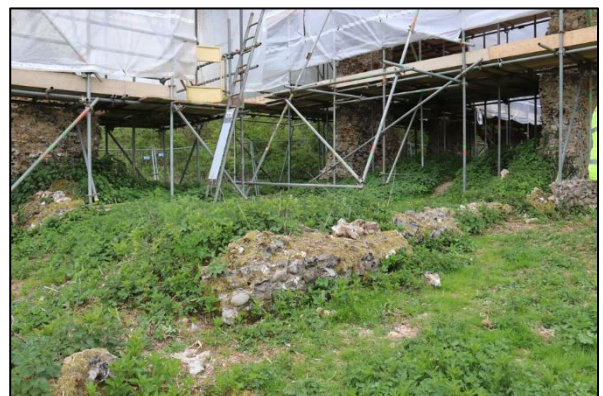
Plate 14: North chancel wall from the northeast
