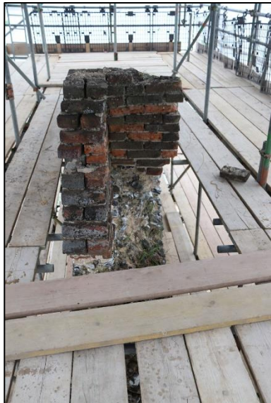
Plate 5: Bellcote from the south
