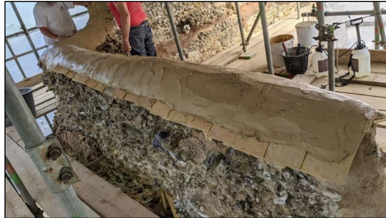
Plate 12: Completed repairs to south nave wall
