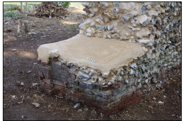
Plate 28: Detail of east side of the north nave wall opening from the southwest
