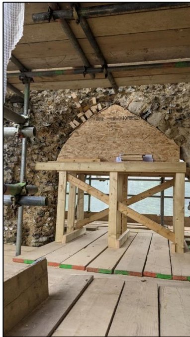
Plate 14: Arched opening under repair
