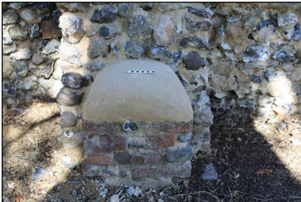
Plate 21: Detail of south chancel/nave buttress repair
