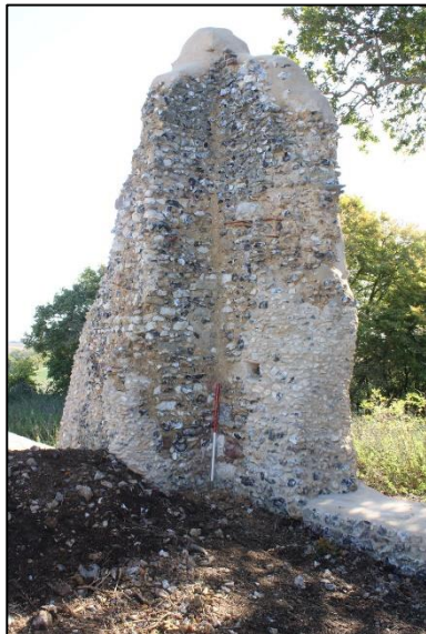
Plate 17: South wall at the nave/chancel interface from the northwest
