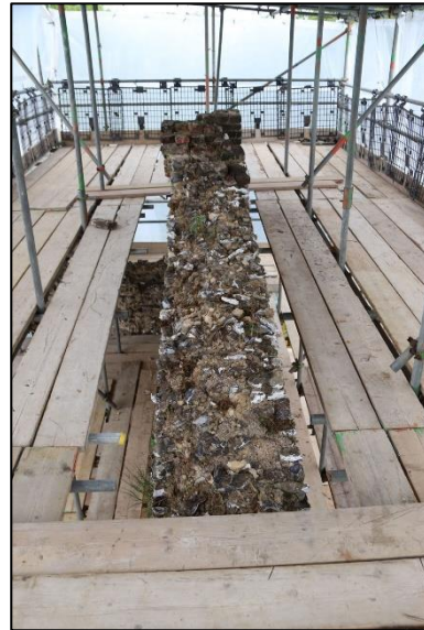
Plate 4: Wall and bellcote from the north
