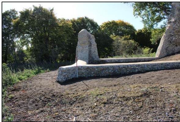
Plate 7: Chancel from the north
