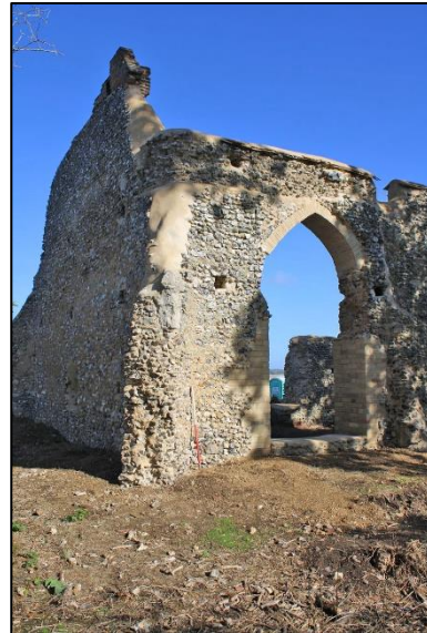
Plate 2: Southwest corner of the nave
