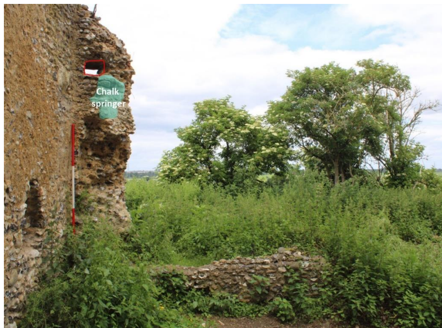
Figure 37: North nave wall interior, west (before)
