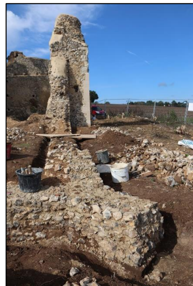
Plate 10: North east buttress from the east
