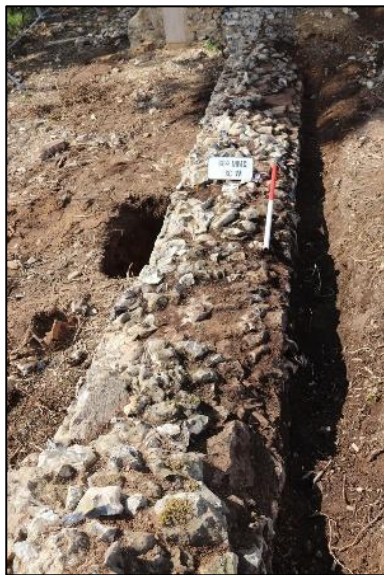
Plate 23: South chancel wall from the east
