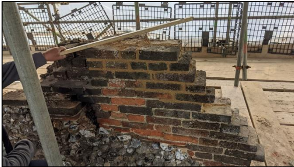
Plate 1: Bellcote under repair, looking east
