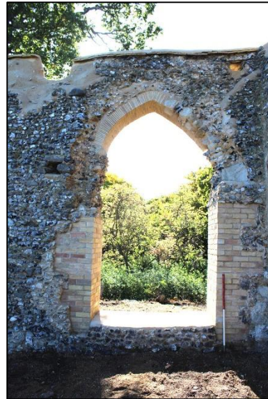
Plate 20: Opening in south nave wall from the north
