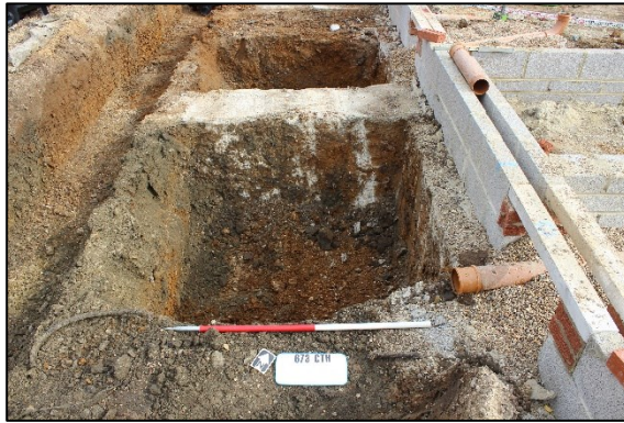
Plate 7: Porch footing, looking northwest
