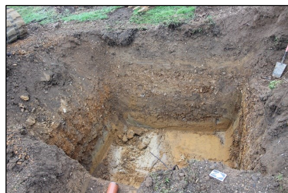
Plate 6: Soakaway, looking southwest
