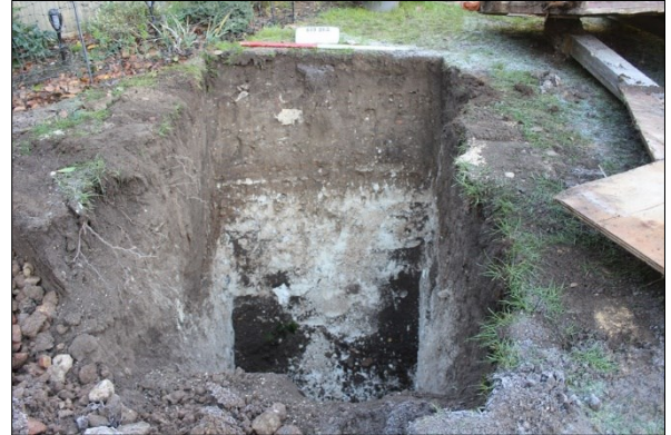
Plate 8: Soakaway, view NNE
