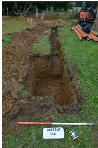
Plate 19: Soakaway 5, looking northeast
