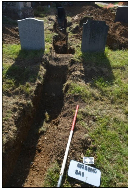
Plate 23: Soakaway 6 service, looking east
