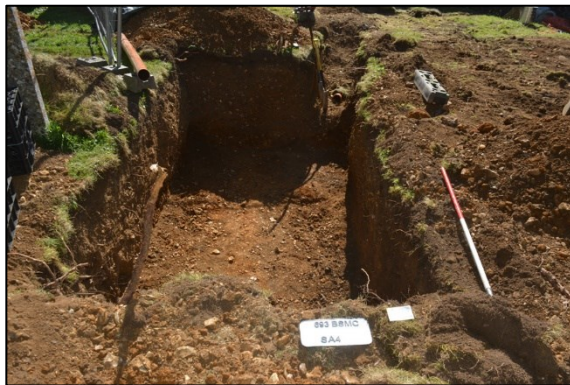
Plate 8: Soakaway 4 fully excavated, looking east
