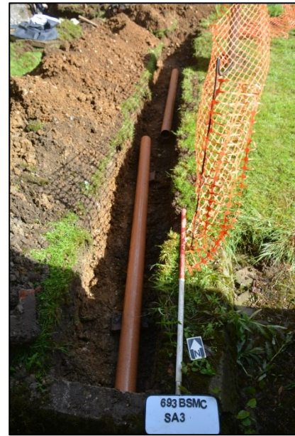
Plate 7: Soakaway 3 service run, looking north northeast
