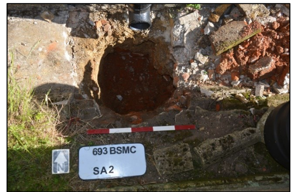
Plate 54: Soakaway 2 Catch Basin, looking north
