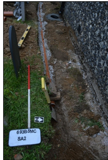
Plate 2: Soakaway 2 service run, looking west
