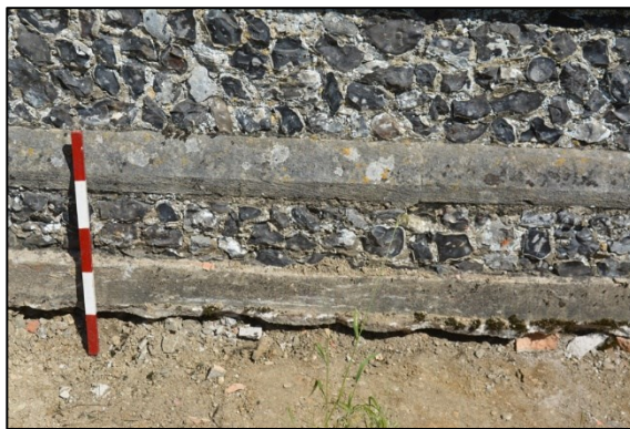
Plate 53: Partially exposed church foundation
