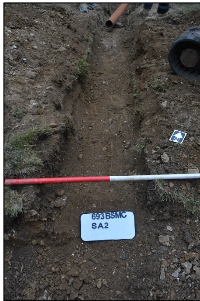
Plate 1: Soakaway 2 service run, looking north northwest
