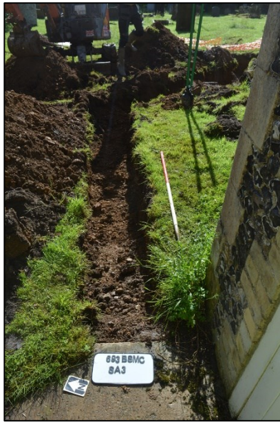
Plate 6: Soakaway 3 service run, looking east northeast
