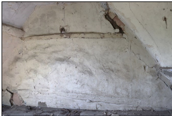
Plate 49: F1: west wall
