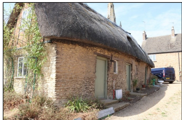
Plate 2: North elevation from the northeast
