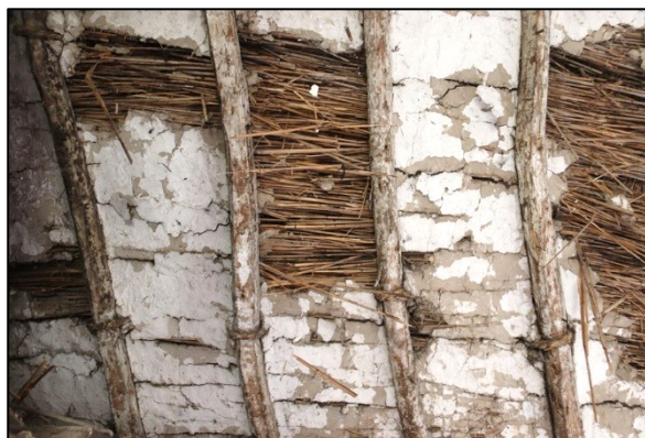
Plate 25: G1: thatching detail in north wall
