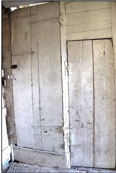
Plate 35: G2: doors to staircase and understairs cupboard
