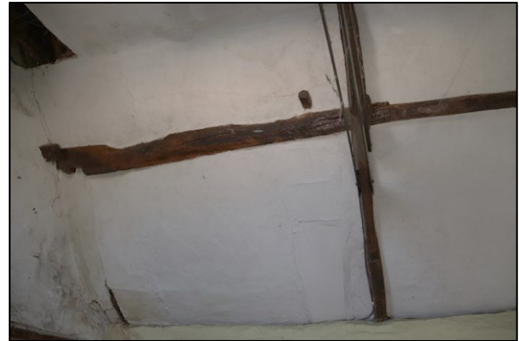
Plate 20: G1: ceiling timbers
