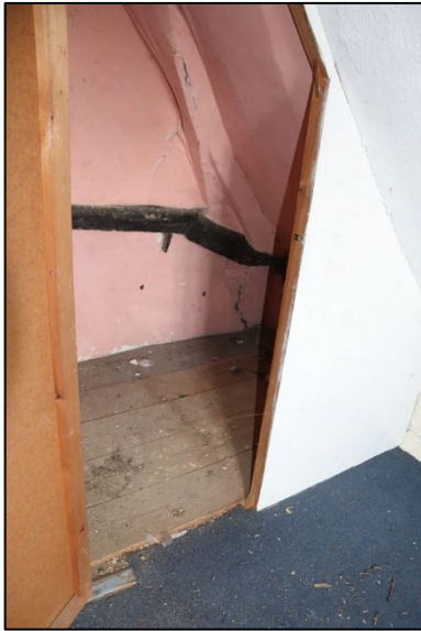
Plate 56: F2: cupboard in northwest corner
