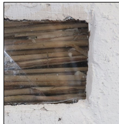
Plate 43: G4: Building fabric of stairs
