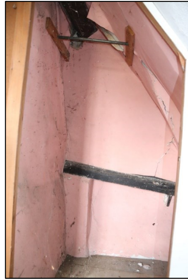
Plate 57: F2: cupboard in northwest corner
