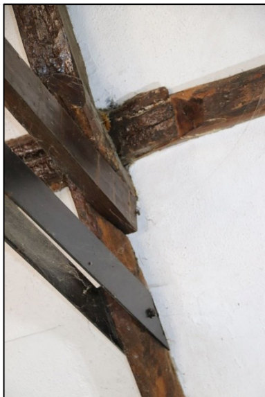
Plate 21: G1: truss and purlin detail
