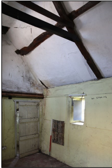
Plate 19: G1: southeast corner
