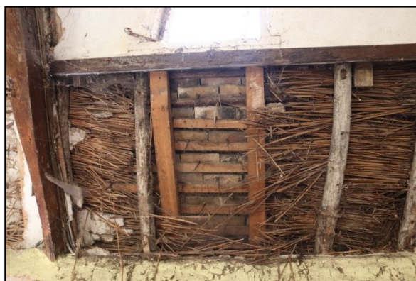
Plate 27: G1: roof detail beneath dormer window
