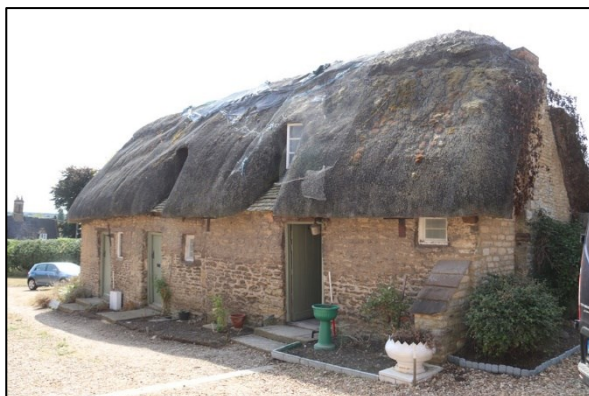
Plate 1: North elevation from the northwest
