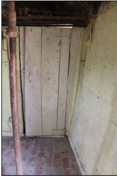
Plate 29: G1: plank and batten door to cupboard (external face)
