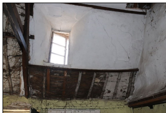
Plate 16: G1: north wall ceiling, east of door
