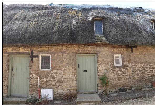
Plate 4: North elevation: central unit
