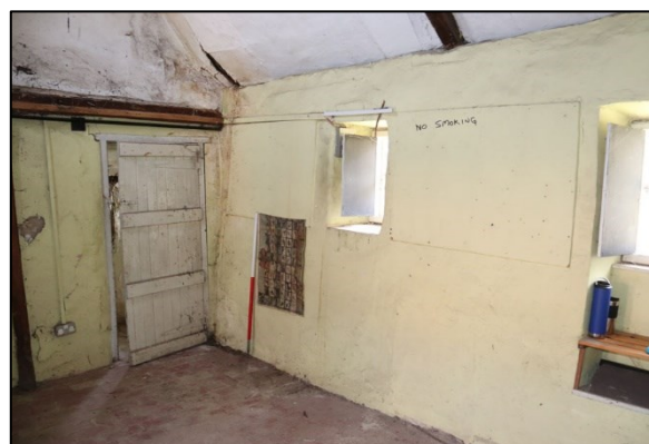
Plate 18: G1: southeast corner
