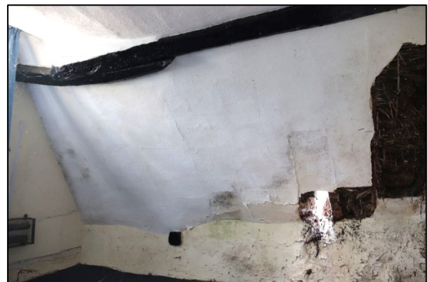
Plate 55: F2: south wall
