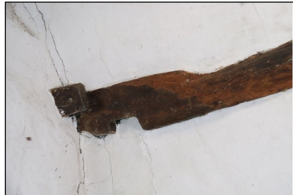
Plate 22: G1: purlin detail (SE corner of room)
