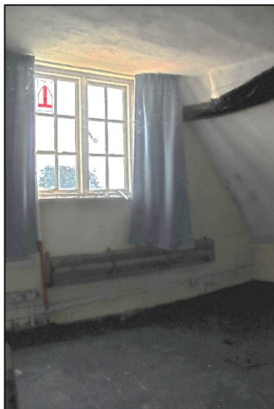
Plate 54: F2: east wall
