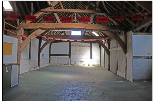
Plate 8: Barn 1, Unit 1, looking east
