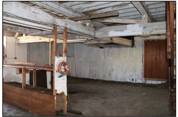
Plate 14: Barn 1, Unit 2, looking southwest
