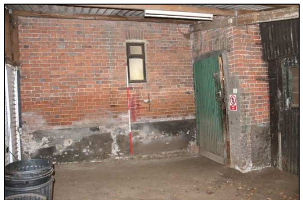
Plate 22: Barn 1, Unit 4, looking east
