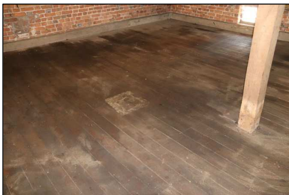
Plate 21: Barn 1, Unit 2, first floor, floor detail
