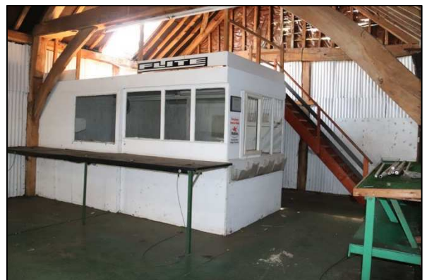
Plate 12: Barn 1, Unit 1, looking southwest
