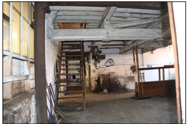
Plate 16: Barn 1, Unit 2, looking north
