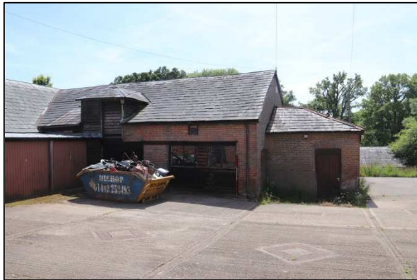
Plate 7: Barn 1, east elevation, looking southwest
