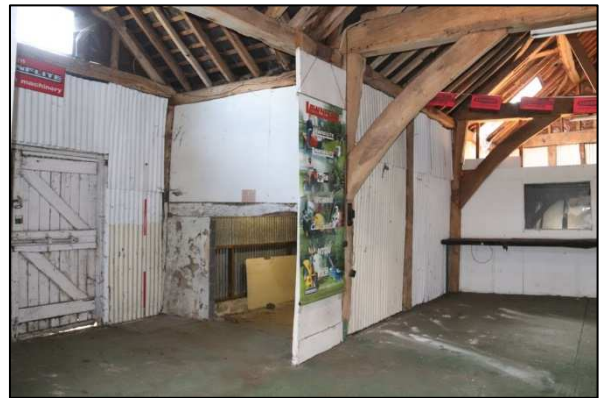
Plate 10: Barn 1, Unit 1, looking southwest
