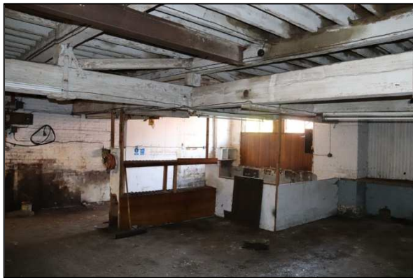
Plate 15: Barn 1, Unit 2, looking northeast
