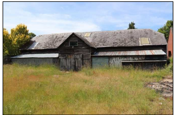
Plate 4: Barn 1, south elevation, looking north
