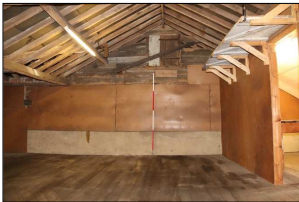
Plate 19: Barn 1, Unit 2, first floor, looking south
