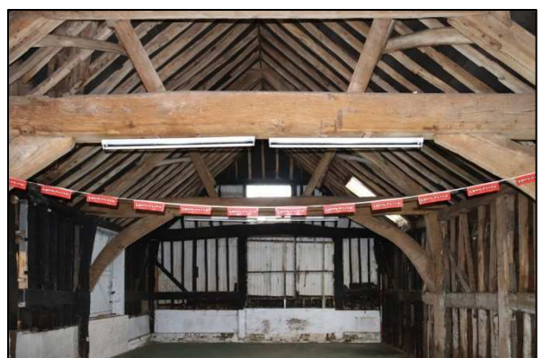
Plate 24: Barn 1, Unit 1, looking east
