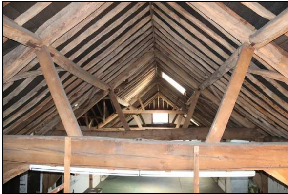
Plate 13: Barn 1, Unit 1, detail of roof structure, looking east
