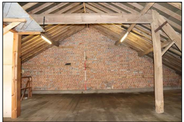
Plate 20: Barn 1, Unit 2, first floor, looking north
