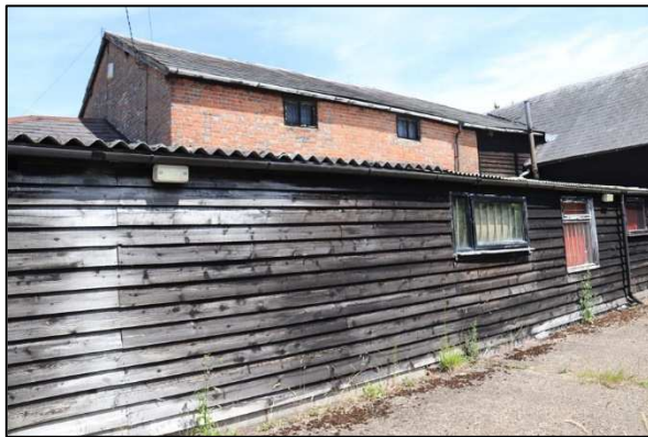
Plate 3: Barn 1, west elevation, looking southeast
