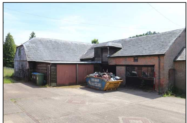
Plate 6: Barn 1, east elevation, looking southwest
