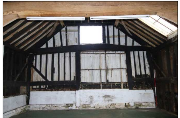
Plate 36: Barn 1, Unit 1, east wall, looking east
