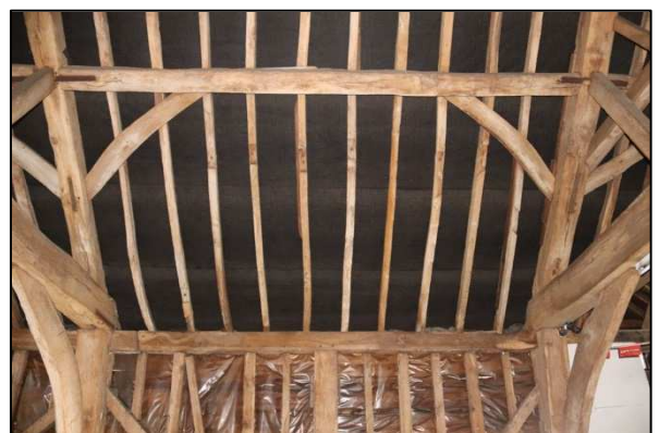
Plate 40: Barn 1, Unit 1, roofing detail, looking south
