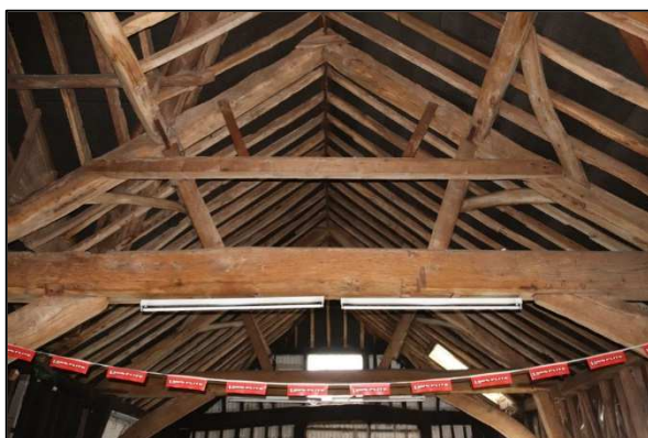
Plate 39: Barn 1, Unit 1, roofing detail, looking east
