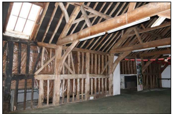
Plate 30: Barn 1, Unit 1, southern walls, looking south
