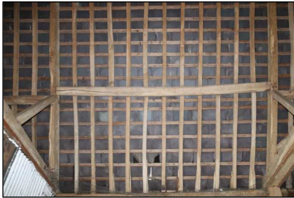
Plate 50: Barn 2, Unit 1, looking roof detail, looking north
