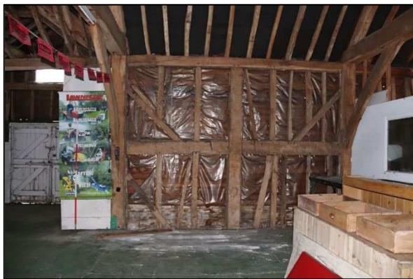
Plate 29: Barn 1, Unit 1, southern wall, looking south
