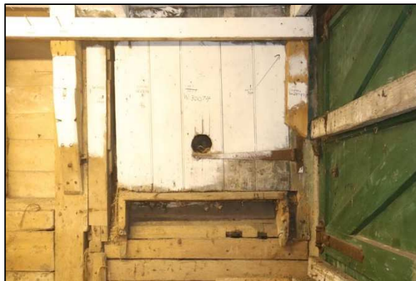
Plate 43: Barn 1, Unit2b, door to original stair to first floor, looking north
