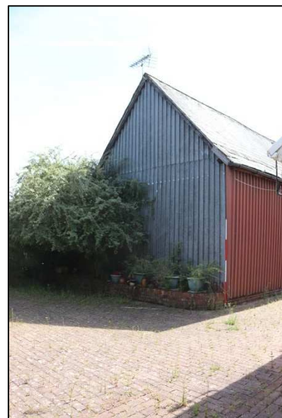
Plate 47: Barn 2, east/north elevations, looking southwest
