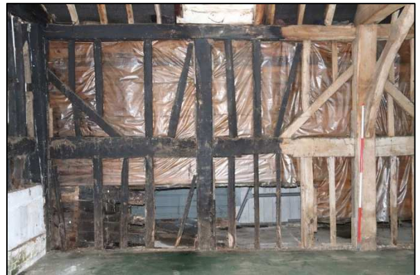
Plate 38: Barn 1, Unit 1, south wall panel detail, looking south
