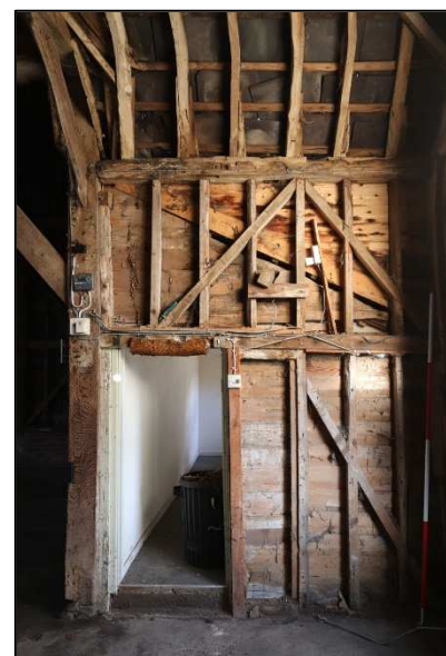
Plate 61: Barn 2, Unit 1-1b, looking east
