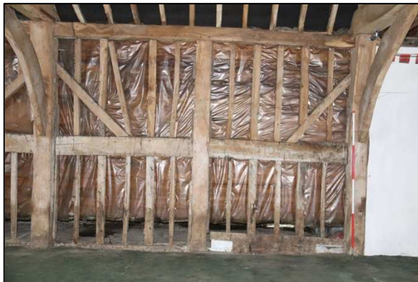
Plate 37: Barn 1, Unit 1, south wall panel detail, looking south
