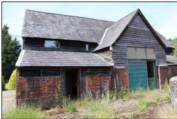
Plate 46: Barn 2, south elevation, looking northeast
