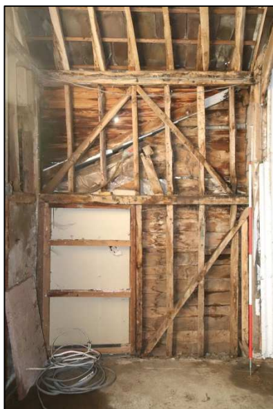
Plate 62: Barn 2, Unit 1, west wall detail, looking west
