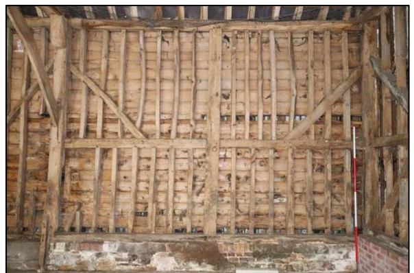
Plate 55: Barn 2, Unit 1, north wall, looking north
