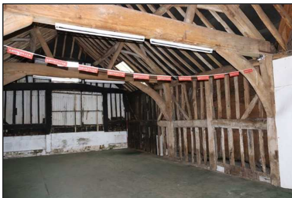
Plate 27: Barn 1, Unit 1, east & south walls, looking southeast
