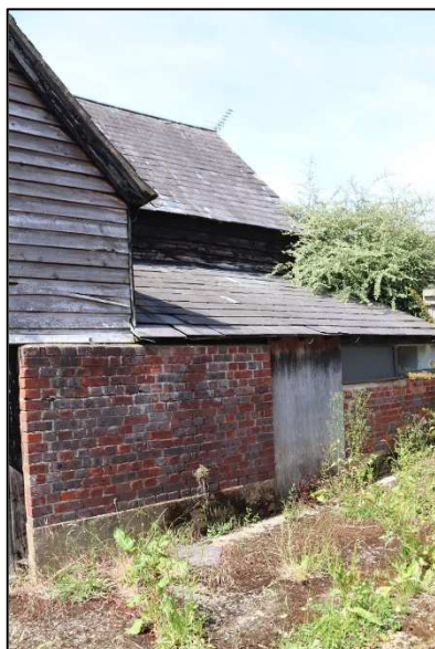
Plate 48: Barn 2, south elevation, looking northeast
