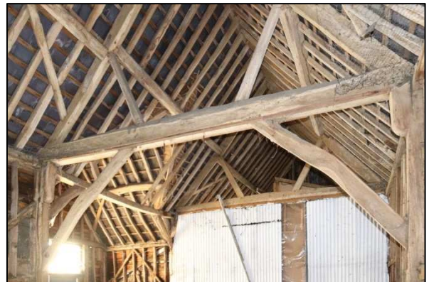
Plate 59: Barn 2, Unit 1, roof detail, looking southwest
