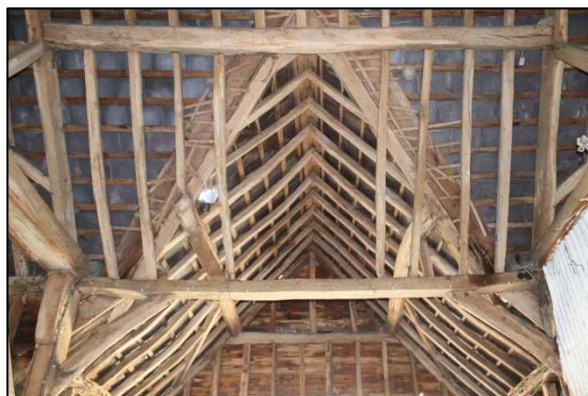
Plate 63: Barn 2, Unit 1, roof detail, looking south
