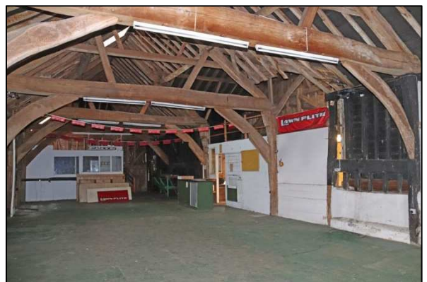
Plate 32: Barn 1, Unit 1, looking northwest
