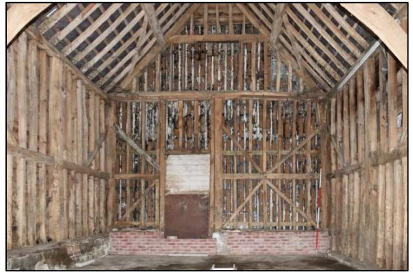
Plate 51: Barn 2, Unit 1, east wall, looking east
