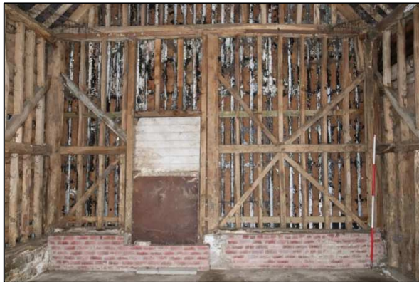
Plate 56: Barn 2, Unit 1, east wall, looking east
