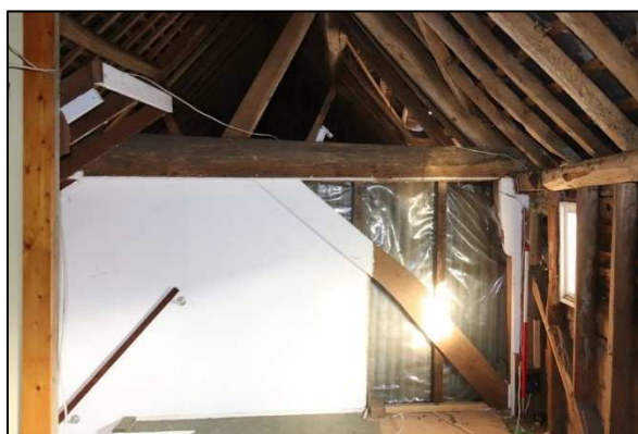
Plate 64: Barn 2, Unit 2a, looking northeast
