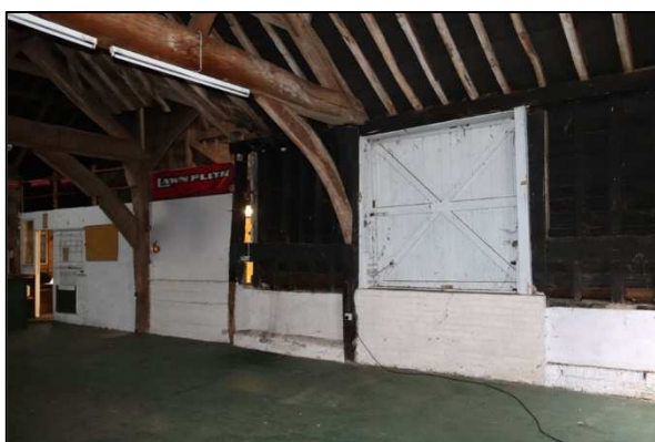
Plate 33: Barn 1, Unit 1, north wall, looking northwest
