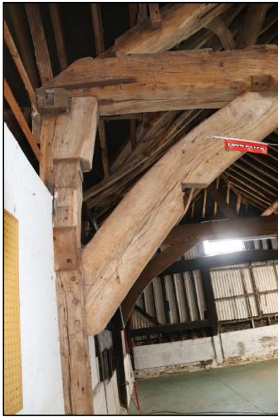
Plate 41: Barn 1, Unit1, Truss 2 detail, looking northeast
