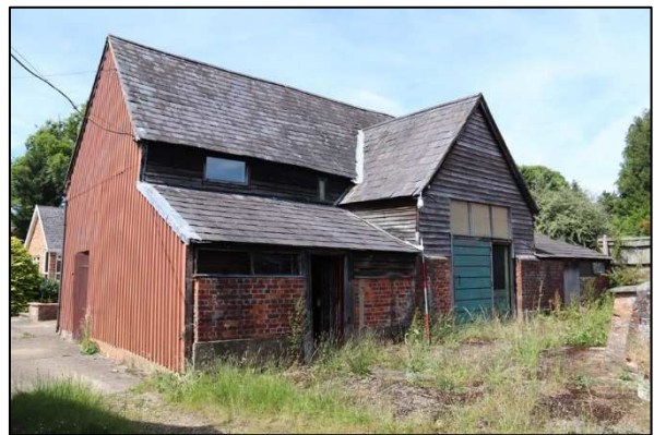
Plate 45: Barn 2, west/south elevations, looking northeast
