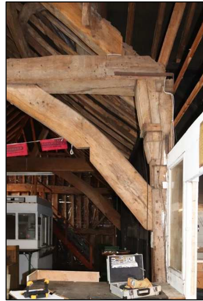
Plate 42: Barn 1, Unit1, Truss 2 detail, looking northwest
