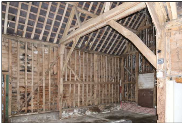
Plate 52: Barn 2, Unit 1, north wall, looking northeast
