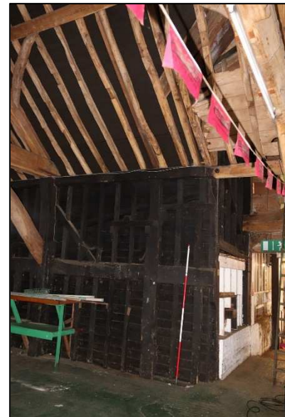
Plate 28: Barn 1, Unit 1, north wall, looking northwest
