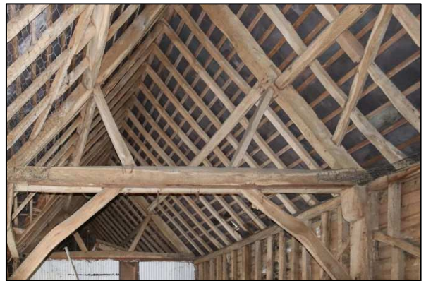
Plate 53: Barn 2, Unit 1, roof detail, looking northwest
