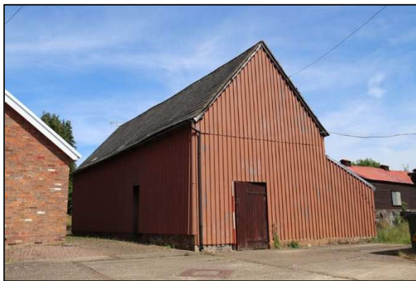
Plate 44: Barn 2, north/west elevations, looking southeast
