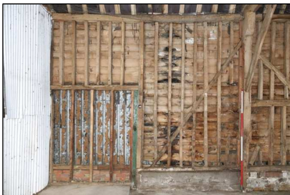
Plate 54: Barn 2, Unit 1, north wall, looking north
