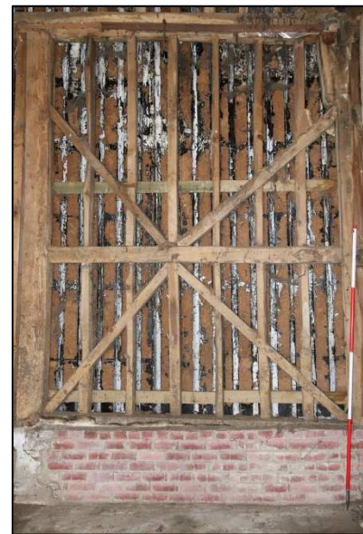
Plate 57: Barn 2, Unit 1, east wall detail, looking east
