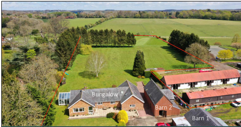
Figure 36: The site in its setting, view to the east
