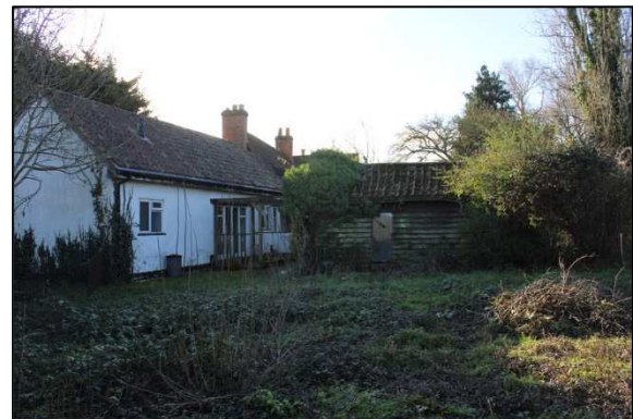
Plate 4: Shed to the west of Number 7 from the north
