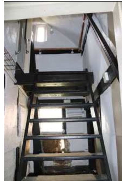
Plate 2: G5, view to first floor (25)
