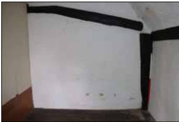
Plate 1: F2, east wall (48)
