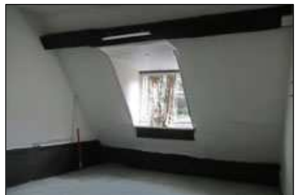
Plate 4: F4, east wall (57)
