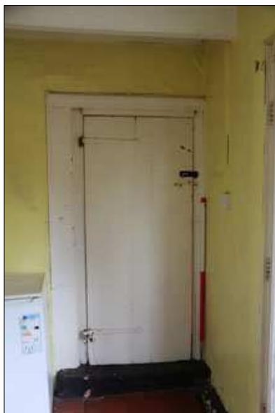
Plate 5: G9, plank and batten door (38)
