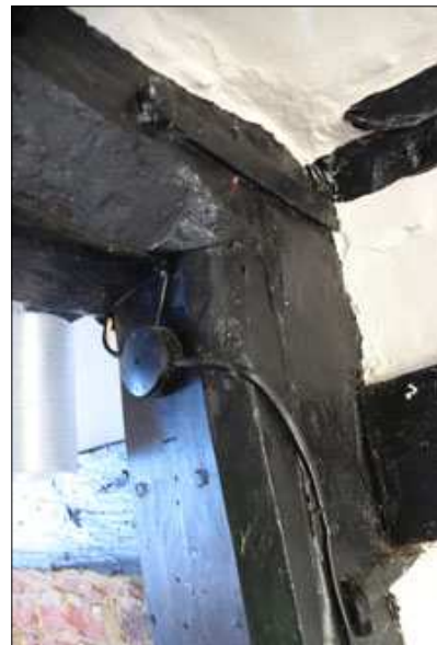
Plate 8: G4, lambs tongue chamfer stop (22)
