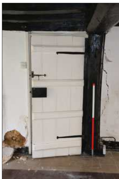
Plate 9: G4, plank and batten door in south wall (23)
