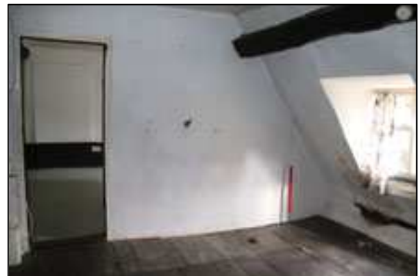
Plate 2: F4, north wall (55)
