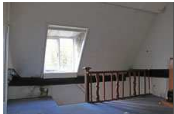
Plate 4: F6, west wall (64)
