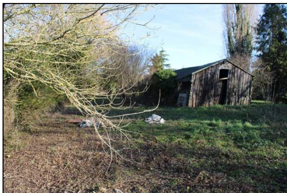
Plate 5: Large shed to west of the plot from the southwest
