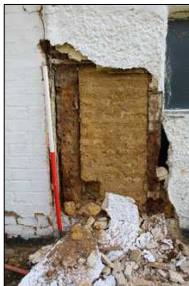
Plate 10: No 5. Exposed timber frame and wattle & daub
