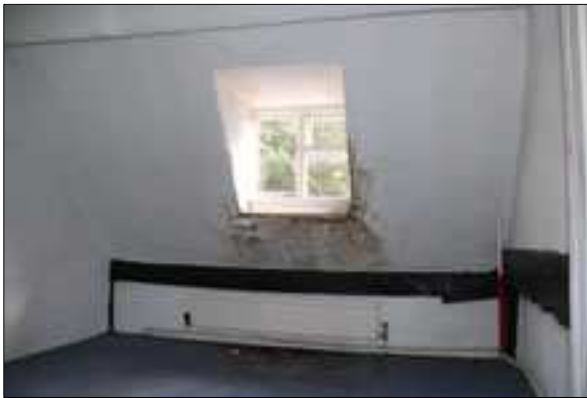
Plate 1: F6, east wall (61)
