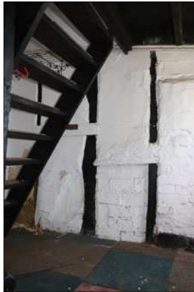
Plate 3: G5, view to south (26)
