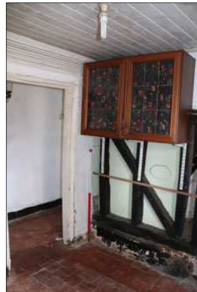
Plate 2: G6, southeast corner (28)
