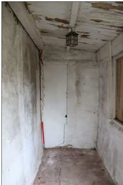
Plate 1: G10, view to south (39)
