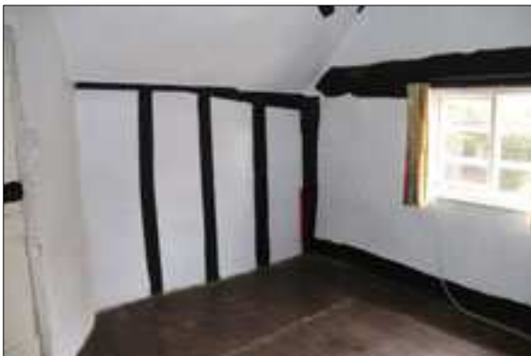
Plate 3: F3, north wall (52)
