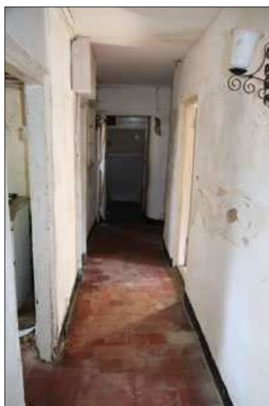
Plate 5: G1, passage looking north (5)
