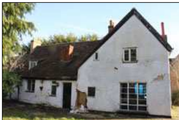
Plate 9: No. 5, west elevation
