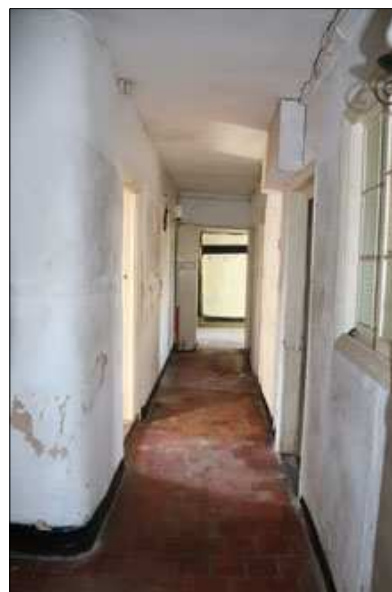
Plate 4: G1, passage looking south (4)
