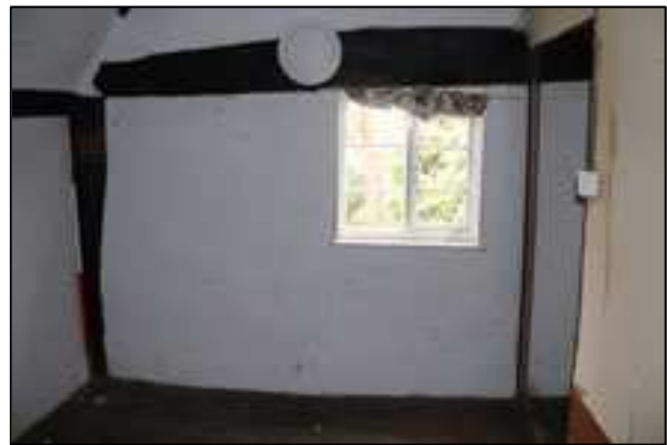
Plate 2: F2, west wall (49)
