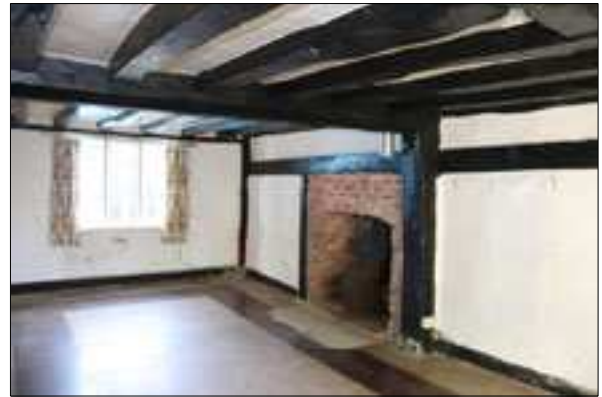
Plate 6: G4, southeast corner (20)
