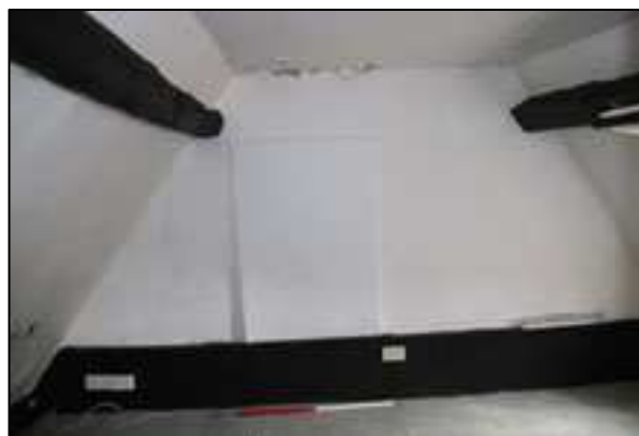
Plate 3: F5, north wall (60)
