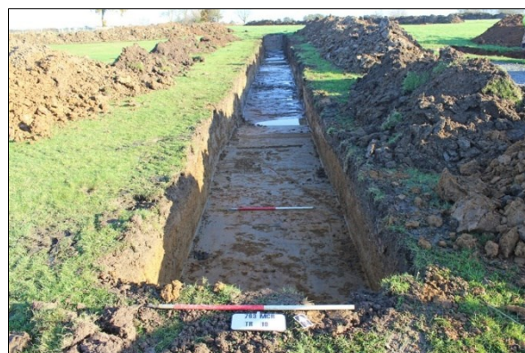
Plate 10: Trench 10 facing northeast
