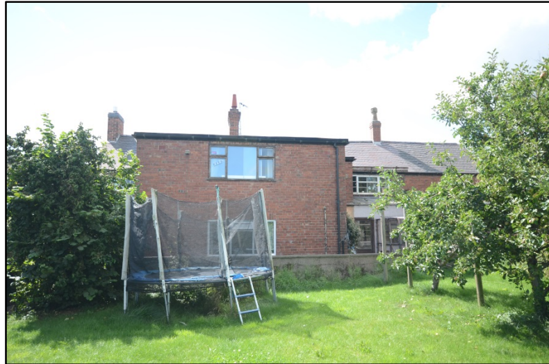
The rear extensions, looking south-west Fig 13
