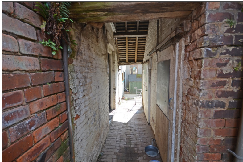
The covered passage, looking south-east Fig 21
