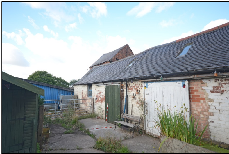
The east barn, east elevation, looking south-west Fig 20
