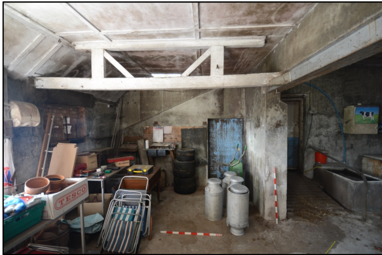
The east barn, southern room, looking south-west Fig 26
