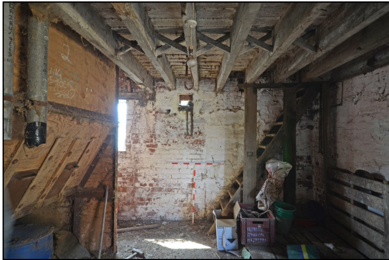
The Granary, ground floor room with access to first floor Fig 35
