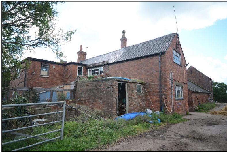
The west elevation and extensions, looking south-east Fig 11
