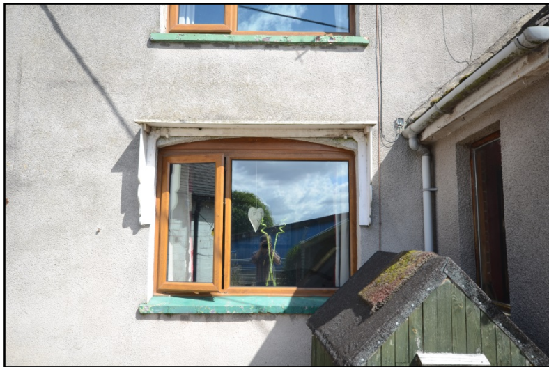
Detail of ground floor window Fig 9
