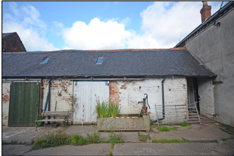
The east barn, east elevation, looking north-west Fig 19
