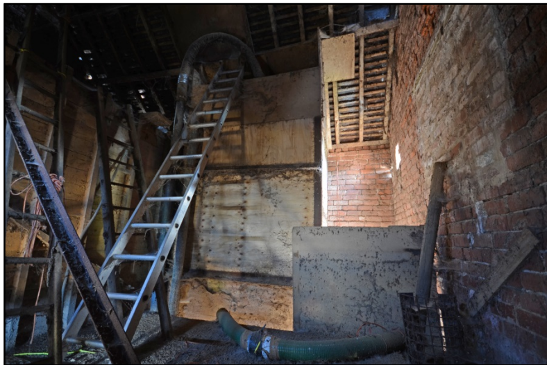
The Granary, first floor room, looking south-east Fig 37
