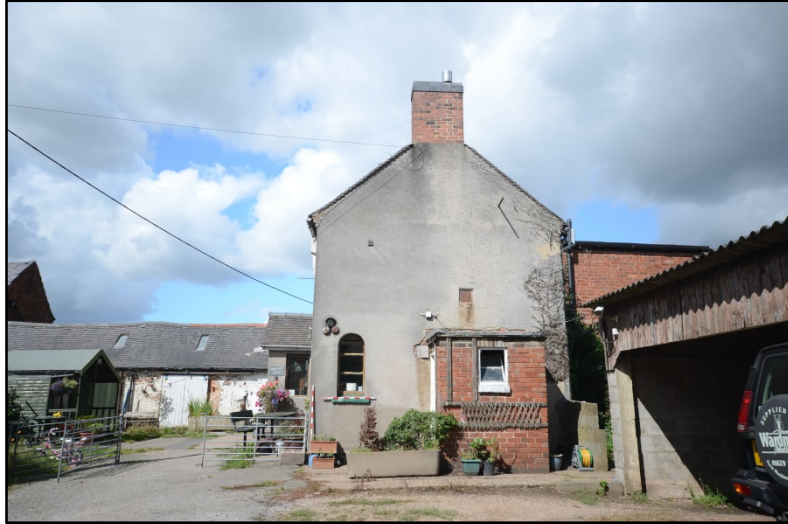
The Farmhouse, east elevation, looking north-west Fig 7
