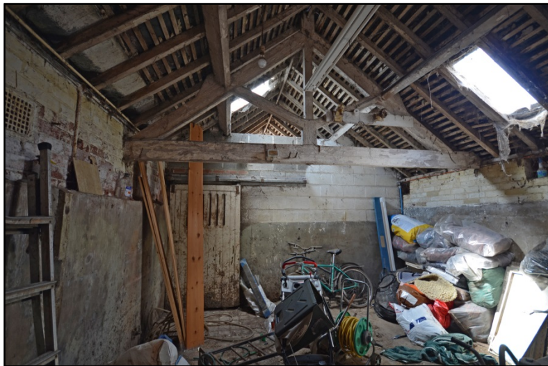
The north room of the east barn Fig 30
