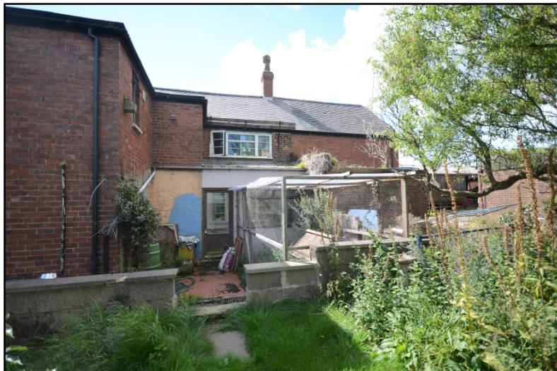
The rear extensions, looking south-west Fig 12
