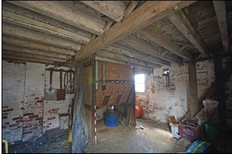
The Granary, ground floor room with feed chute Fig 34
