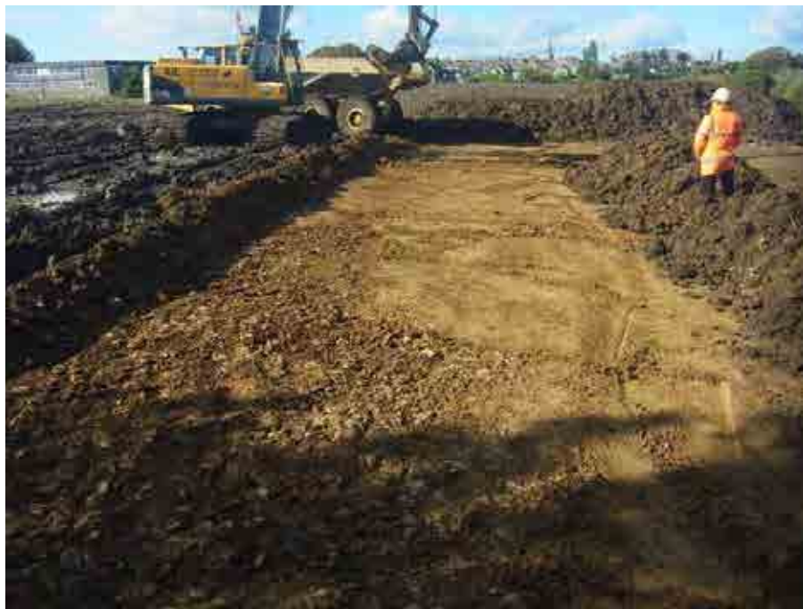
Geological variation observed during watching brief, looking north-west Fig 4
