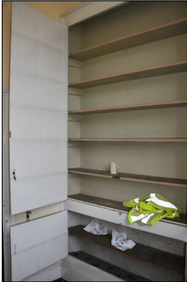
Interior of the cupboards in the Service Room, taken from the east Fig 118
