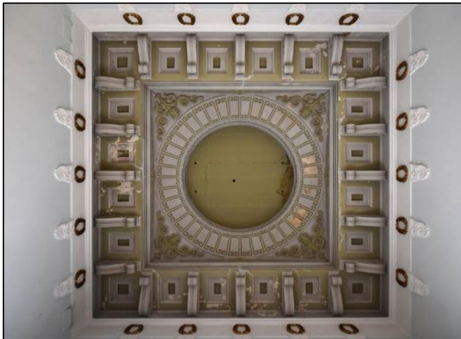
Ceiling in the Reading Room, looking up Fig 59
