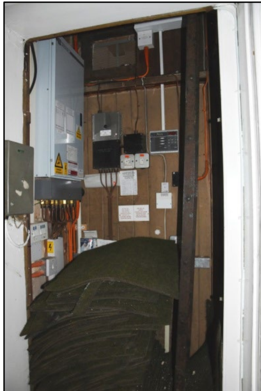
Interior of the service cupboard, taken from the south-west Fig 49
