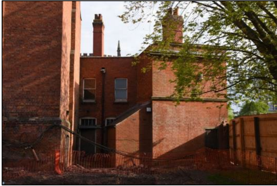
Rear of the Summoner's house, taken from the south Fig 28
