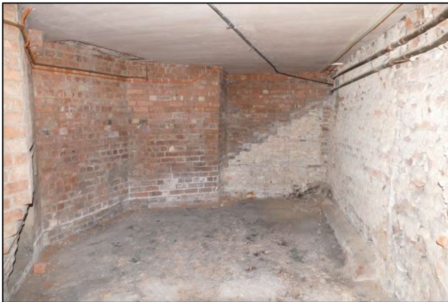
South end of the Store, taken from the north Fig 168
