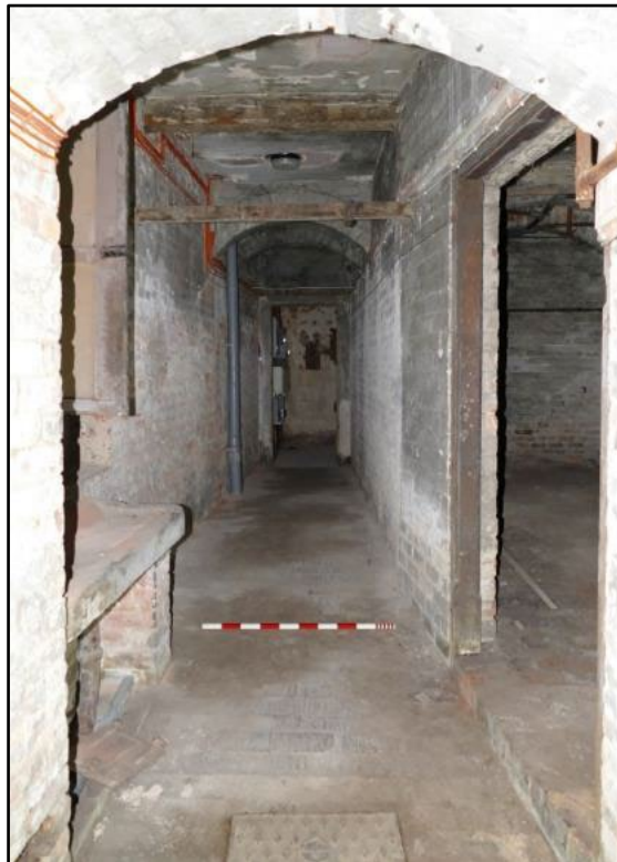
Basement Corridor, taken from the south Fig 155
