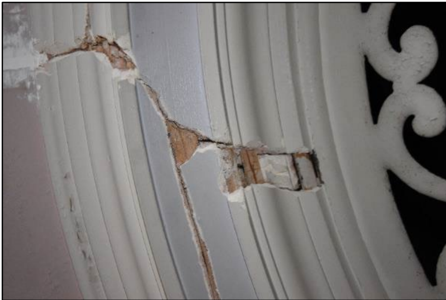
Carved timberwork beneath the ornate mouldings, looking north-west Fig 81
