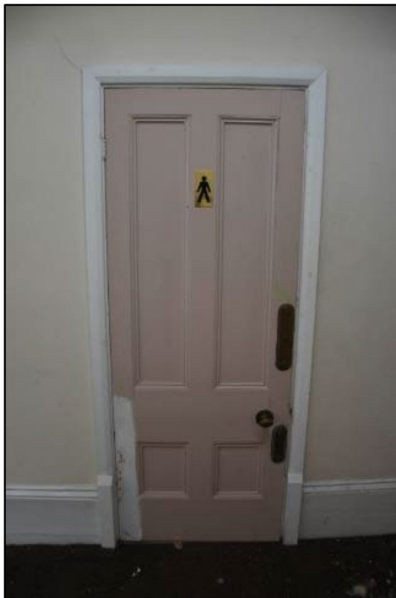
Door to the WCs, taken from the north Fig 90
