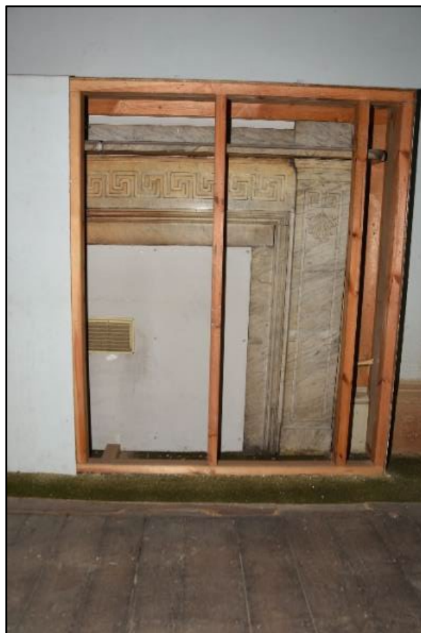
Exposed fireplace in the Billiard Room, taken from the east Fig 67
