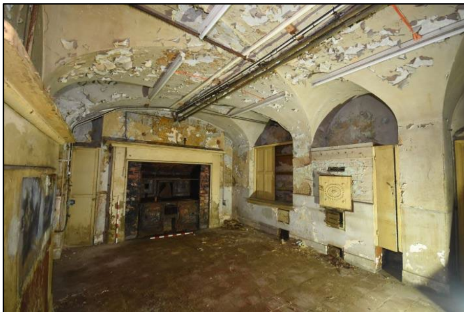
Interior of the Kitchen, taken from the north-east Fig 138
