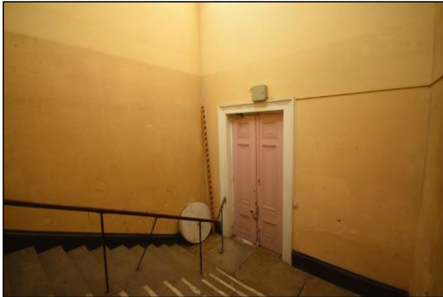
Interior of the Vestibule, taken from the south-east
