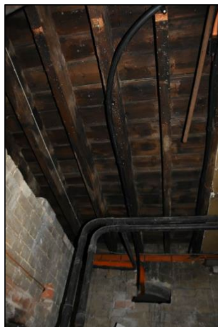
Exposed ceiling in the Duct Room, taken from the east Fig 153
