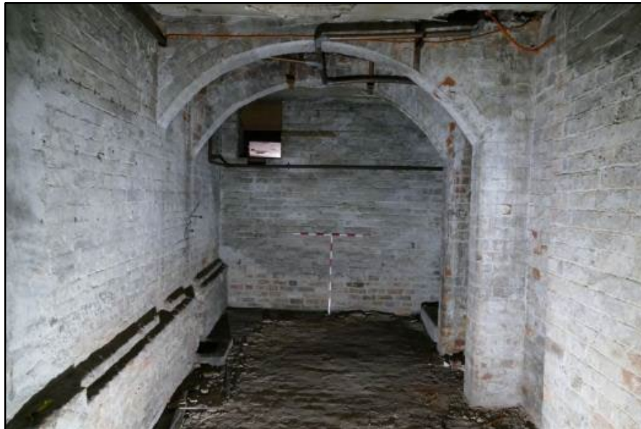
Interior of Store 63, taken from the south Fig 159
