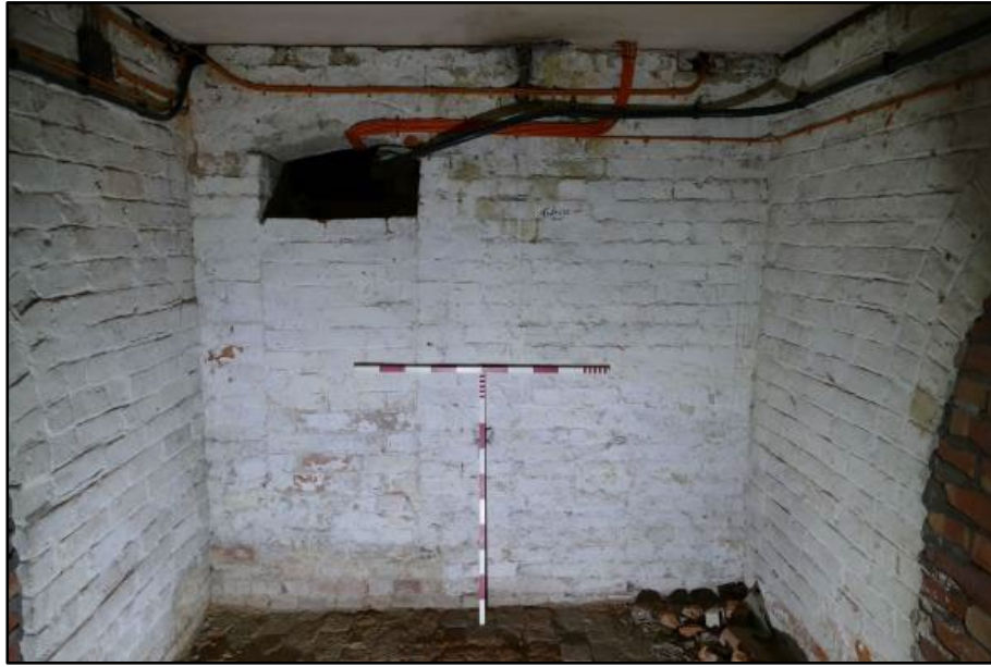
Blocked aperture in Store 70, taken from the west
