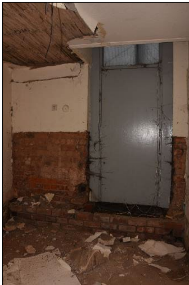
Lobby area during monitoring phase of the project, looking east Fig 182
