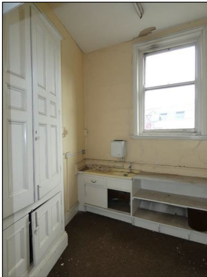
Interior of the Service Room, taken from the west Fig 117
