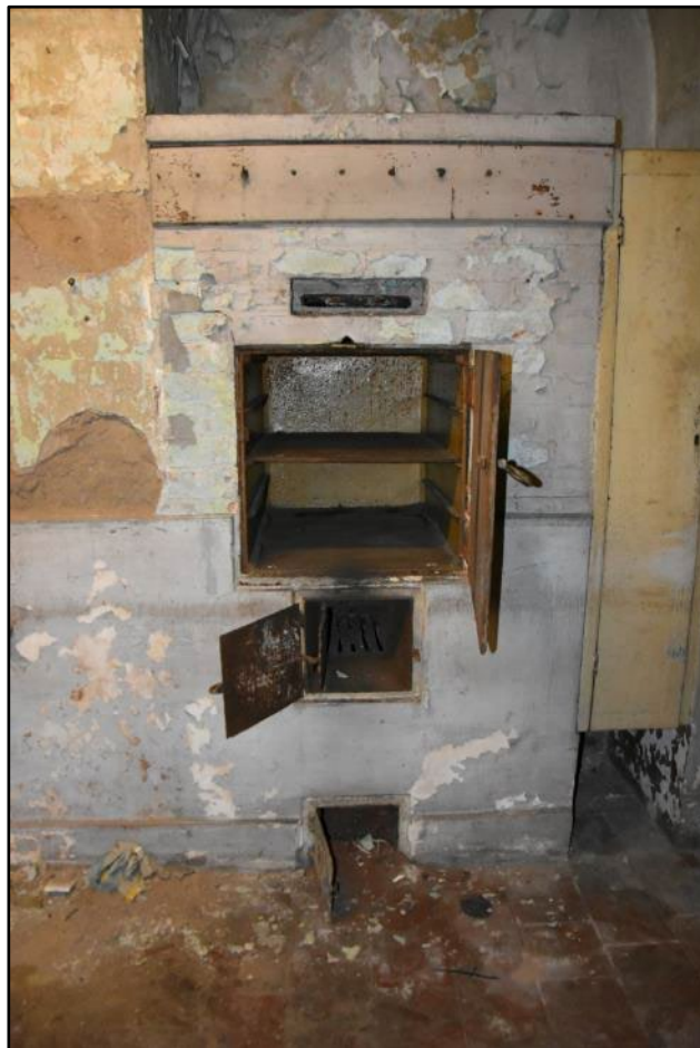
Oven-type structure in the Kitchen, taken from the east Fig 142
