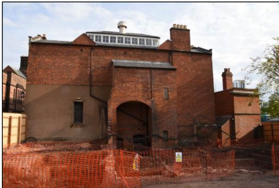
South elevation of the 1830s range, taken from the south Fig 29
