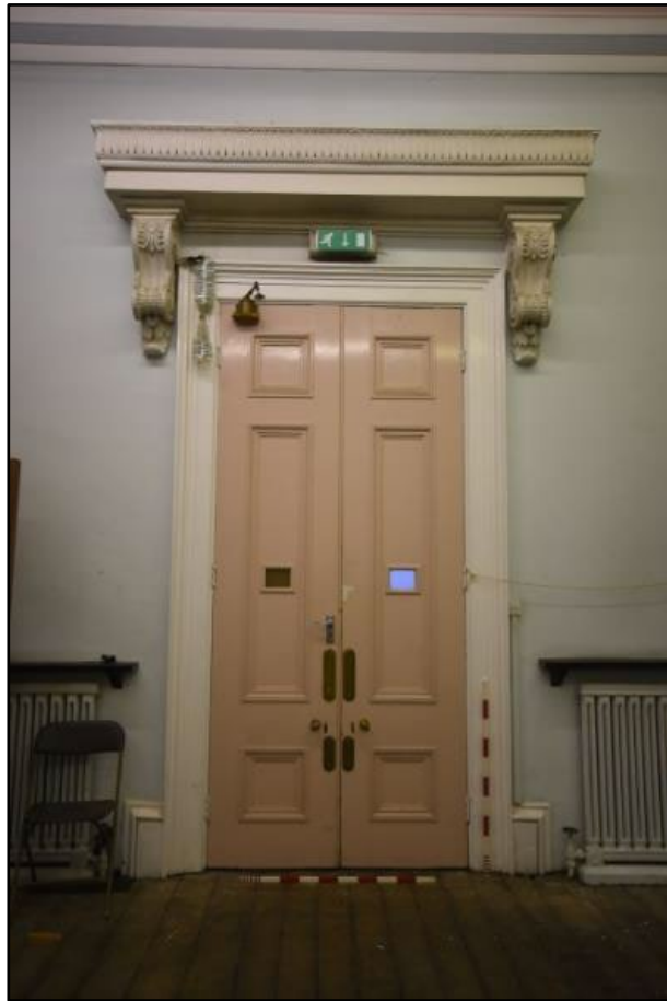
Doors to the Central Corridor from the Tea Room, taken from the west Fig 68
