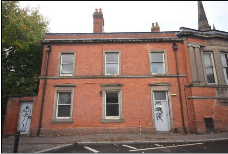
Sumner's House, part of the 1890s range, taken from the east Fig 25
