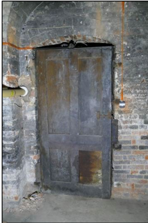
Door providing access into the Former Coal Store, taken from the west Fig 130
