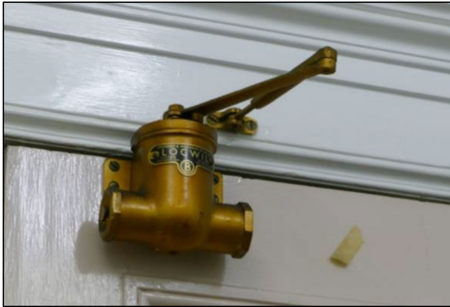
Brass door closer in the Tea Room, taken from the south
