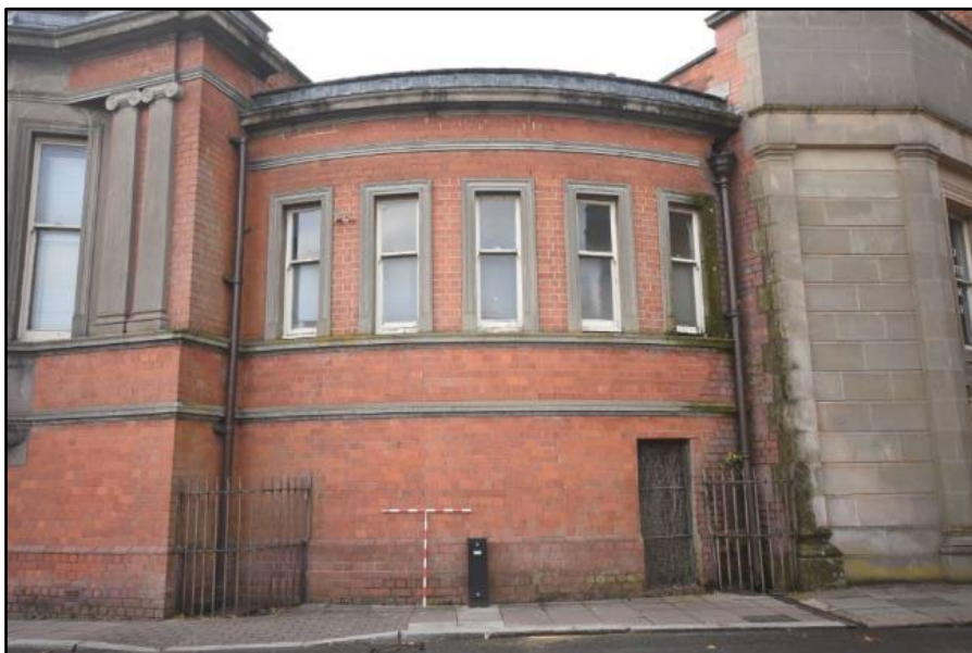
Curved sanitary block of 1890s range, taken from the north-east Fig 22
