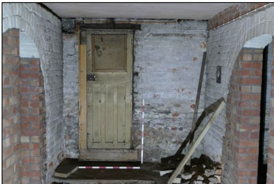
Door to exterior in Store 72, taken from the east Fig 149
