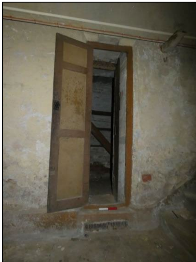
Door into Store from the Corridor, taken from the south-west Fig 125
