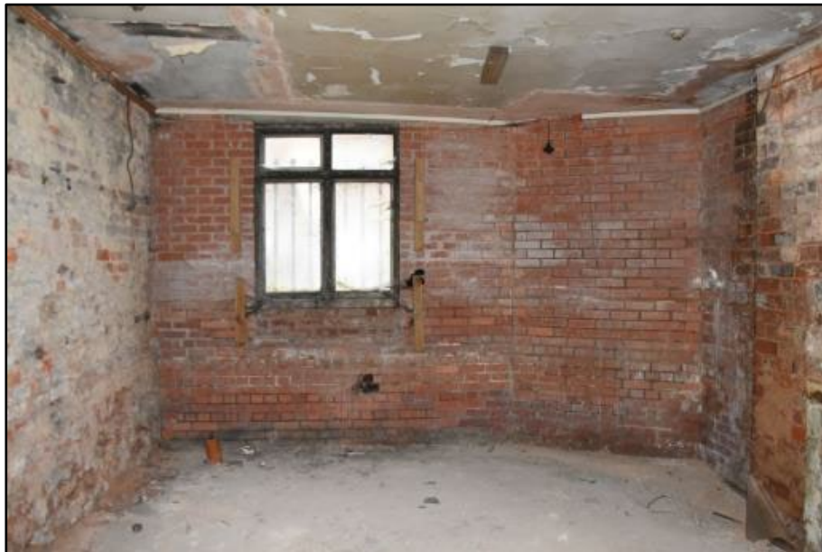
North wall of the Coachmen's Waiting Room, taken from the south
