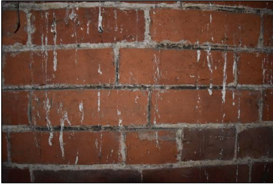
Tuck pointing to the brickwork within the porch, looking east
