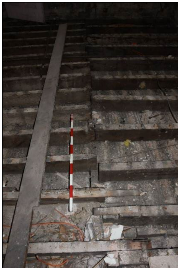
Arrangement of joists in the kitchen on lifting of floorboards Fig 87
