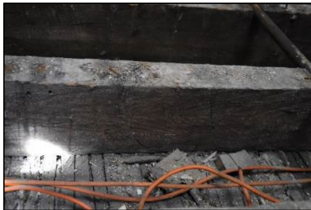
Scribed or scratched markings to the joists Fig 89
