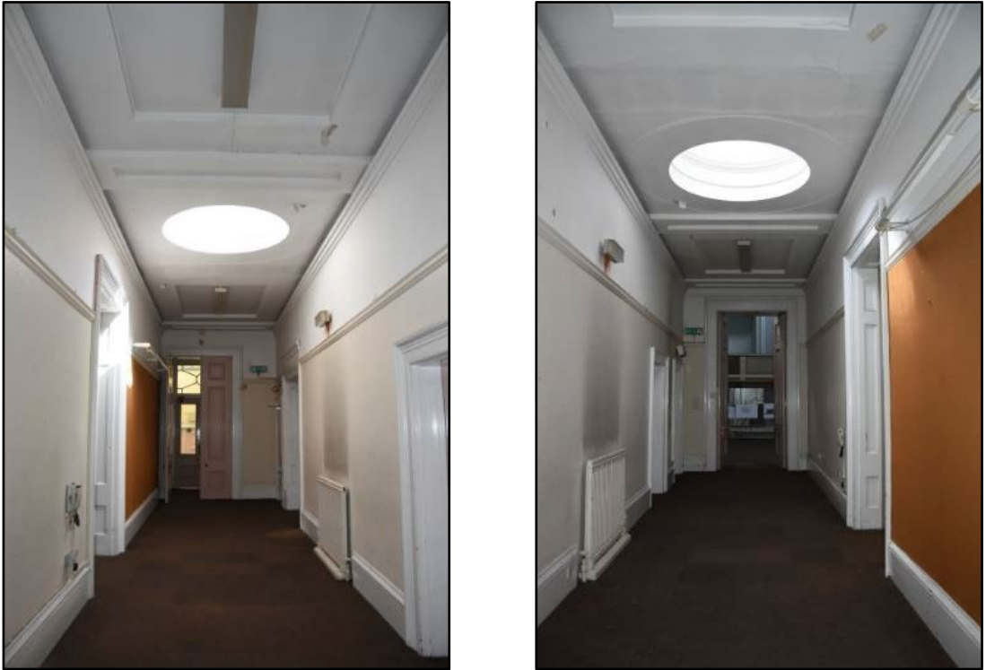
The Central Corridor taken from the south (left) and north (right) Fig 48
