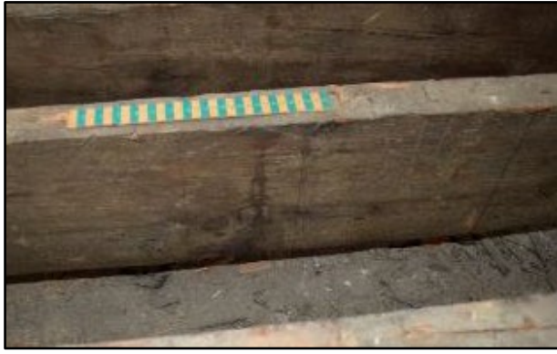
Examples of scribed/scratched timber marks in the Ballroom
