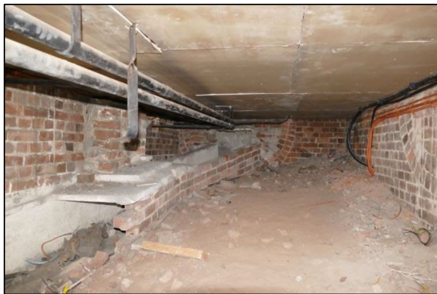
Interior of the Duct Room, taken from the south Fig 152
