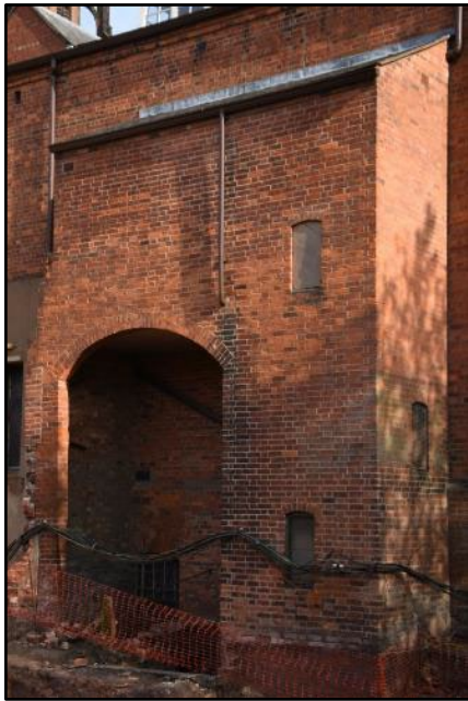
Brick porch giving access to the 1841 orchestra pit within the ballroom, with arch indicated, taken from the south-east Fig 30
