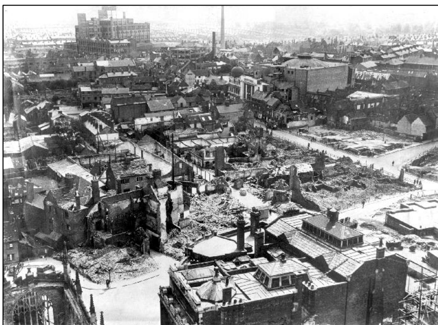
Photograph of Drapers Hall (foreground) following November 1940 blitz, source unknown Fig 13
