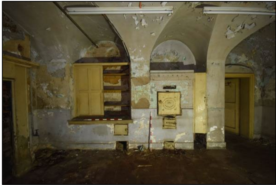
West wall of the Kitchen, taken from the east Fig 141
