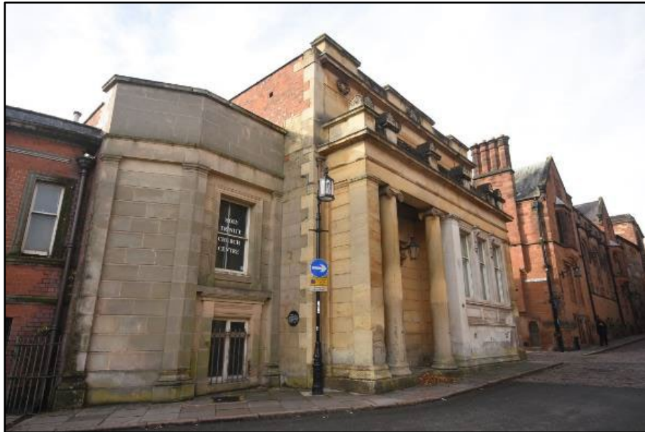
The north elevation of the 1860s range, taken from the north-east Fig 21
