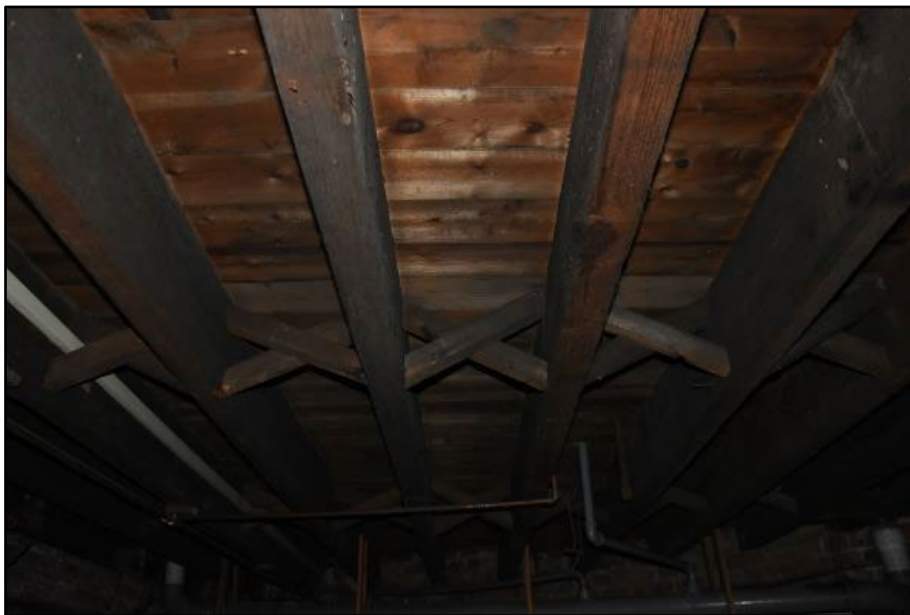
Ceiling in the Coachmen's Waiting Room, taken from the south Fig 172
