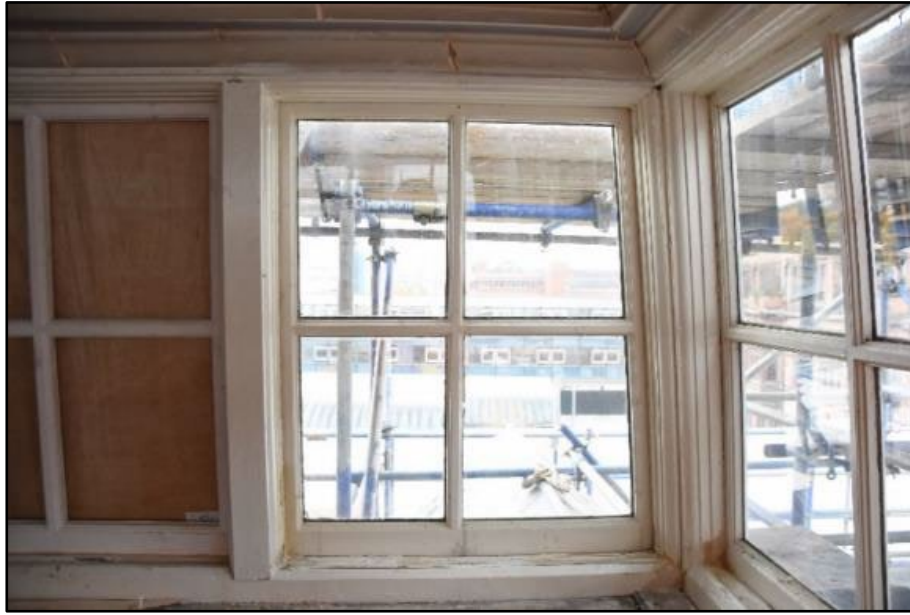
Timber windows to the roof lantern, looking north Fig 78
