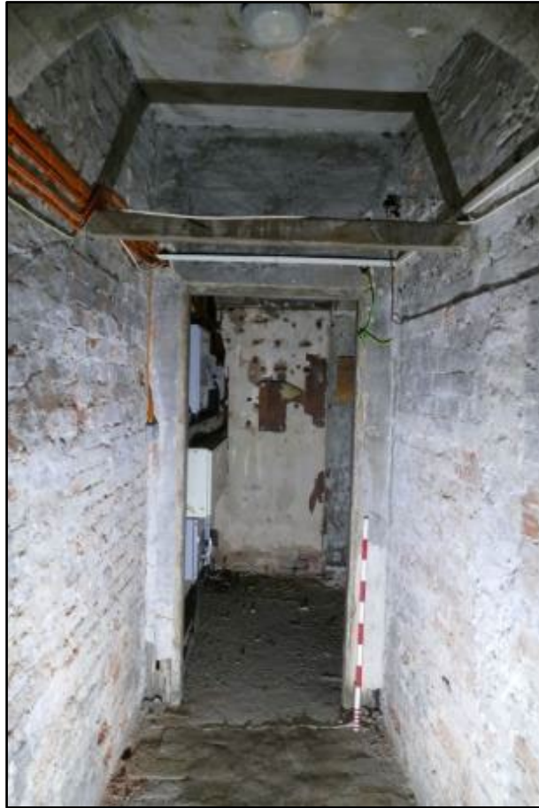
North end of the Basement Corridor, taken from the south
