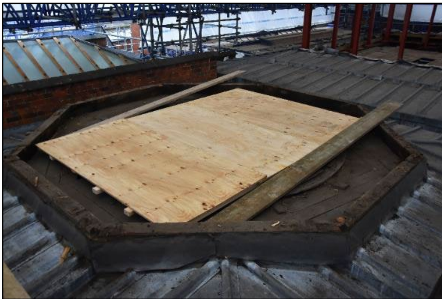
Exposed timber frame to the Reading Room lantern, looking south-east Fig 41
