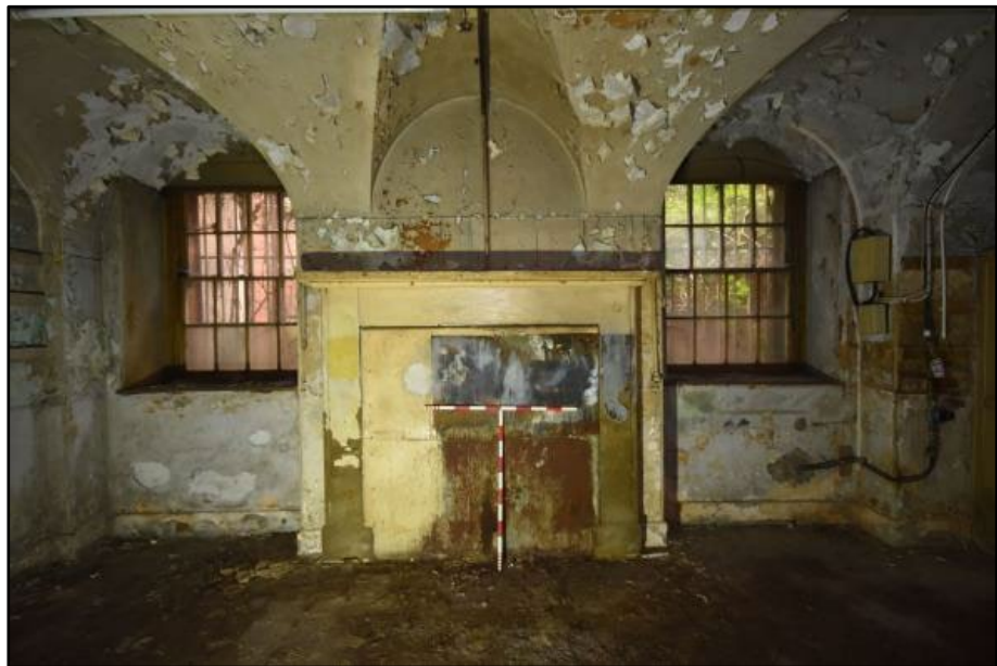
East wall of the Kitchen, taken from the west Fig 140
