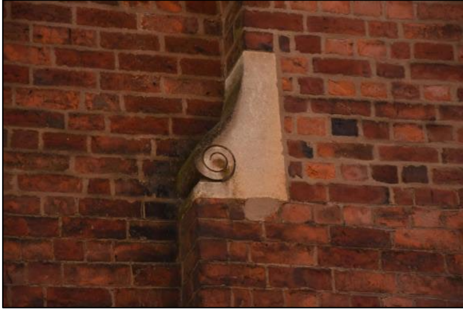
Detail of stone shoulders to chimney stacks along west elevation, taken from the west Fig 34
