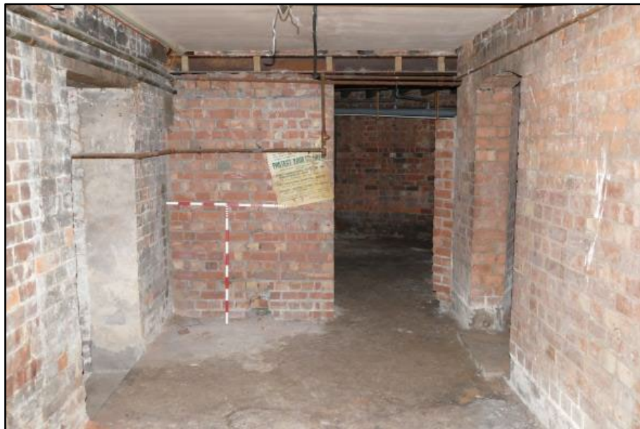
North end of the Store, taken from the south
