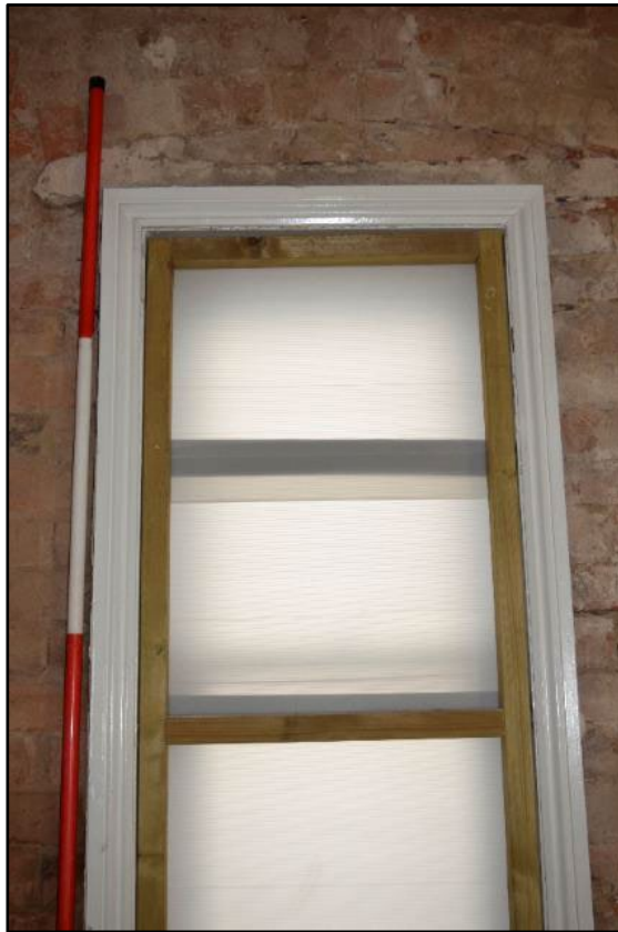
Brickwork exposed during the monitoring phase, looking north-east
