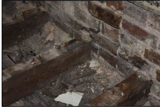
Arrangement of joists meeting the south (left) and north (right) wall
