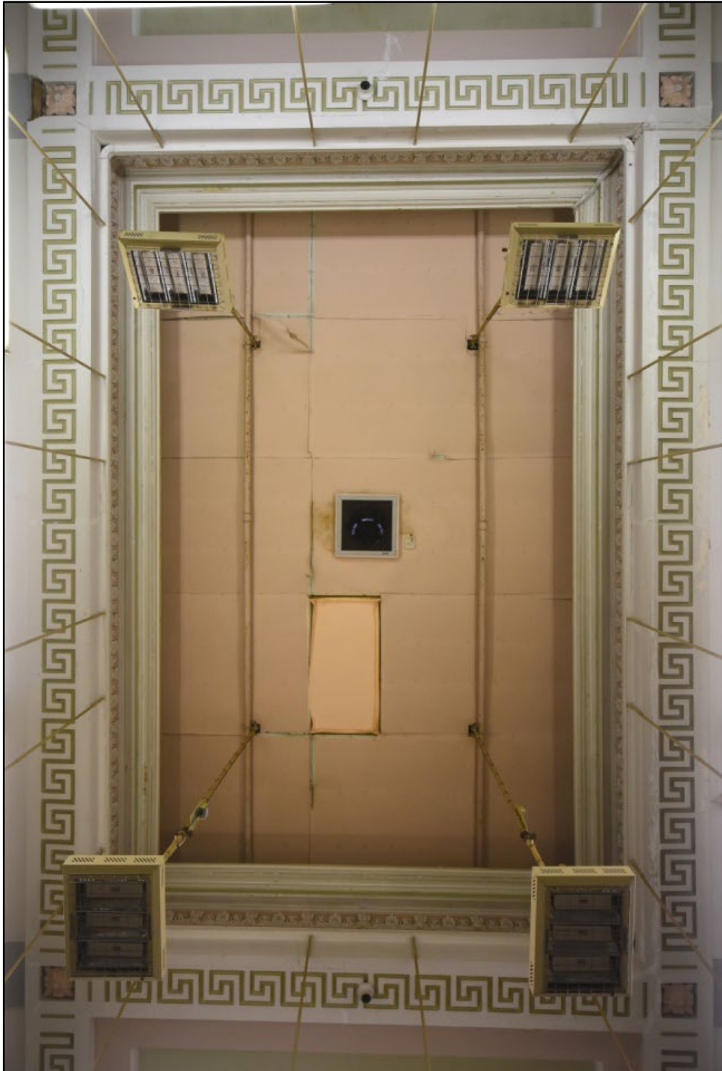
Central section of the ceiling in the Tea Room Fig 69
