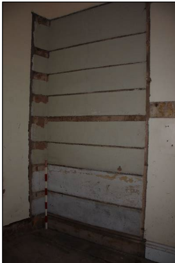
Cupboard area following soft strip, looking east Fig 121
