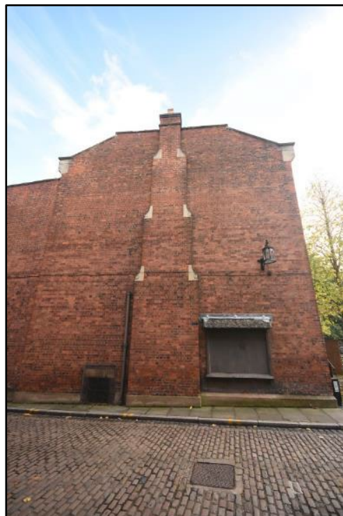
Gable end of the 1830s range, taken from the west
