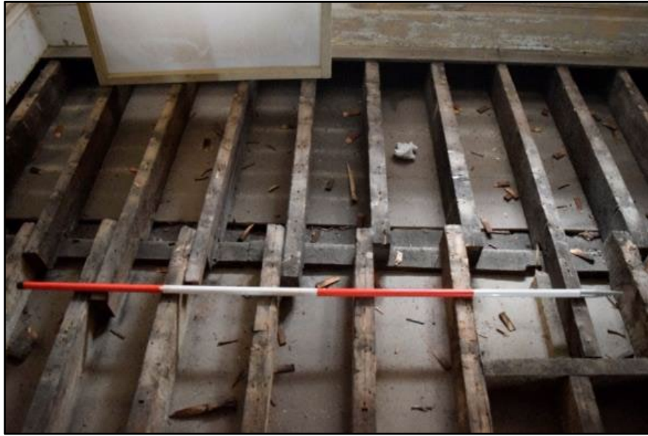
Floor joists in the Reading Room showing the distinction between the main room (bottom) and the extended north bay (top) taken from the south Fig 56
