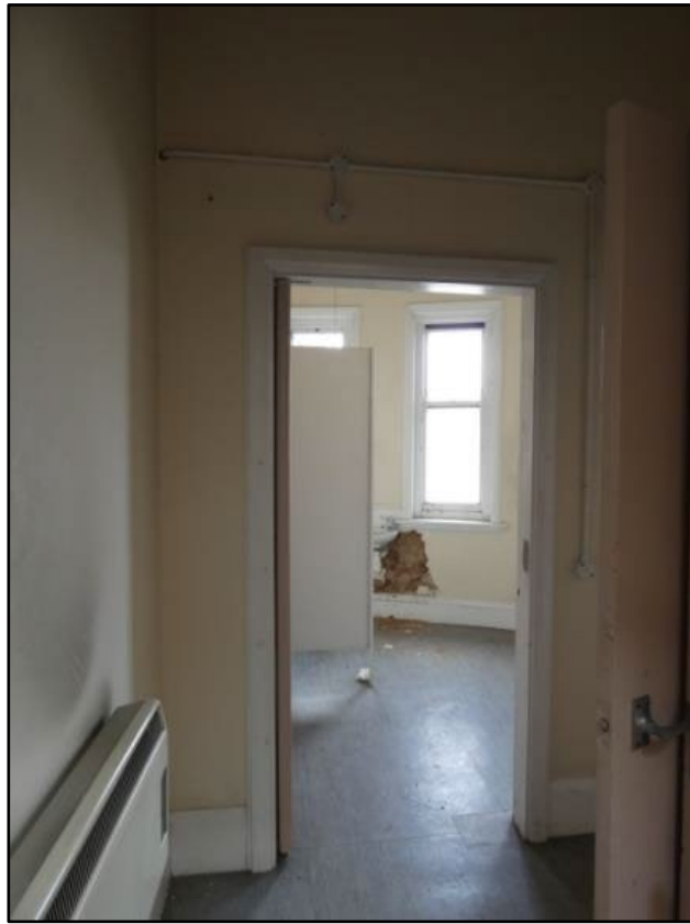
Interior of the Former Restrooms, taken from the south Fig 103
