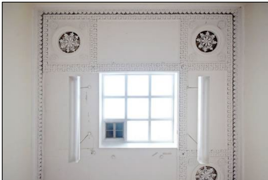
Ceiling in the Kitchen, looking up
