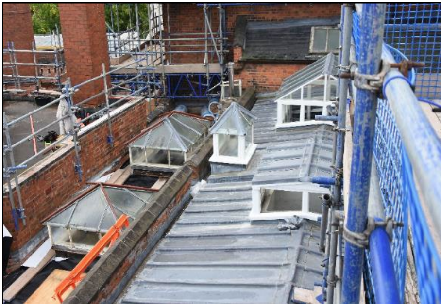
Roof over the 1860s range, looking south Fig 39
