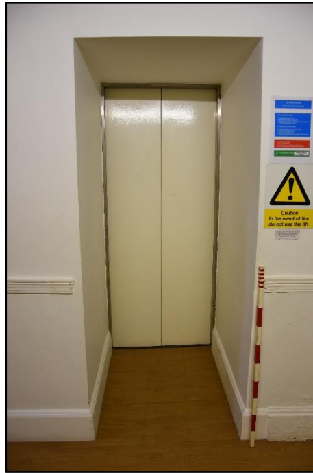
Access to the lift from the stair hall (GF01), looking east Fig 45
