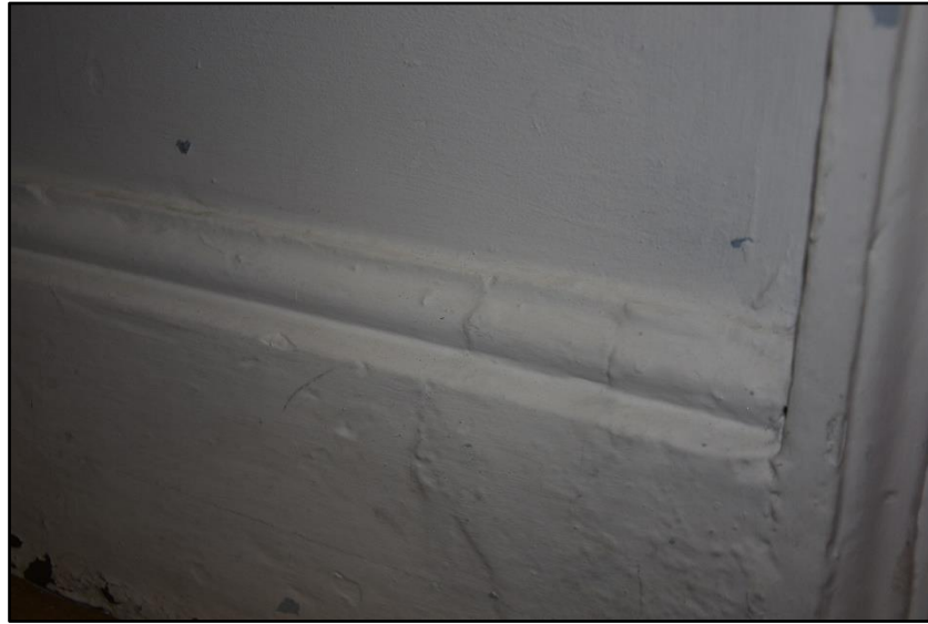
Ovolo-moulded skirting in the stair hall (GF01), looking south Fig 47
