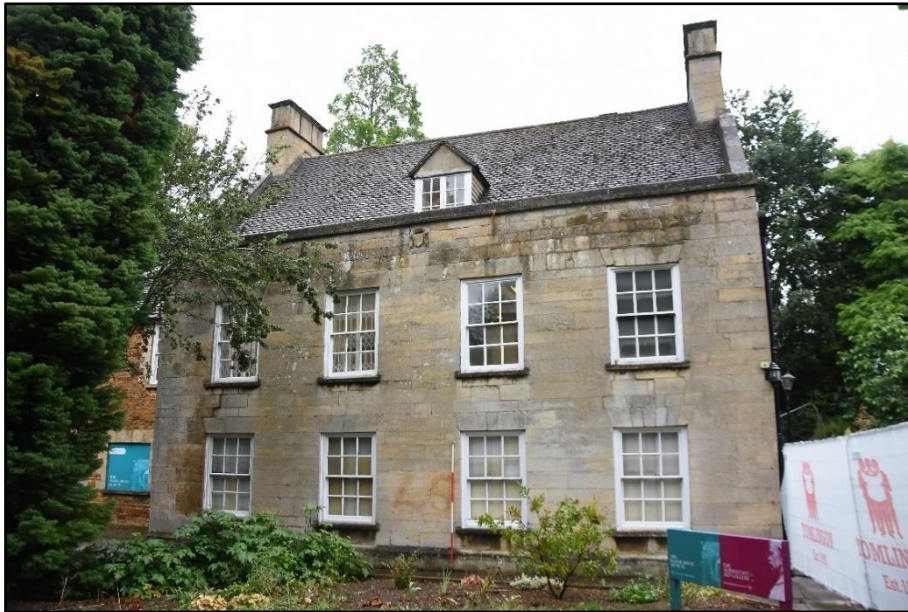
View of the west elevation of the main range, looking north-east Fig 17
