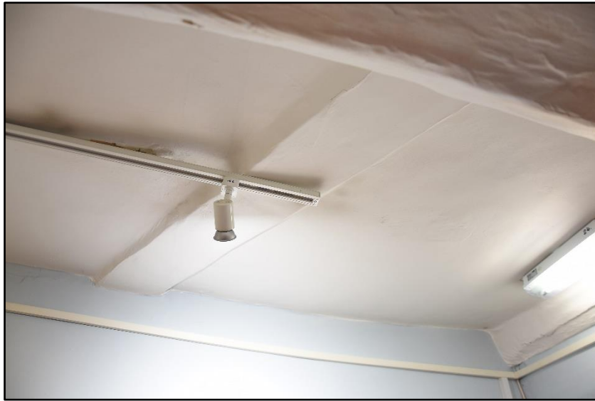
Diagonal beam in FF02, looking west Fig 73
