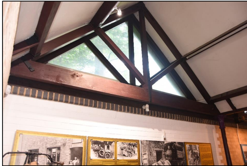
King-post roof structure of GF06, looking east Fig 61
