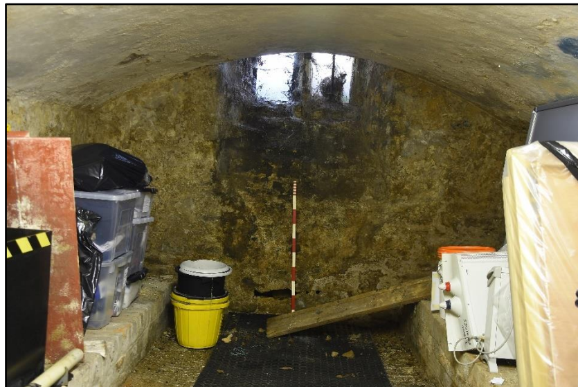
Basement below the main range, looking east Fig 36
