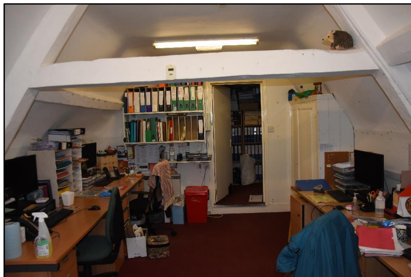
Office space (SF04) over the rear range with truss exposed, looking west Fig 94
