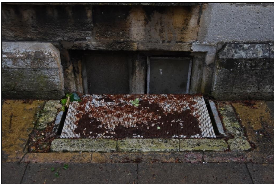
Basement light to the west elevation, looking east Fig 18
