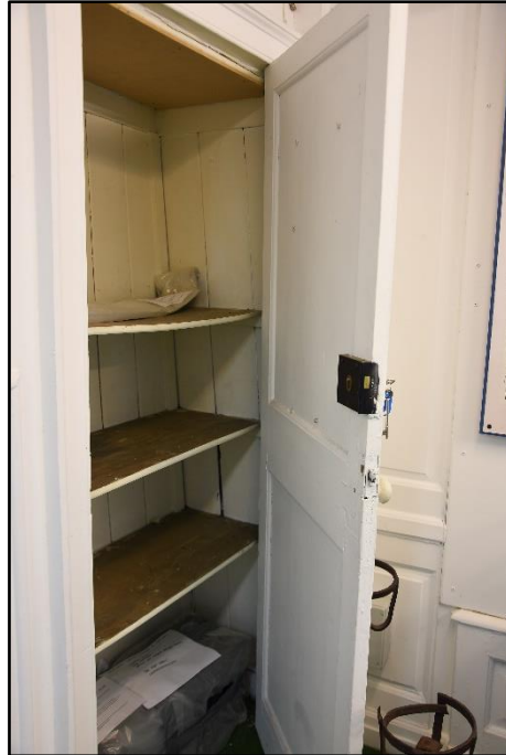
Interior to the cupboard in FF03, looking south-west
