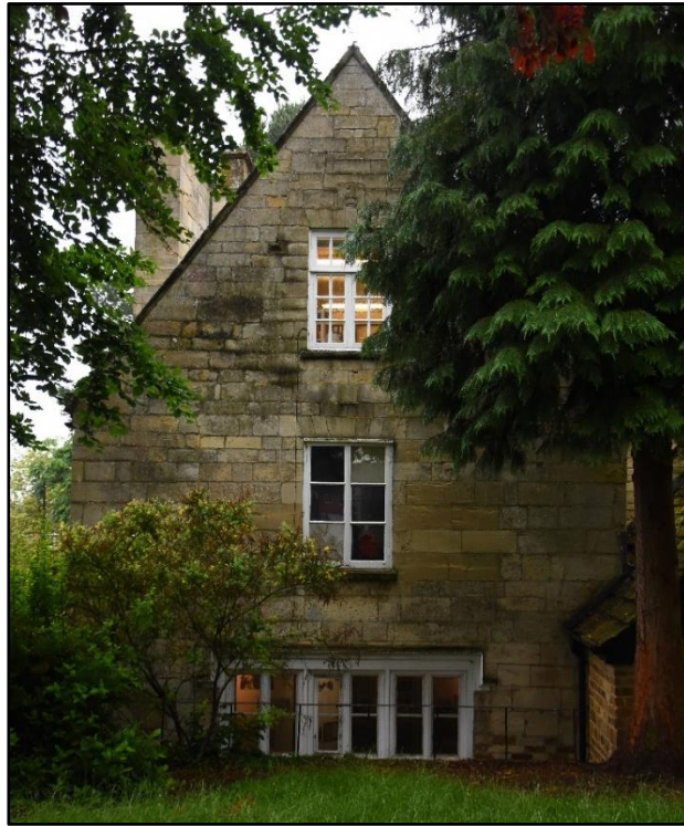
East elevation of the rear range, looking west Fig 26
