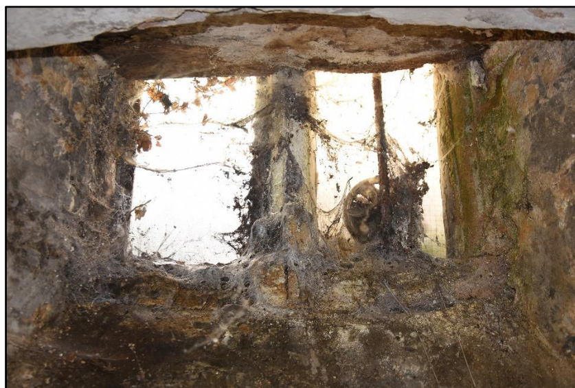
Basement window, looking east Fig 38
