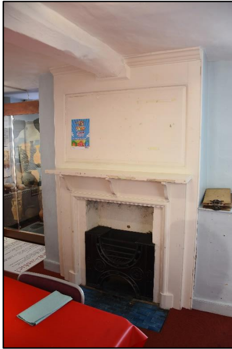
Chimney stack in the blue exhibition room (FF02), looking south-east Fig 71
