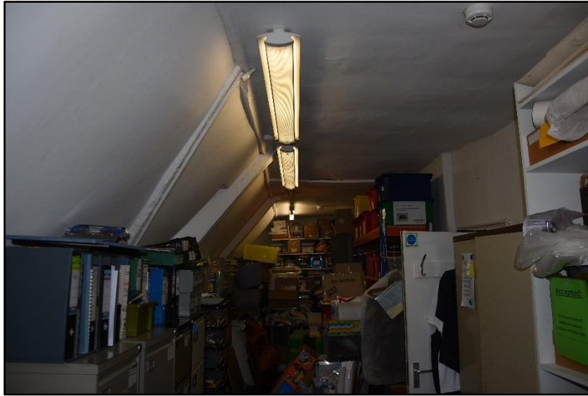
View of the storeroom on the second floor (SF02), looking north Fig 89
