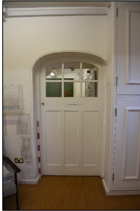
Door giving access to the stair hall from the lobby (GF03), looking south Fig 41
