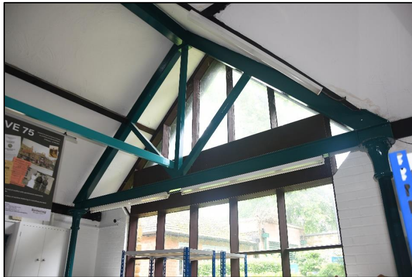
King-post roof structure in cast-iron in GF06, looking north-west Fig 62
