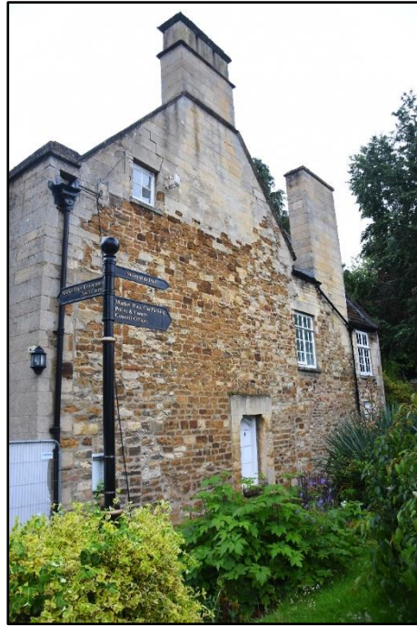
View of the south elevation of the main and rear ranges, looking north-east Fig 29
