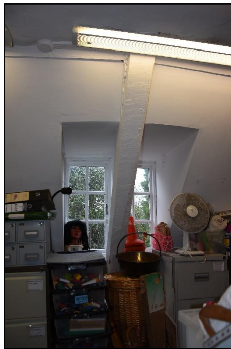
Rafter to the roof over the main range in SF02 cutting a dormer window, looking west Fig 90
