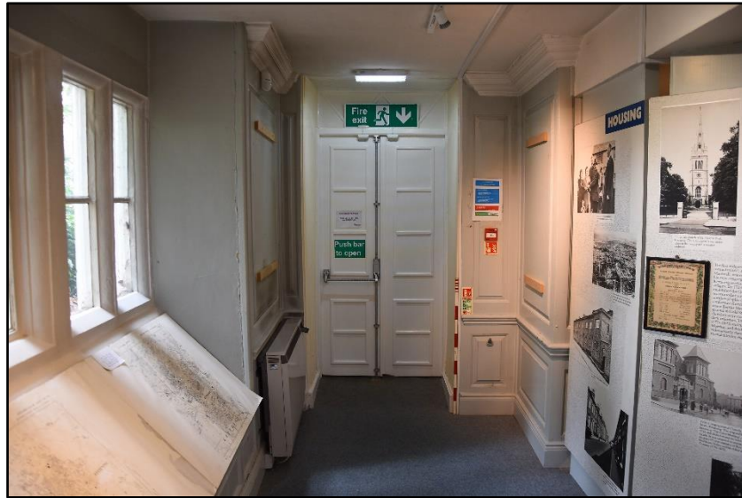
Fire door visible within GF03, looking south Fig 59
