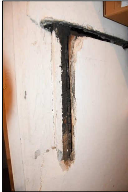
Stud and rail exposed within the cupboard (SF03), looking north-east Fig 93
