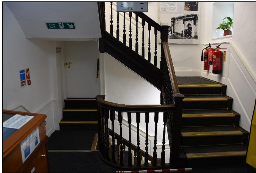
View of the landing to the first floor (FF01), looking north Fig 66
