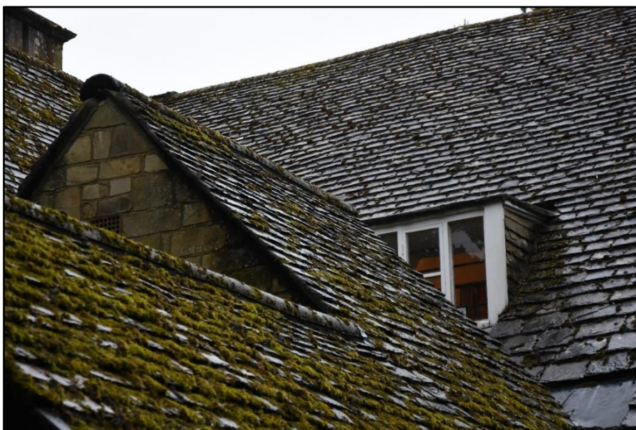
Stone extension to the east elevation, looking south-west Fig 24
