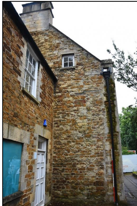
View of the main range's north elevation, looking south Fig 22
