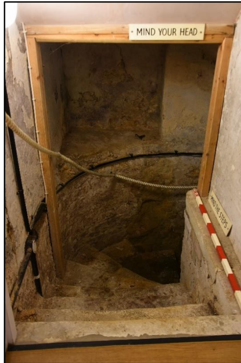
Stairs descending into the basement, looking west Fig 35
