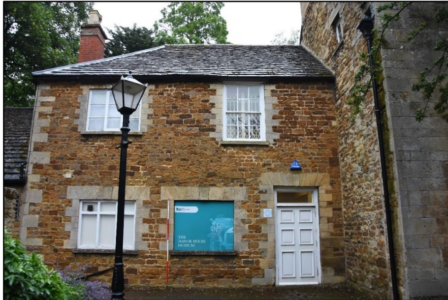
View of the west elevation of the north range, looking east Fig 19
