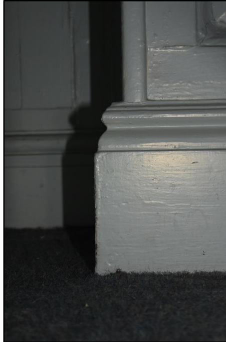
Skirting profile in the green museum space (GF03), looking west Fig 55
