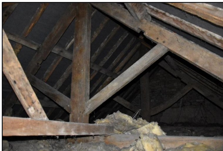
Roof structure over the north range, looking south-east Fig 96
