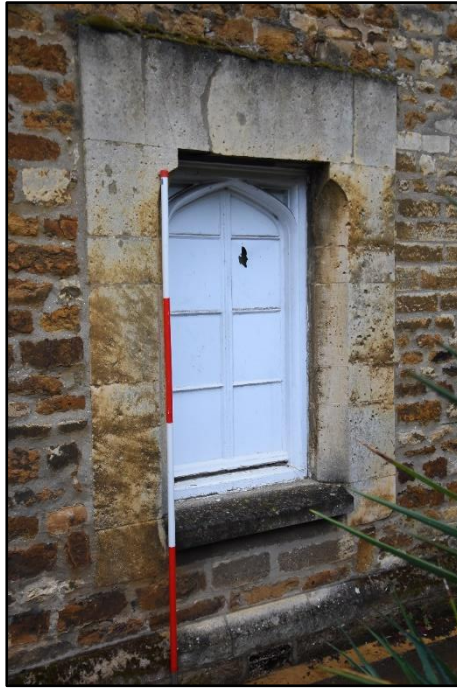
Painted window on the south elevation of the main range, looking north-east Fig 31
