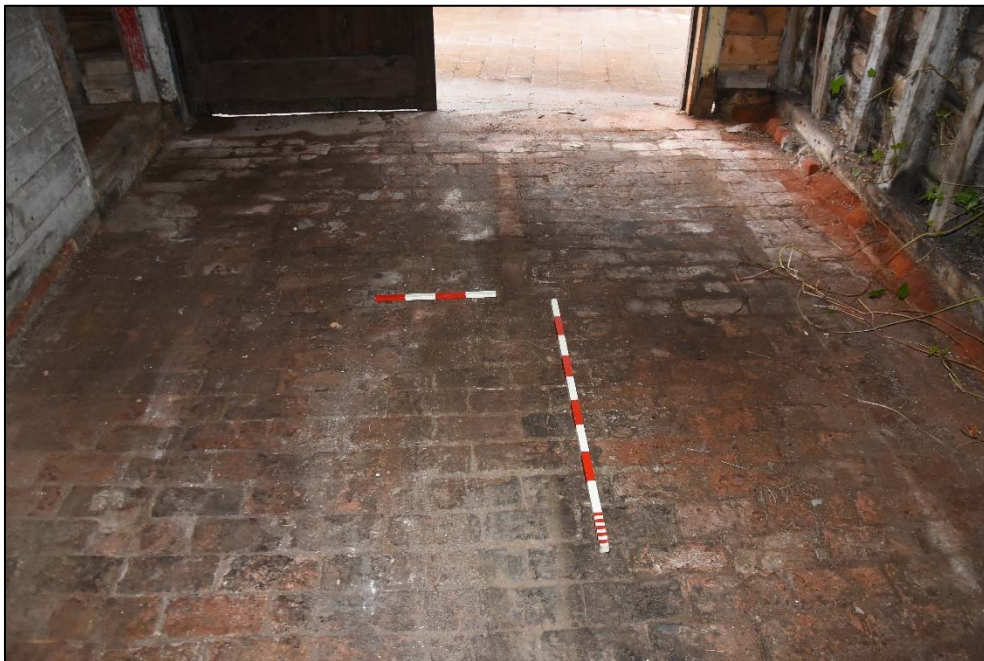
The brick floor to Store A, looking south Fig 8
