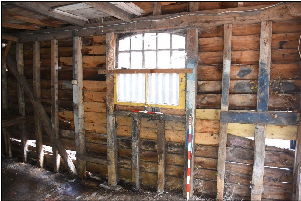
East timber stud wall to Store C, looking north-east Fig 27
