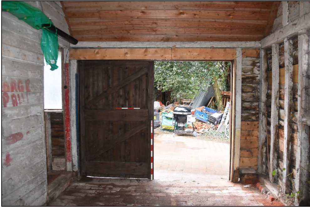
South wall of Store A, showing double doors, looking south Fig 9
