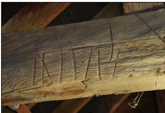
Timber marks on the south face of the tie-beam (left) and common rafter to the west pitch (right) in Store D, looking north-west Fig 36
