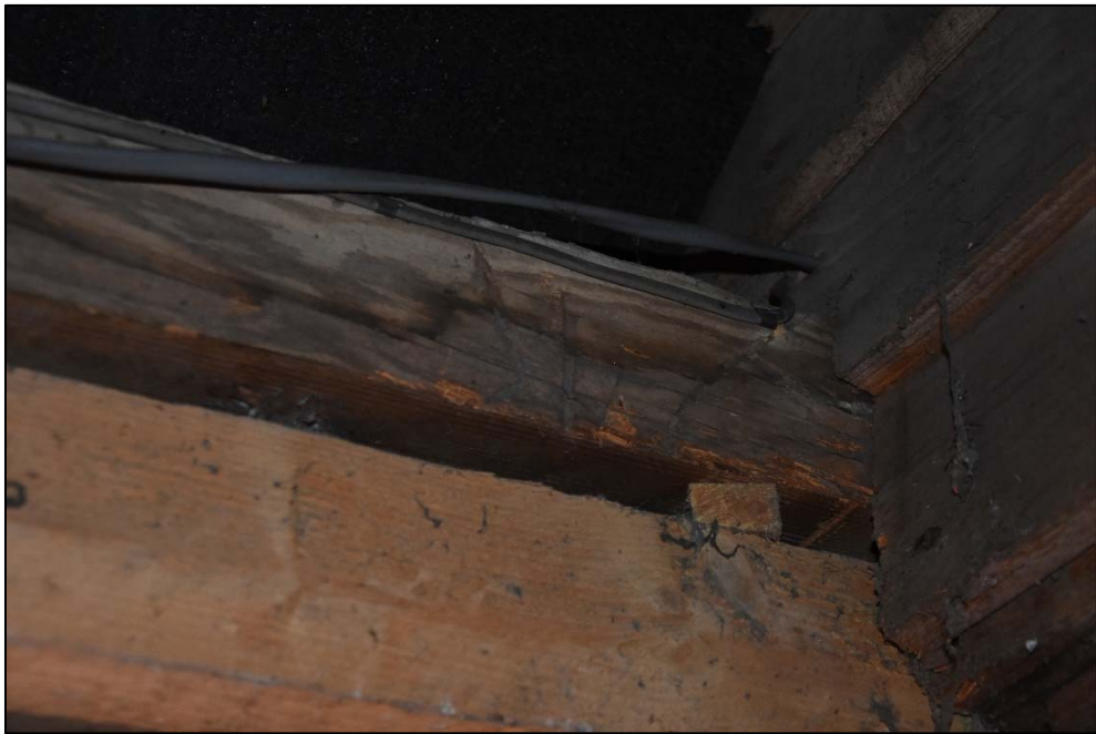
Scribed timber mark to the face of the wall-plate on the south wall of Store C, looking south-east Fig 24
