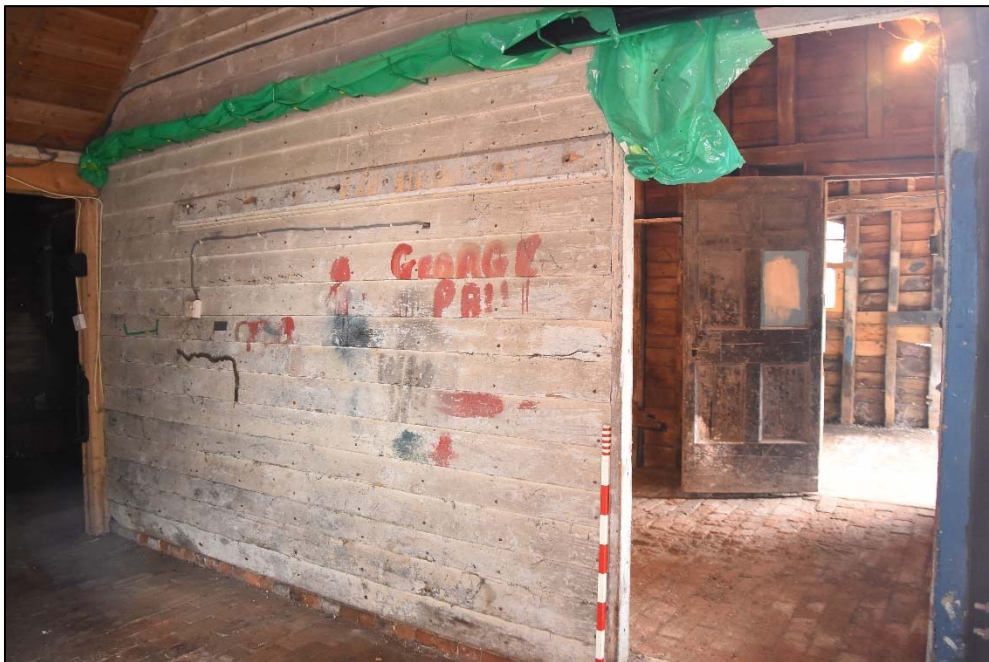
East wall of Store A with weather-boarding and access into Store B, looking north-east Fig 12
