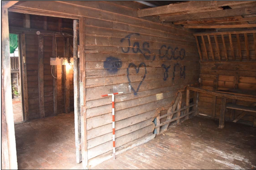
West wall of Store C, looking north Fig 25
