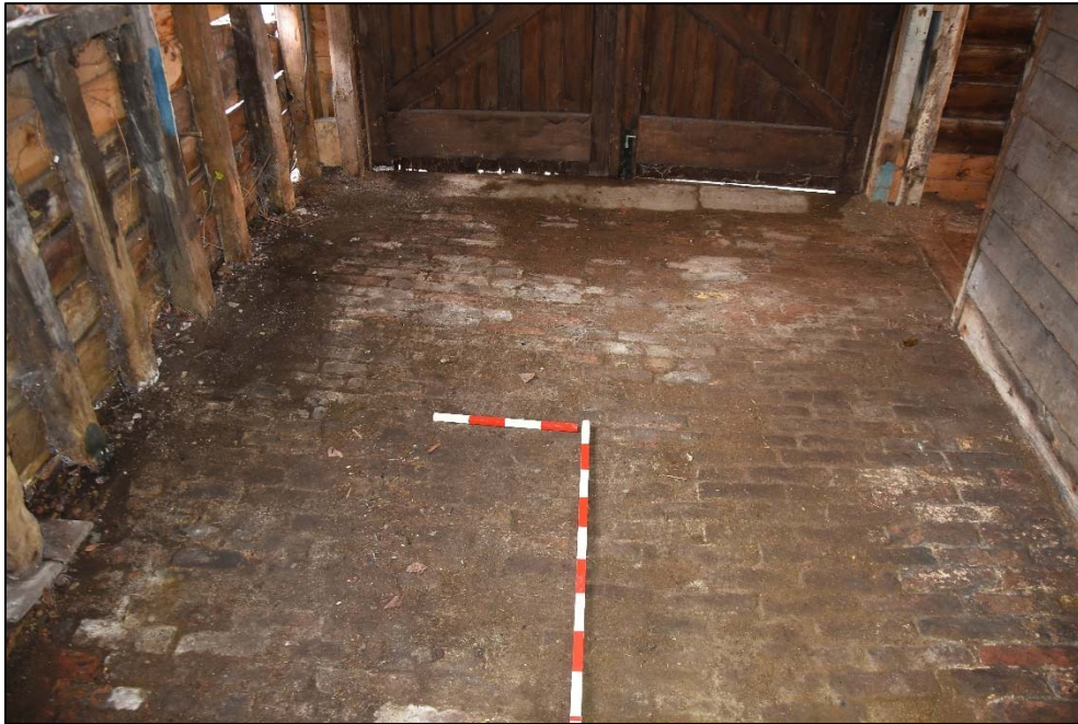
Brick floor in Store C, looking south Fig 22
