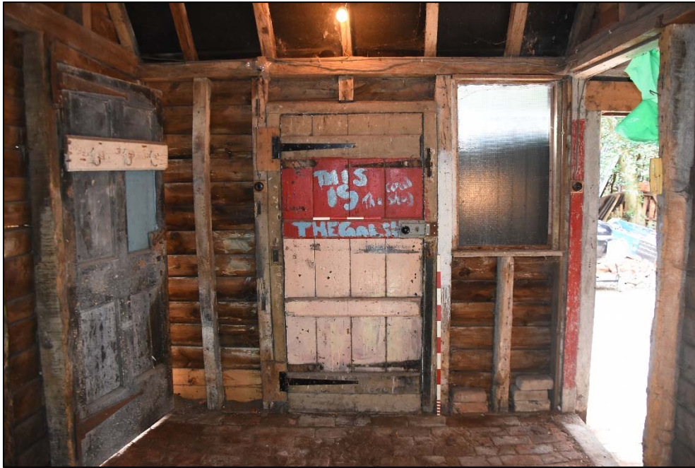
South wall of Store B, looking south Fig 15
