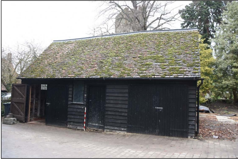
South elevation of the outbuilding, looking north Fig 4
