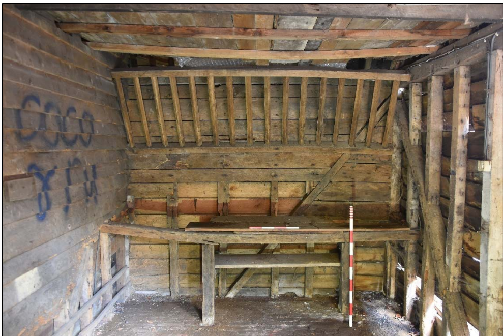
North wall of Store C with hay rack and trough, looking north-east Fig 26
