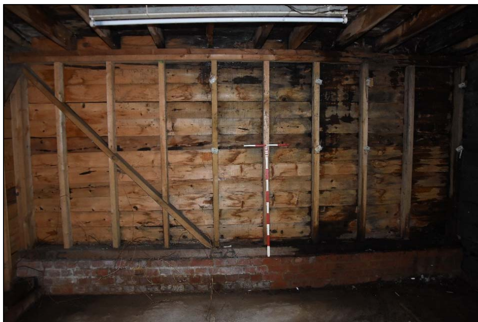
North studwork wall in Store E, looking north-east Fig 38
