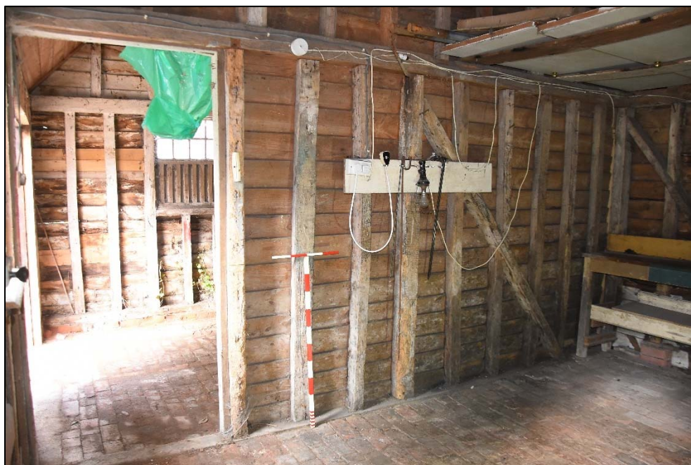
West wall of Store B, looking north-west Fig 16
