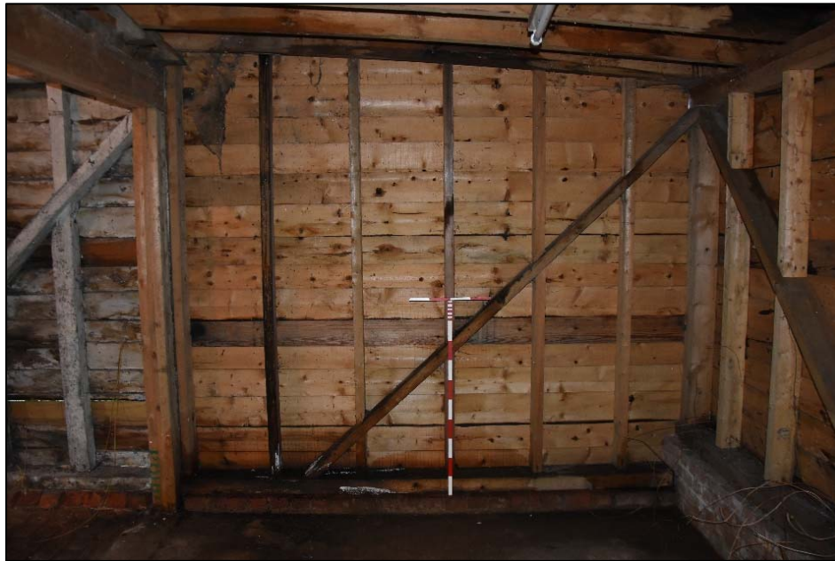
West studwork wall in Store E, looking north-west Fig 37
