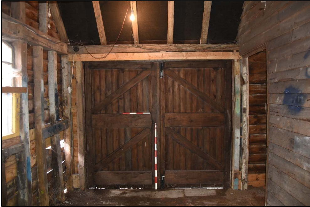
South wall of Store C with double doors, looking south Fig 23
