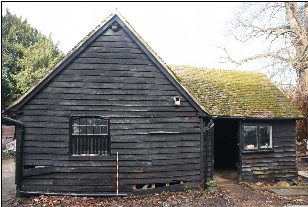
East elevation of the outbuilding with north range extension, looking north-west
