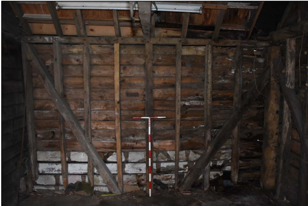
The timber-framed west wall of Store D, looking north-west Fig 33
