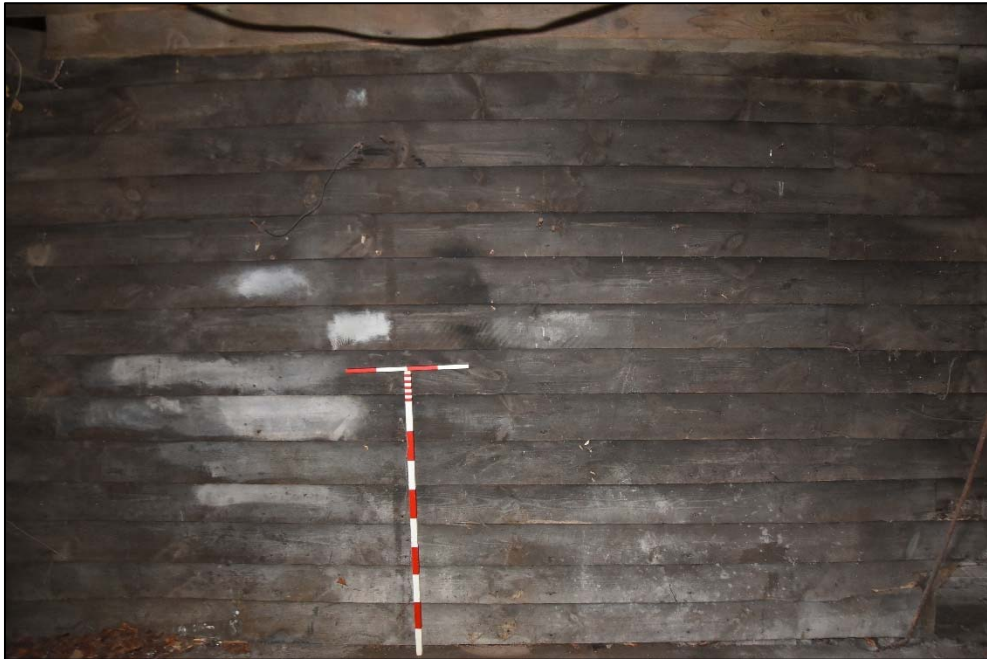
Weather-boarding to the south wall of Store D, looking south-west Fig 31
