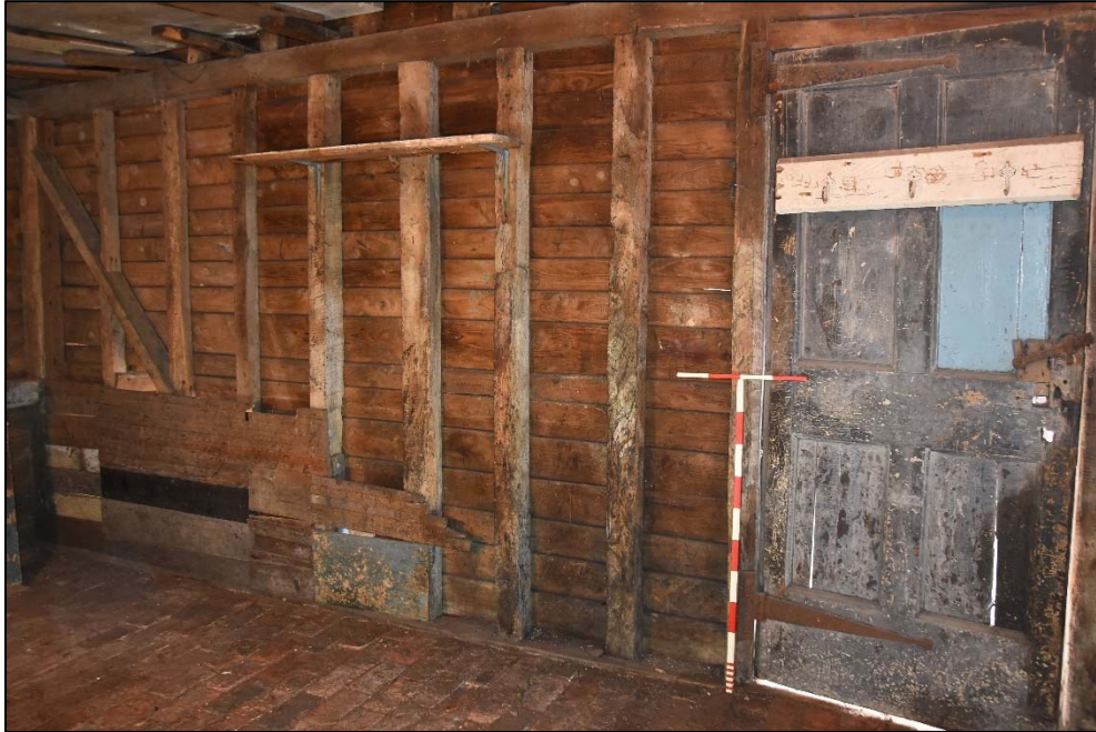
East wall of Store B, looking north-east Fig 20
