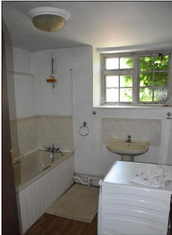
Manager’s flat bathroom (GF20), looking south-west
