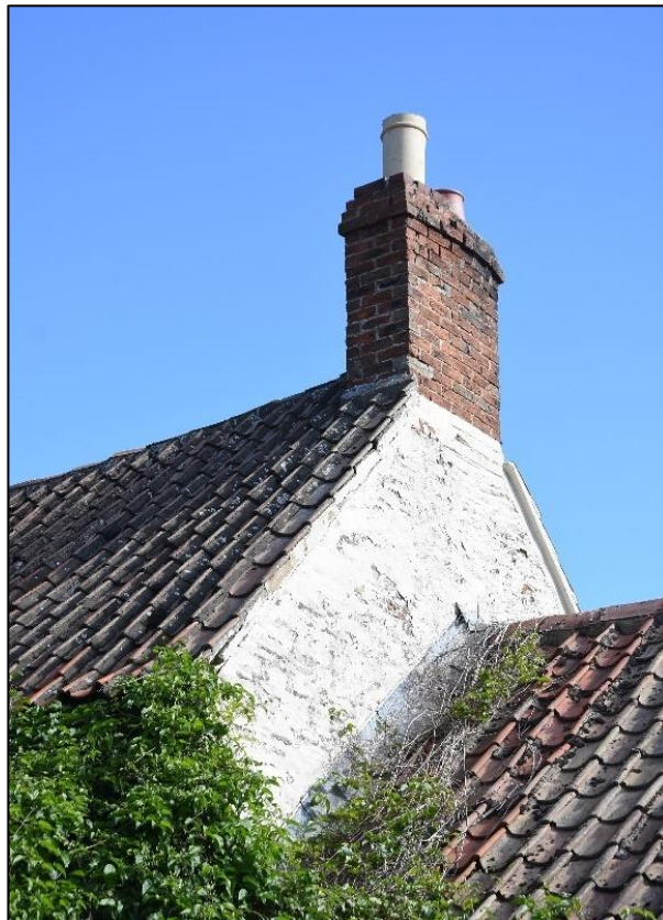
East gable end of Range 1, looking north-west Fig 7
