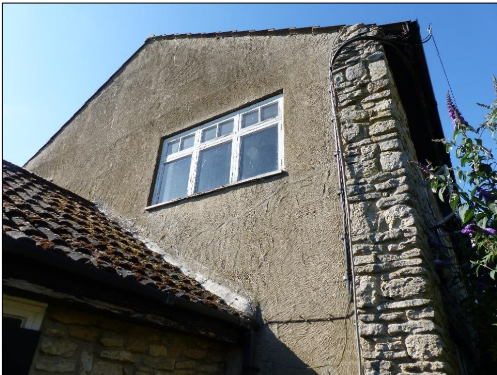
North gable end of Range 5, looking south-west Fig 14
