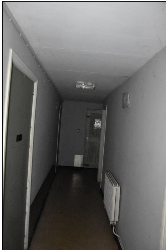
View of the corridor (GF16) looking north-east Fig 53
