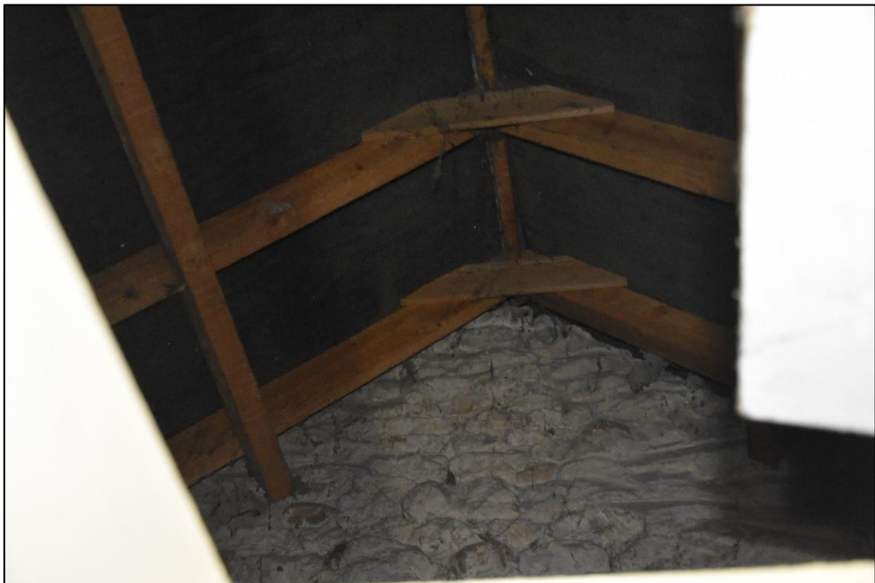
Roof over Range 4 in modern softwood, looking west Fig 103
