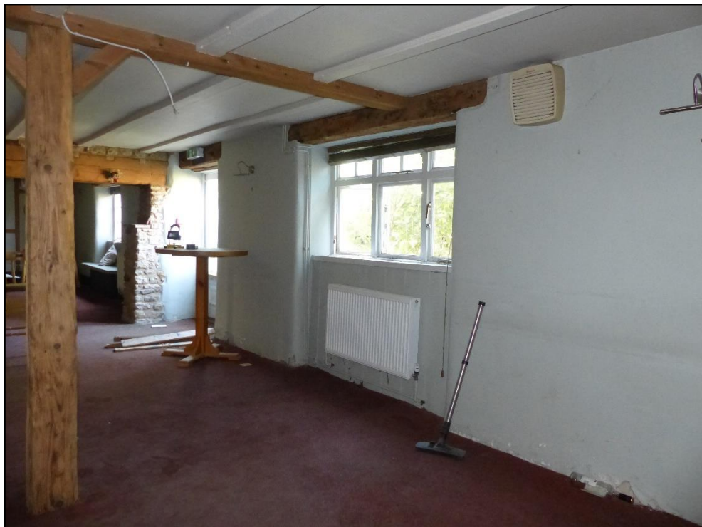
West wall of the lounge (GF02), looking south-west
