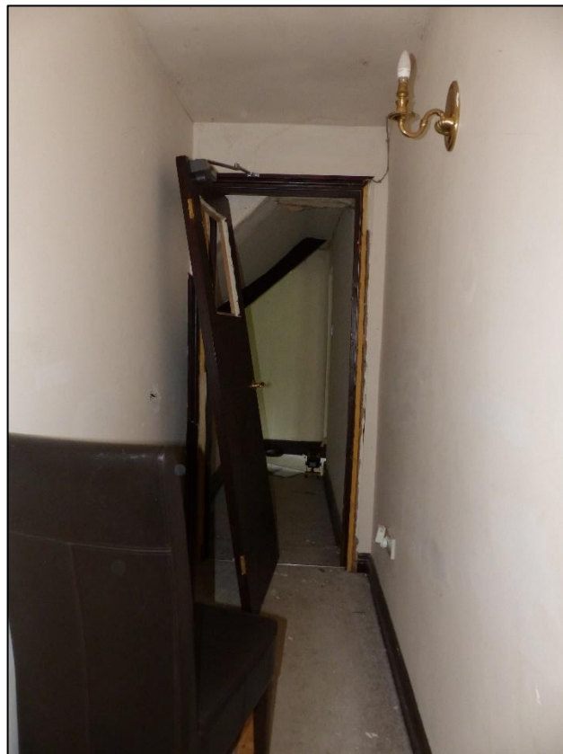
South end of the rear corridor, looking south-west Fig 84
