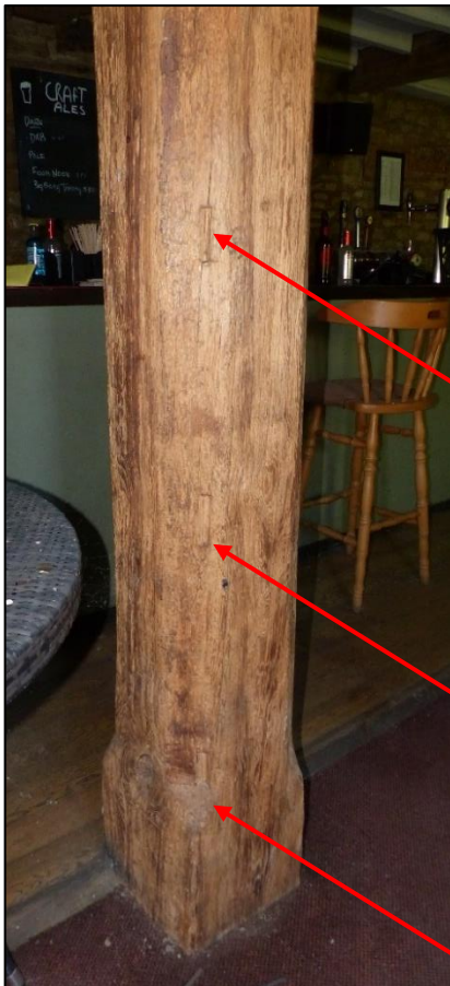
Notches to the post dividing the central and southern bay of the lounge (GF02), looking south-east Fig 30
