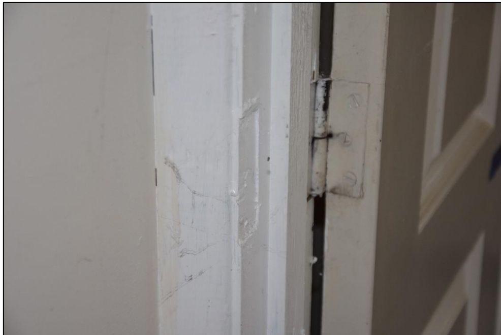
Notch for former door hinge, suggesting door has been re-orientated, or replaced, looking south-west Fig 91
