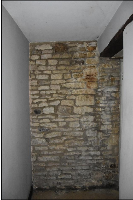
Exposed stone wall of the corridor (GF16), looking south-west Fig 54
