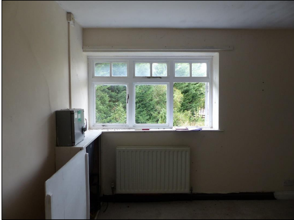
Bedroom to the west of the rear corridor, looking north-west Fig 87
