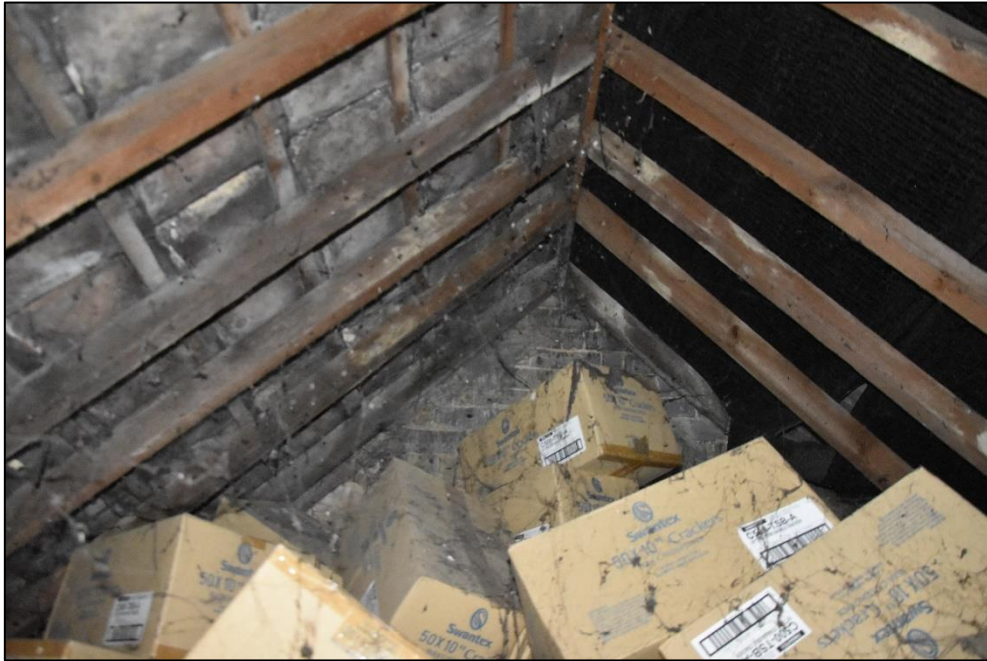
North gable end of the roof over Range 2, looking north-east Fig 98
