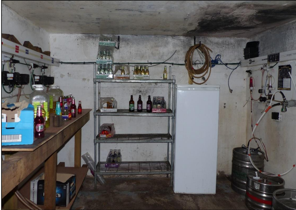
Bar cellar (GF24) interior, looking north-east
