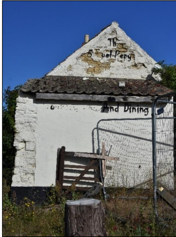
Range 4 abutting Range 3 to the west, looking north-west Fig 12
