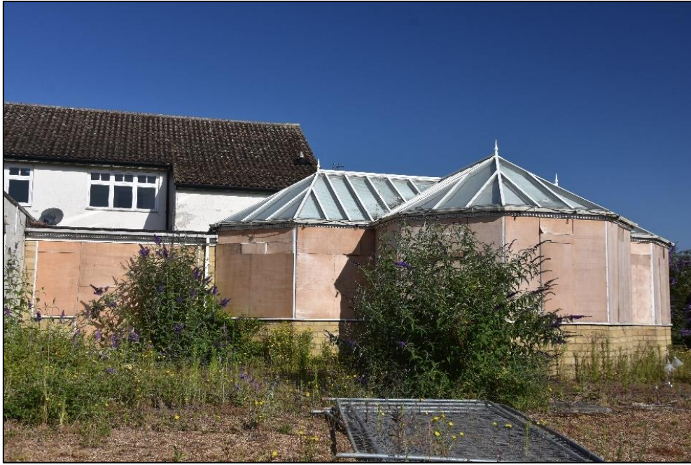
Conservatory range (Range 7), looking north-west Fig 17
