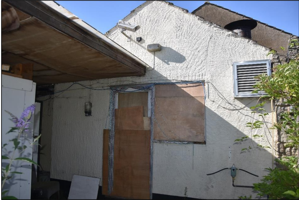
Rendered gable end of Range 8, looking south-west
