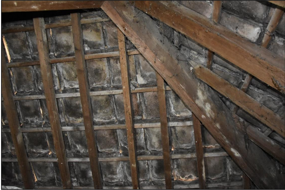
Roof structure above Range 2, looking south Fig 100
