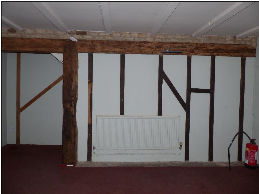
North wall of the lounge with fictive timber-framing, looking north-east Fig 33
