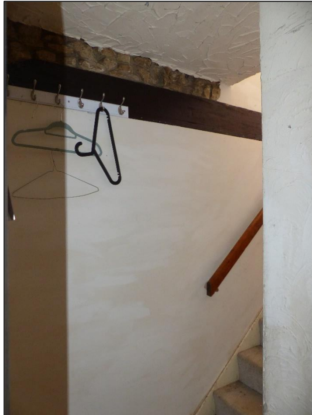
Stone and timber within stair hall (GF06), looking west Fig 44
