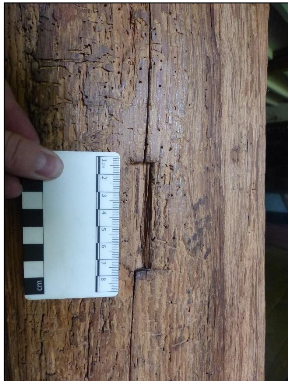
Notches to the post dividing the central and southern bay of the lounge (GF02), looking south-east Fig 30
