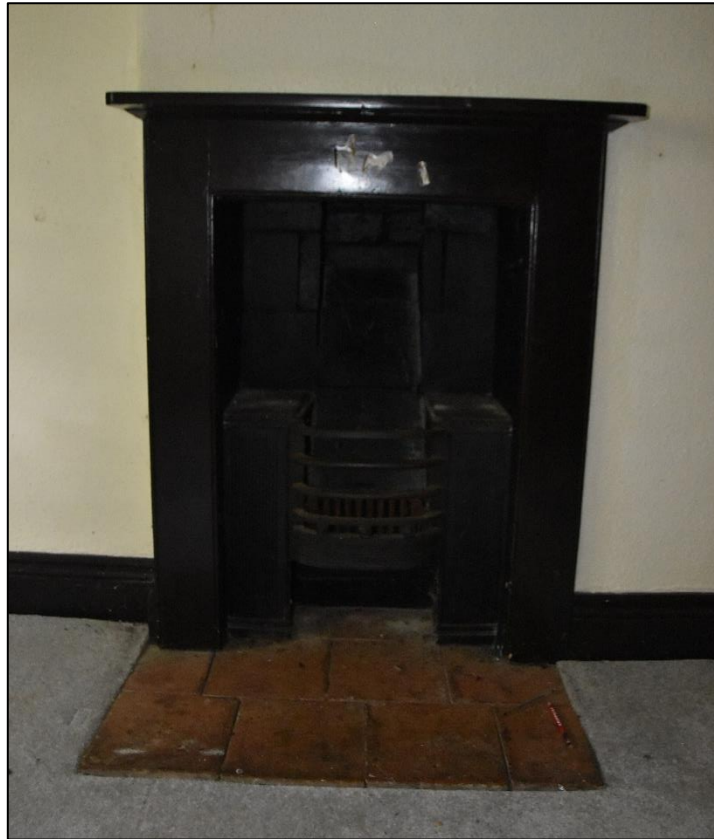
Fireplace in one of the first floor bedrooms (FF05), looking north Fig 82
