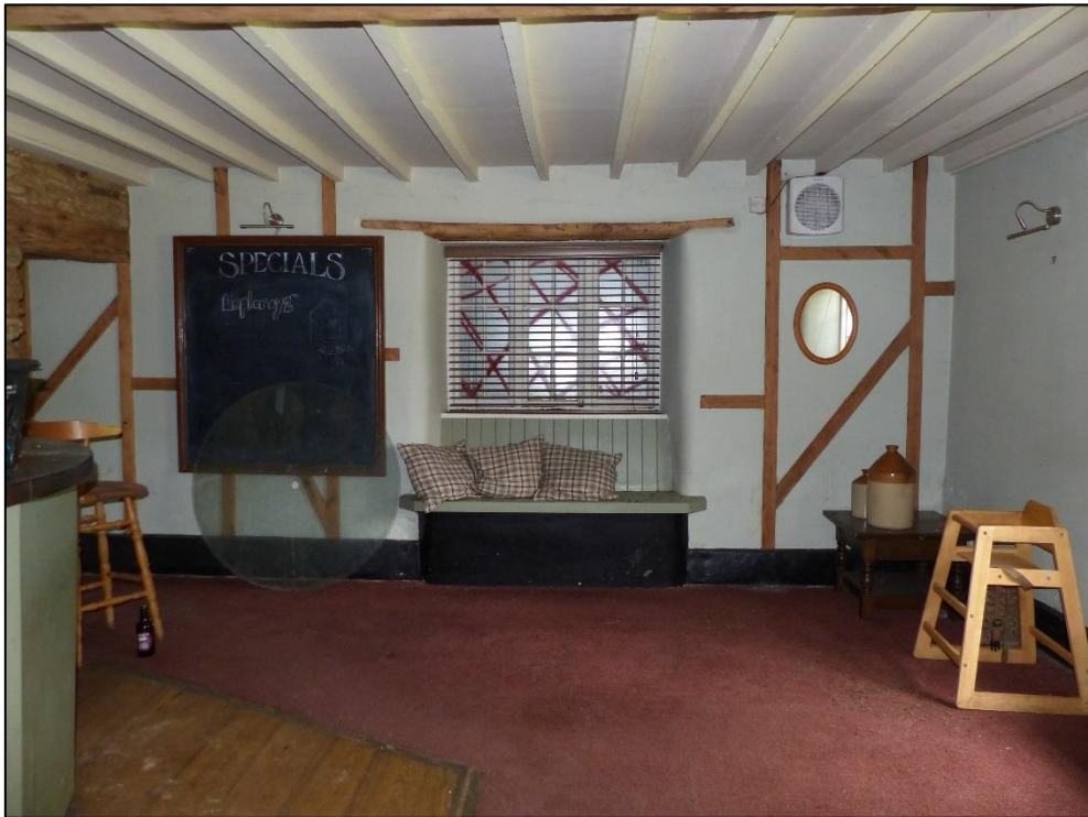
South wall of the lounge (GF02), looking south-west
