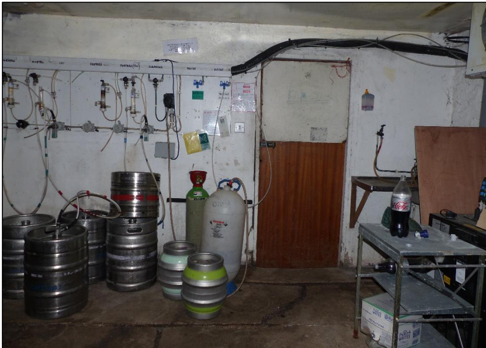
Bar cellar (GF24) interior, looking south-east
