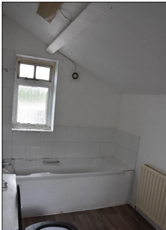
View of the first floor bathroom (FF09a), looking north-east Fig 93
