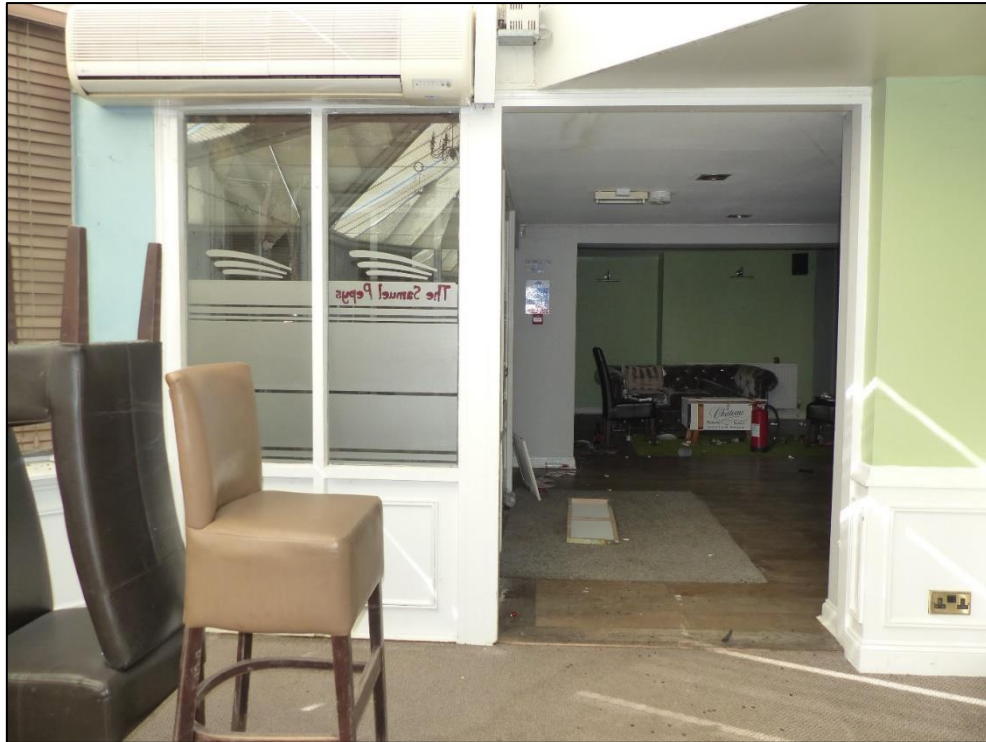
Restaurant looking towards the waiting area (GF04), looking south-west Fig 49
