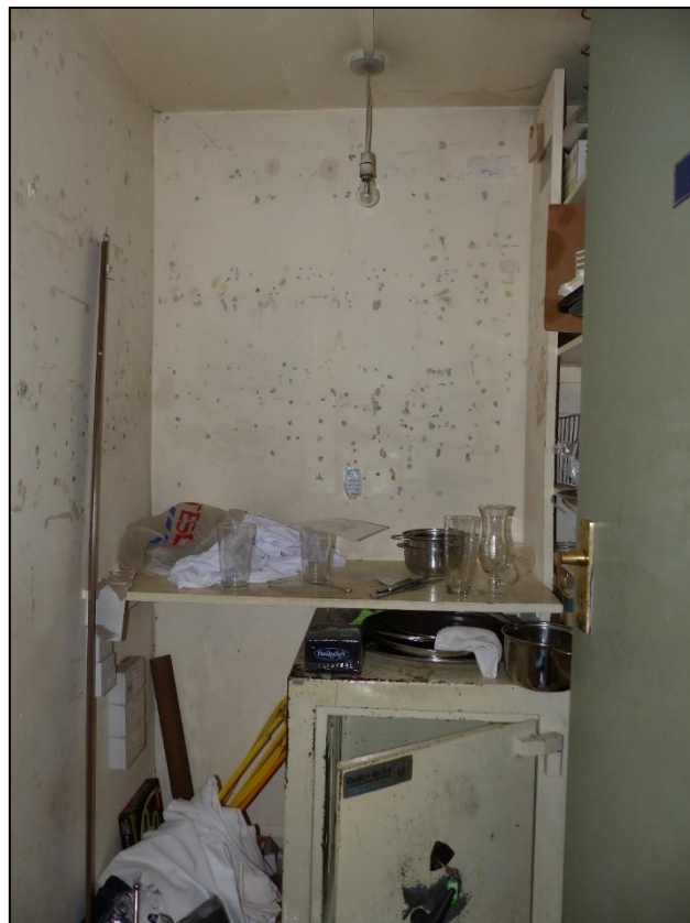
Interior of the safe room (GF05b), looking south-east Fig 41
