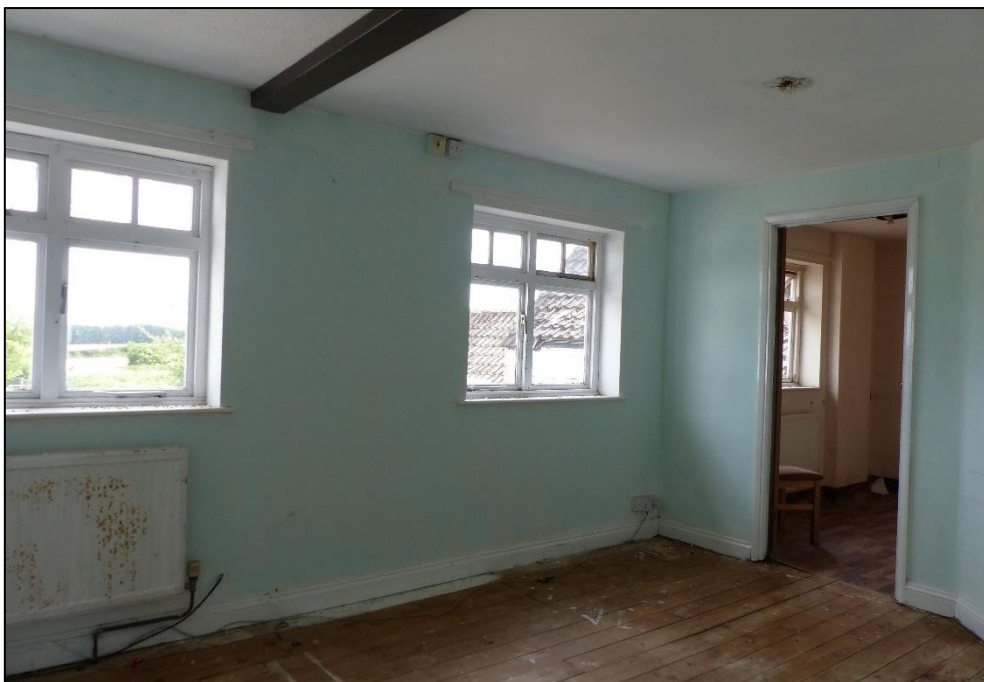
General view of the first floor bedroom (FF10), looking south-east Fig 95
