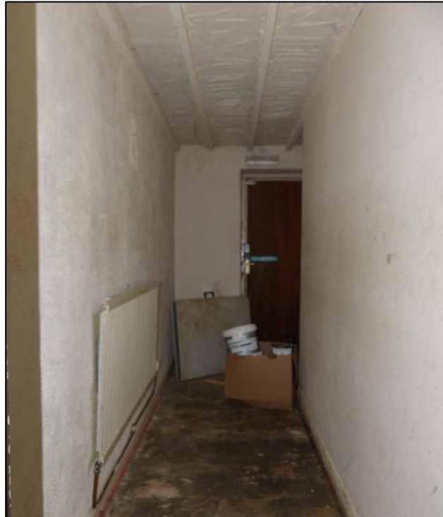
Interior of GF07, looking north-west Fig 45
