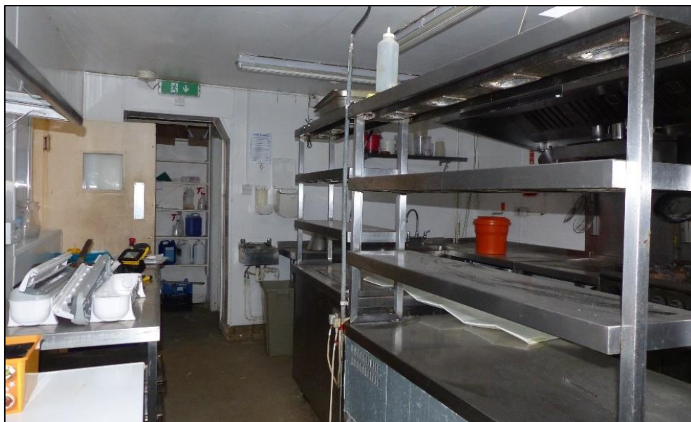
Kitchen (GF10) within Range 8, looking south-west Fig 46
