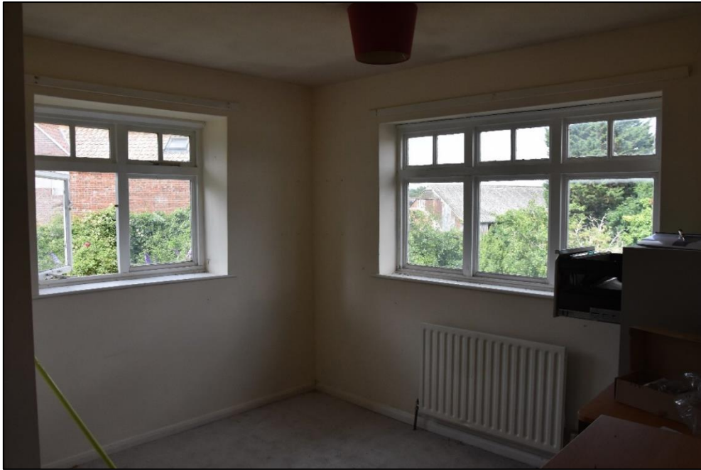
Windows in the first floor office (FF08), looking north-west Fig 89
