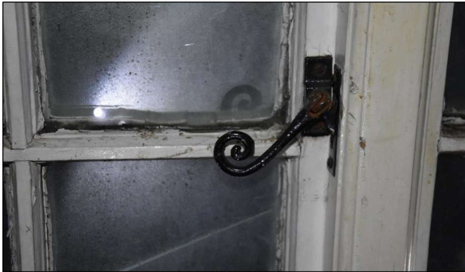
Curled catch and moulded glazing bar to the window in FF03, looking south Fig 74
