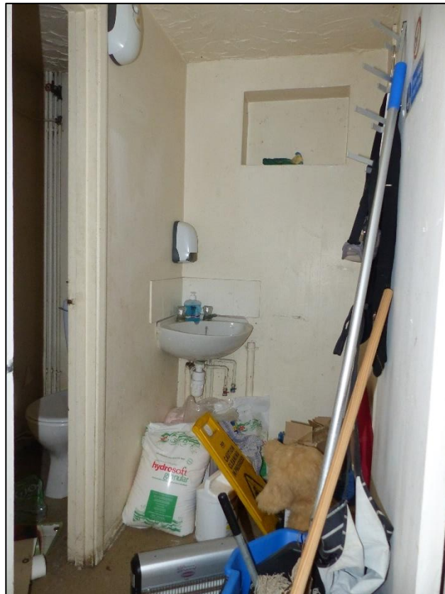
Staff WCs (GF13-13a), looking south-east Fig 43
