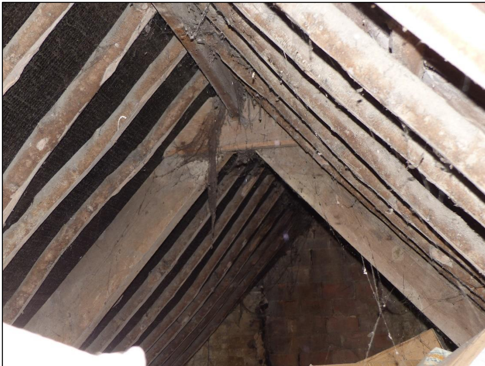
View of the single truss and east gable end within the roof space above Range 1, looking south-east Fig 97
