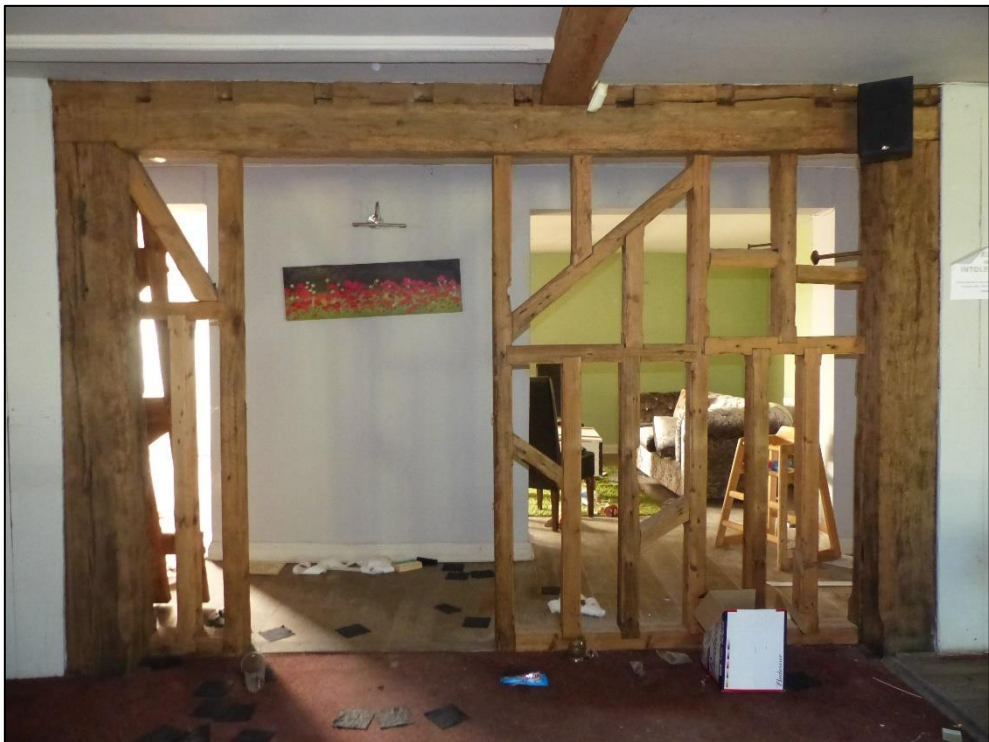
Fictive timber-framing to the east wall of the lounge (GF02), open to the adjoining space (GF05), looking east Fig 35
