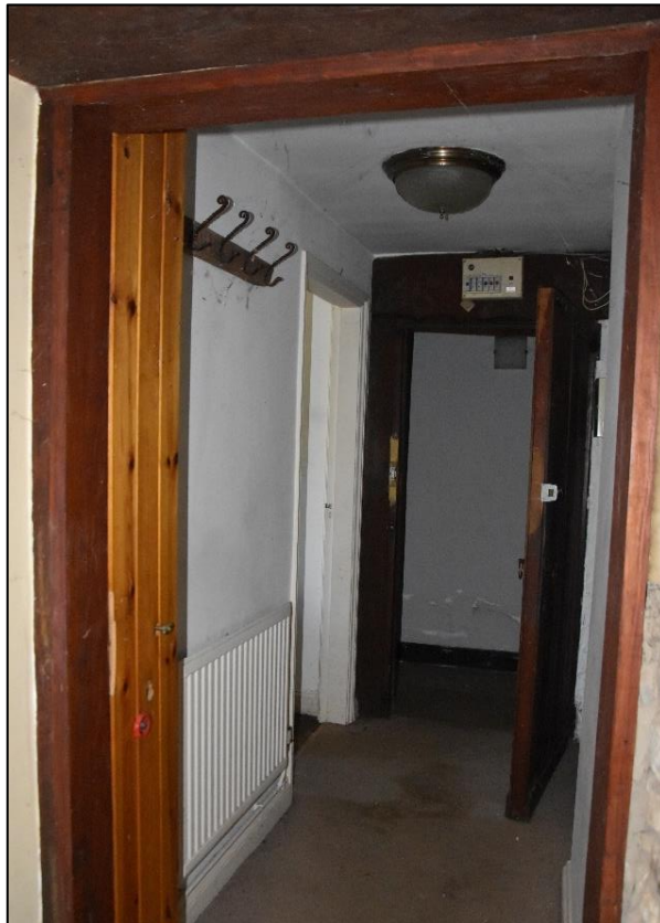
Entrance corridor (GF19), looking north-west
