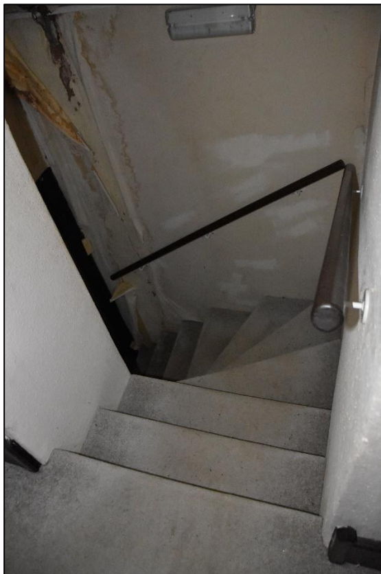
View of the staircase that rises within FF01, looking north Fig 69
