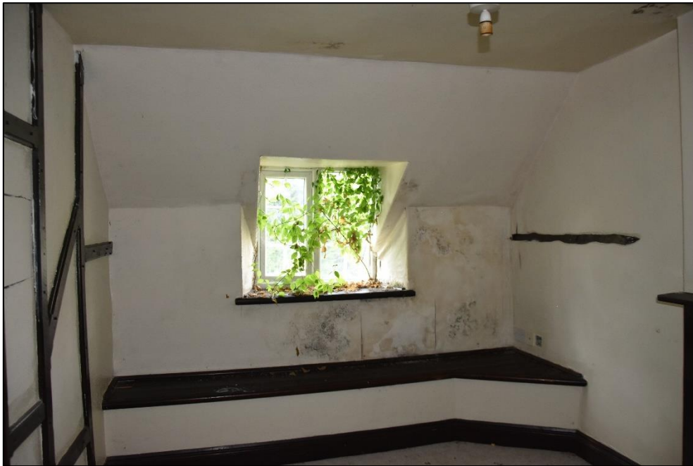
West wall of the first floor bedroom (FF04), looking north-west Fig 81
