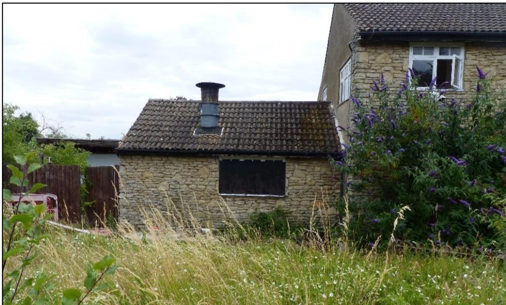
Range 8 abutting Range 5 to the south, looking south-east
