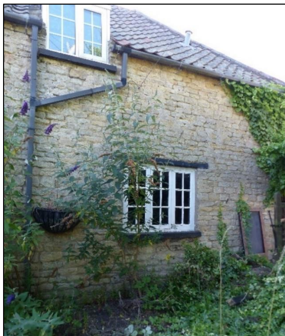
West elevation of Range 2, looking south Fig 9
