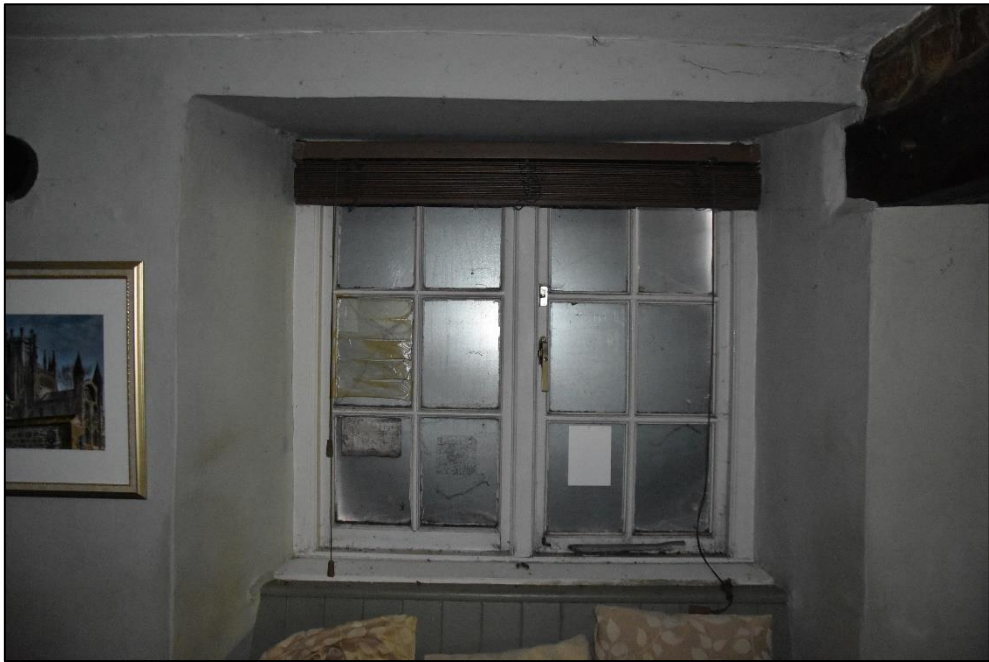
Casement within the bar (GF01), looking south-west
