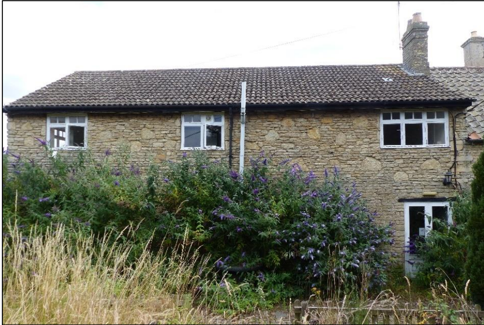
West elevation of Range 5, looking south-east Fig 13
