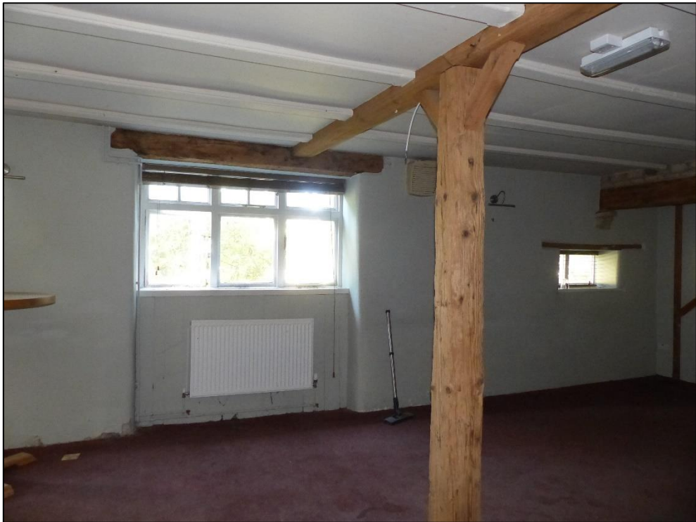
West wall of the lounge (GF02), looking north Fig 32
