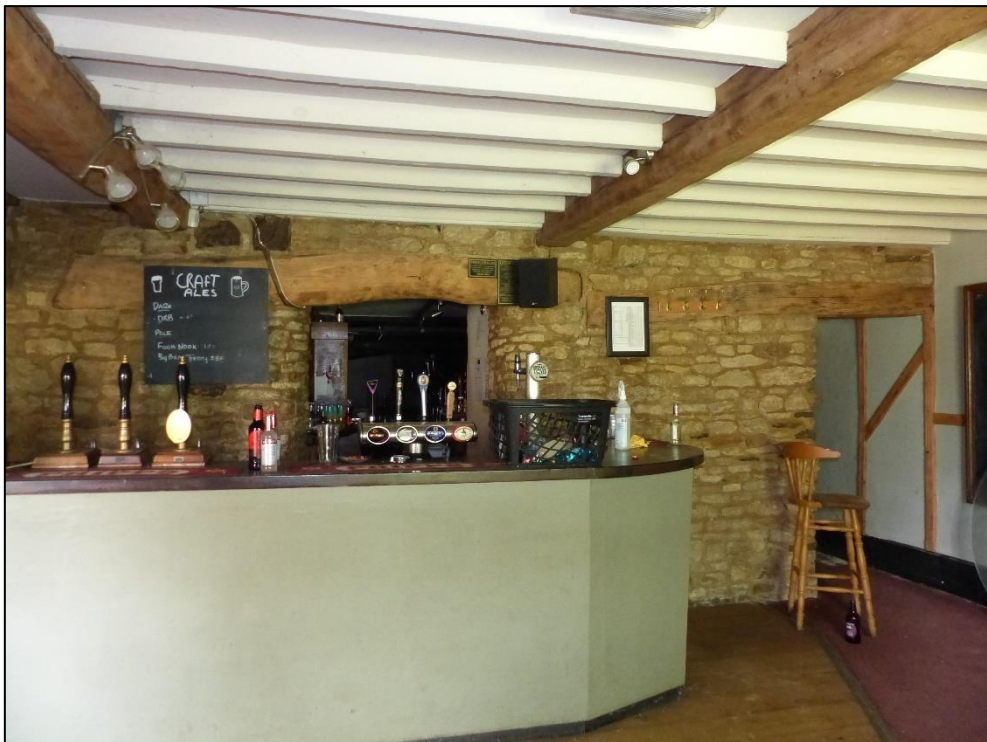
East wall of the southernmost bay in the lounge (GF02), looking south-east
