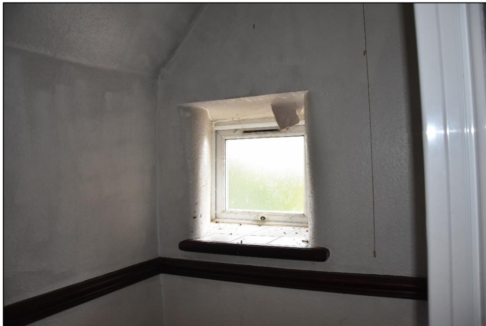
Window to the first floor bathroom (FF02a), looking north-east Fig 73
