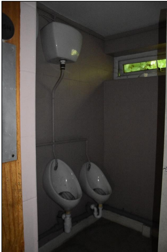
Men's WC (GF18), looking east Fig 55
