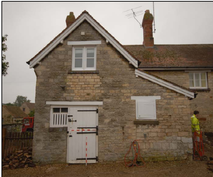
South wing showing stable door and blocked hayloft access
