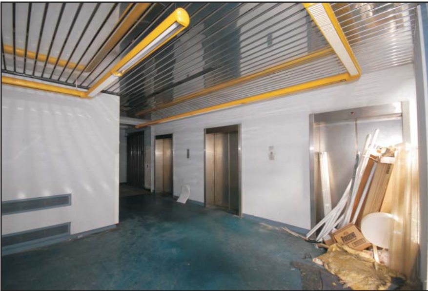
Access Tower, the First Office Level lifts Fig 160
