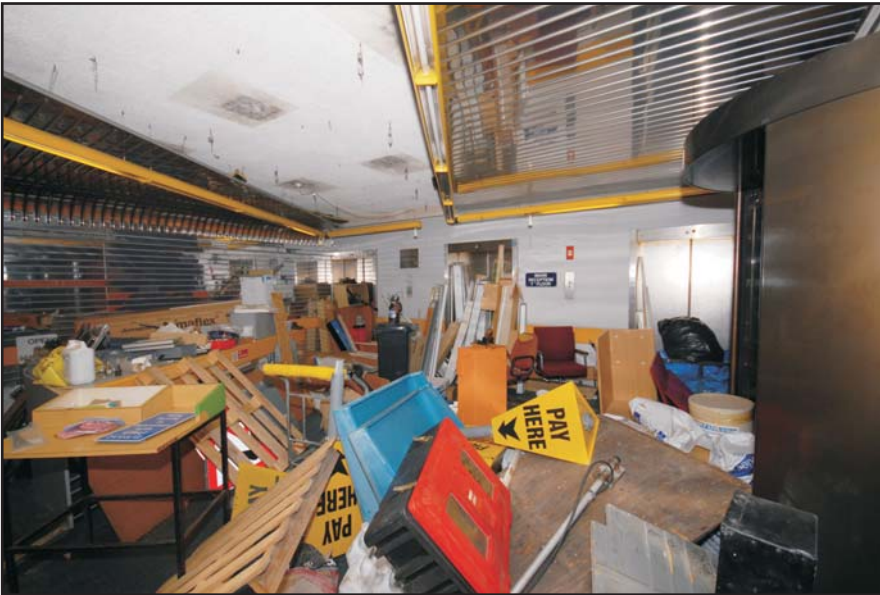
Access Tower, ground level lobby and lifts Fig 152
