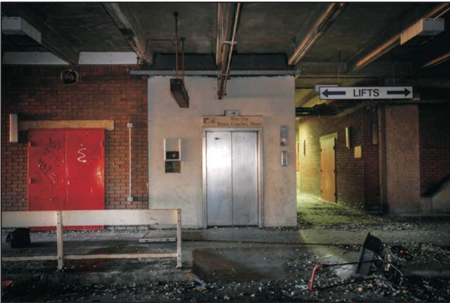
Car Park, the central lift and emergency stairwell, looking west Fig 81
