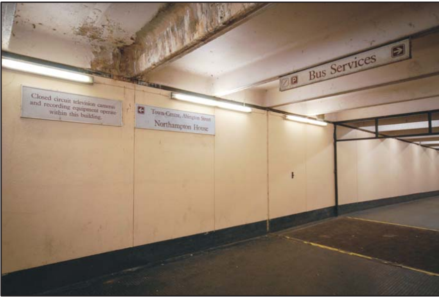
Concourse. detail of signage in the east subway Fig 30
