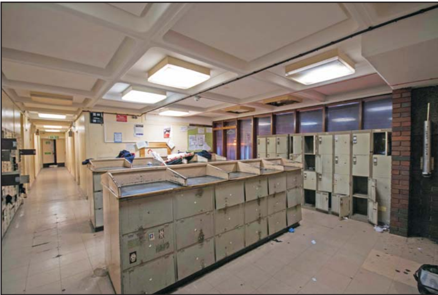
Mezzanine, the staff locker room, looking north Fig 66
