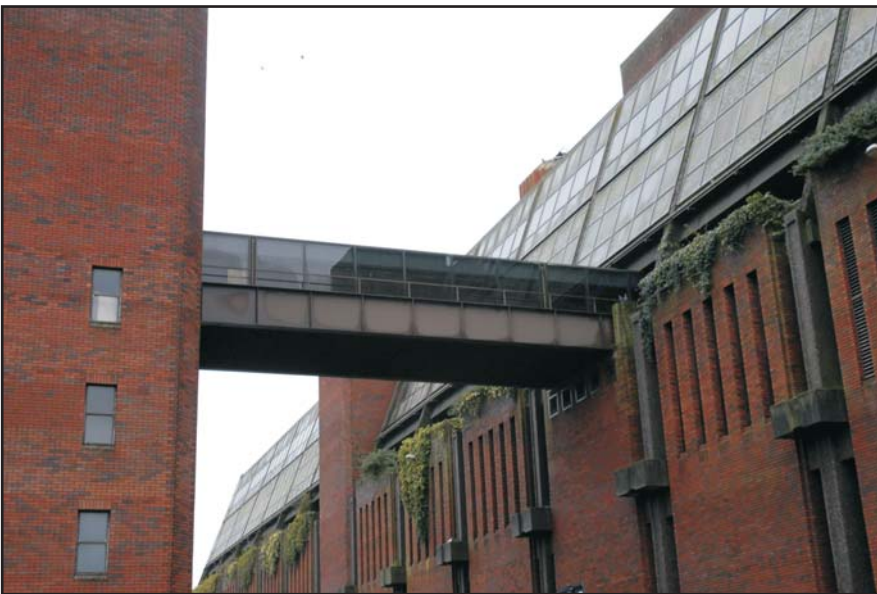
Exterior, the bridge over Lady's Lane, looking east Fig 21
