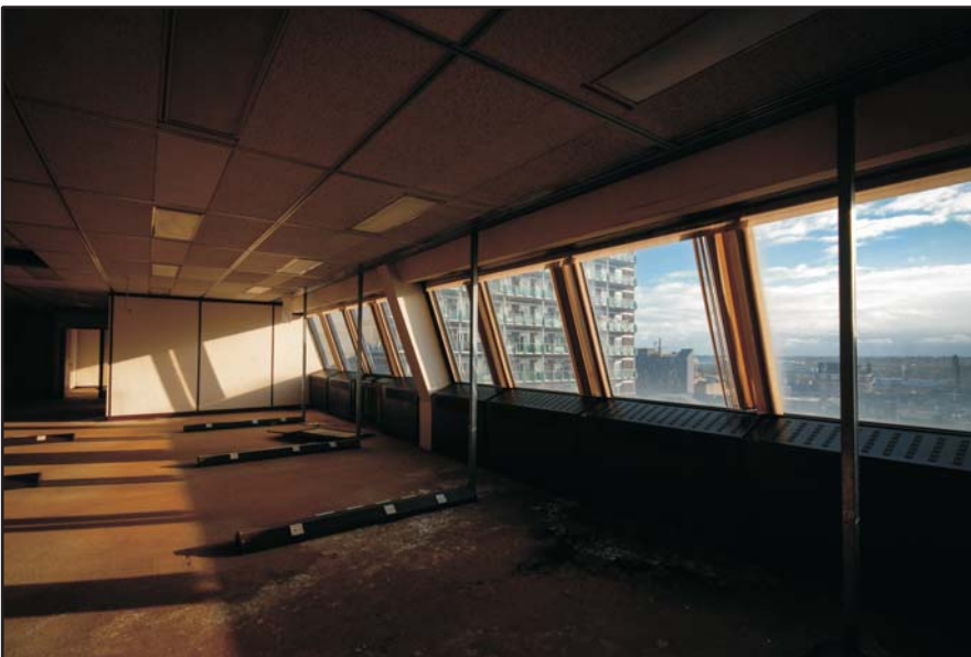
Second Office Level, detail of windows, looking south Fig 112
