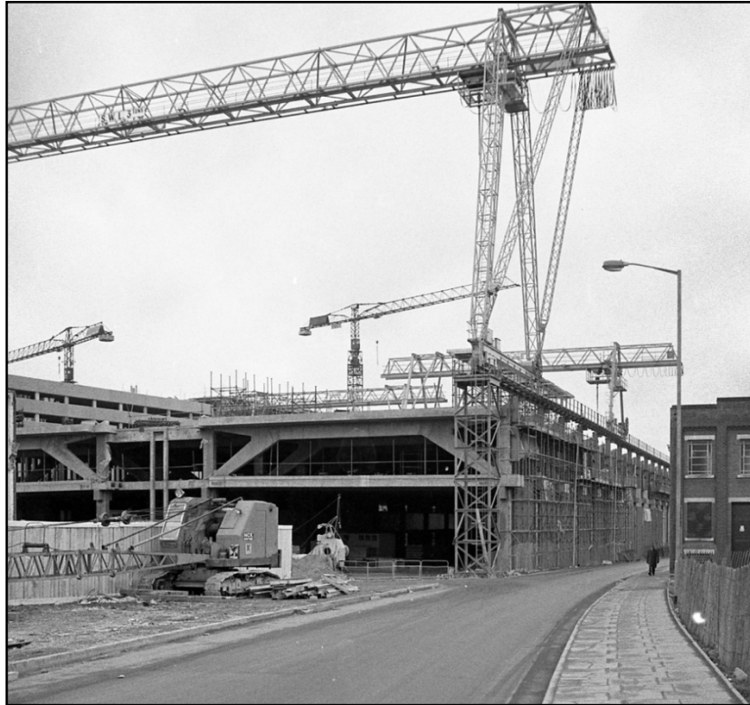
The east elevation and Lady's Lane viewed from the Mounts Fig 10
