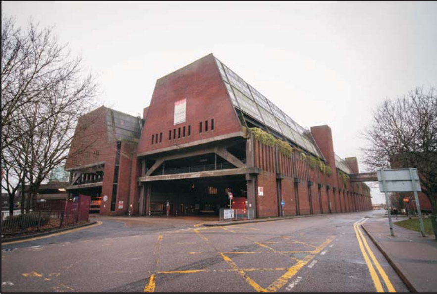
Exterior, the eastern elevation, looking south - west Fig 14
