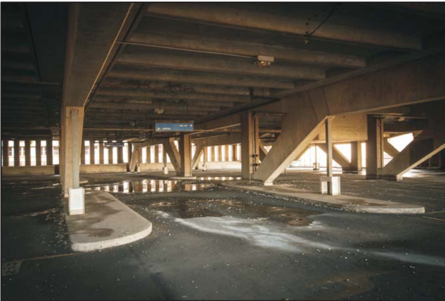
Car Park, general view showing turning kerbs Fig 87
