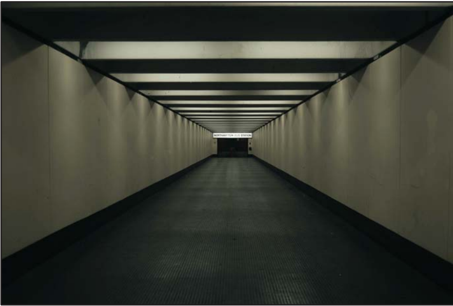
Concourse, the east subway, looking west Fig 31
