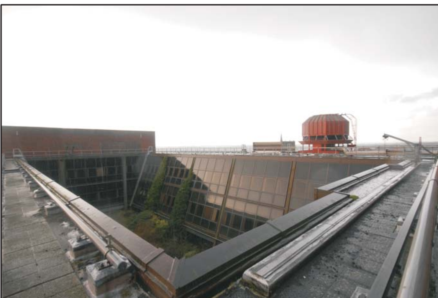
The Roof, the West Atrium, looking north-west Fig 138
