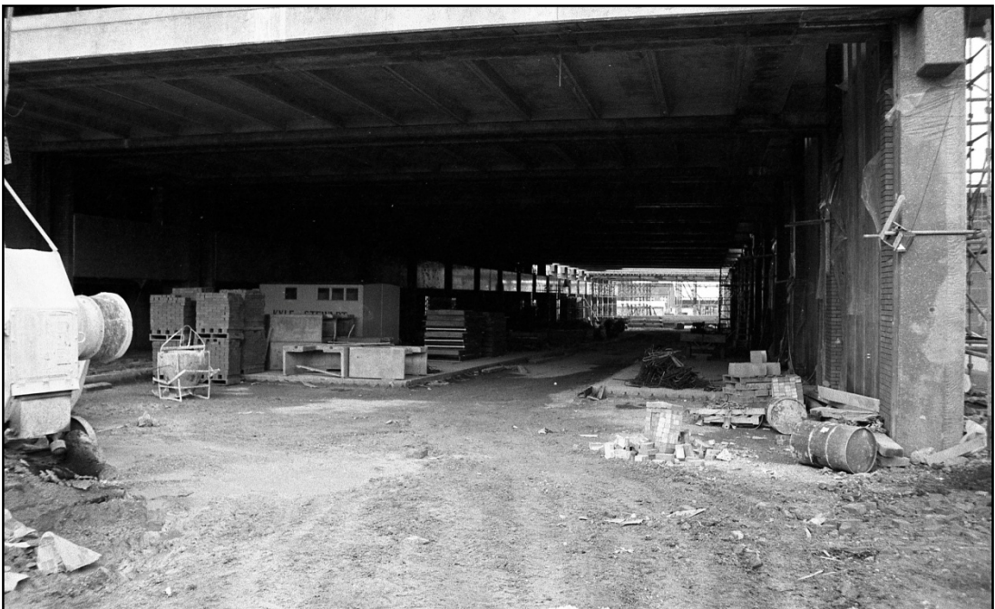
The bus platform under construction, looking west Fig 7
