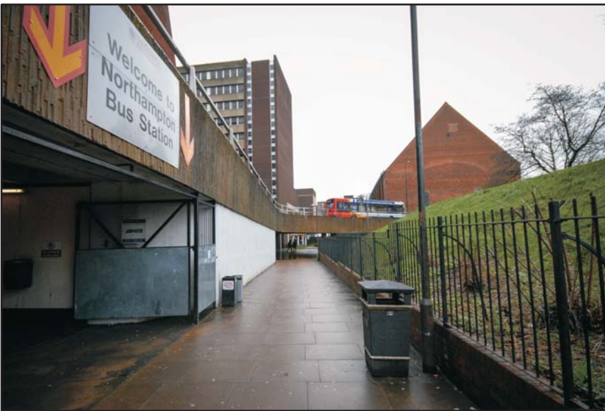
Concourse, the western pedestrian access, looking south Fig 40
