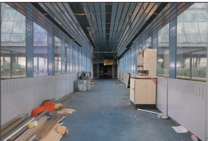
Access Tower, First Office Level, the Bridge, looking south Fig 162
