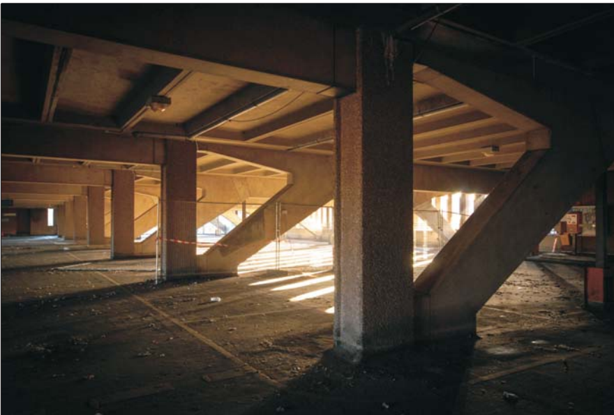
Car Park, detail of the concrete supports Fig 86
