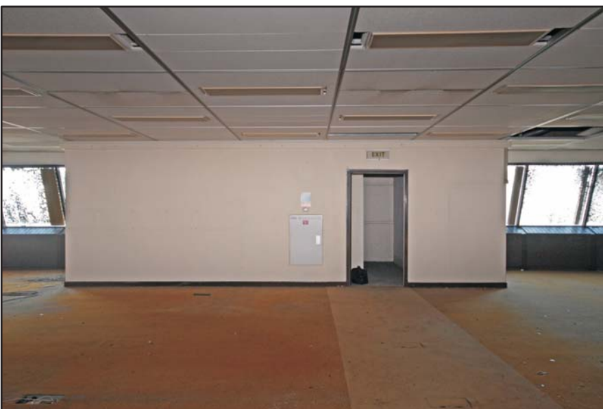
Second Office Level, stairwell to office space Fig 107
