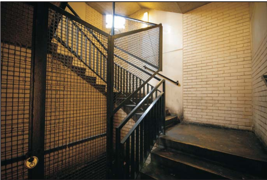
Concourse, stairwell in the east subway Fig 32
