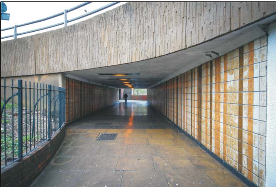
Concourse, the western pedestrian access, looking north Fig 41
