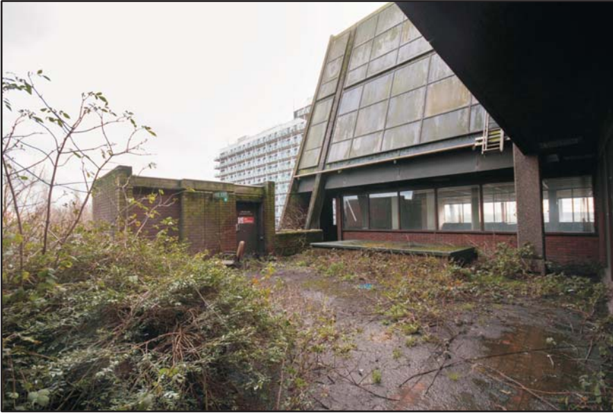
The eastern gable garden, looking south - east Fig 124
