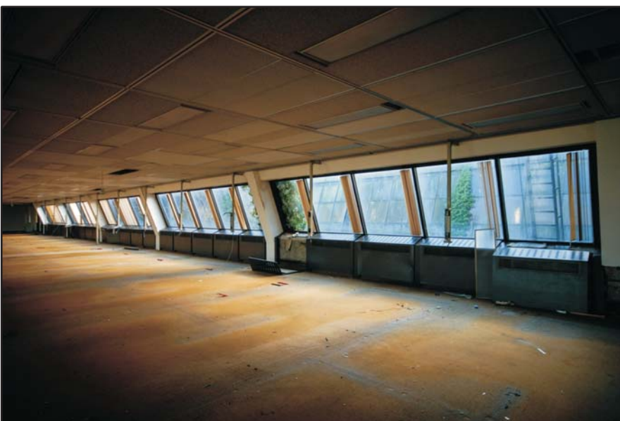
Second Office Level, detail of windows, looking north Fig 113
