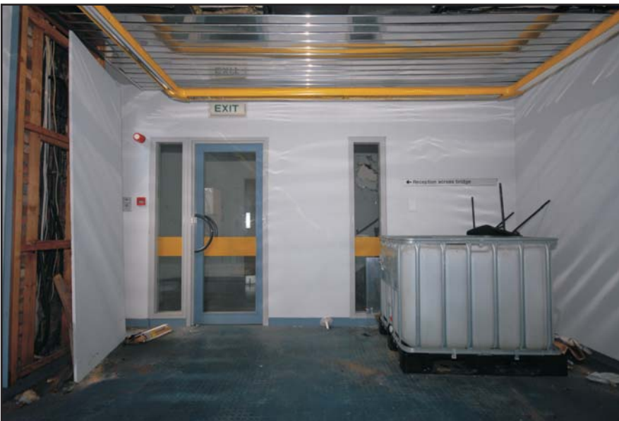
Access Tower, First Office Level stairwell entrance Fig 161
