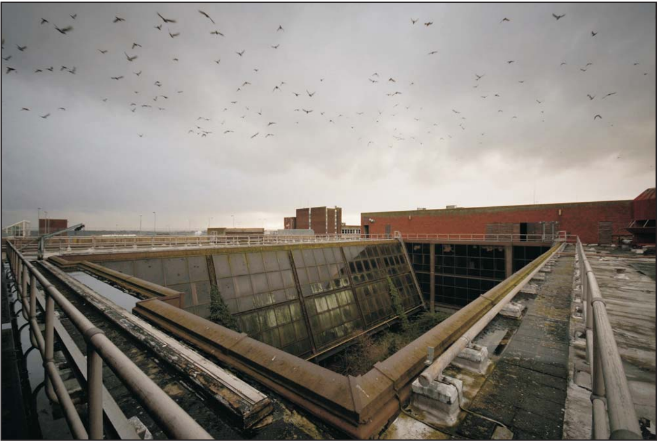
The Roof, the East Atrium, looking south-west Fig 134
