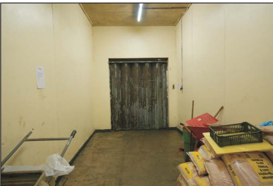
Access Tower, Concourse level goods lift Fig 150
