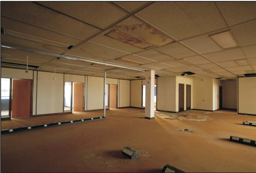
Second Office Level, office partitions, looking east Fig 111
