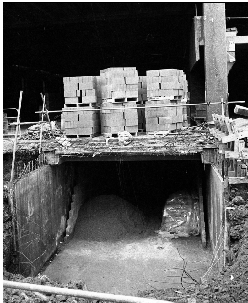
View into the subway through the platform floor Fig 9
