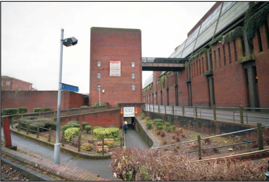
Access Tower, the west elevation, looking east Fig 145
