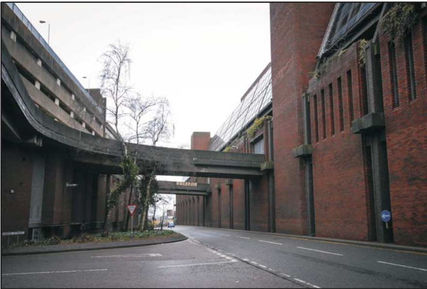
Exterior, the raised bridges over Greyfriars, looking west Fig 17
