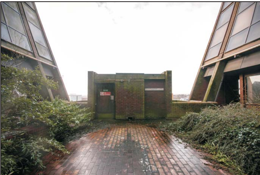
The western gable garden showing the emergency exit, looking west Fig 126
