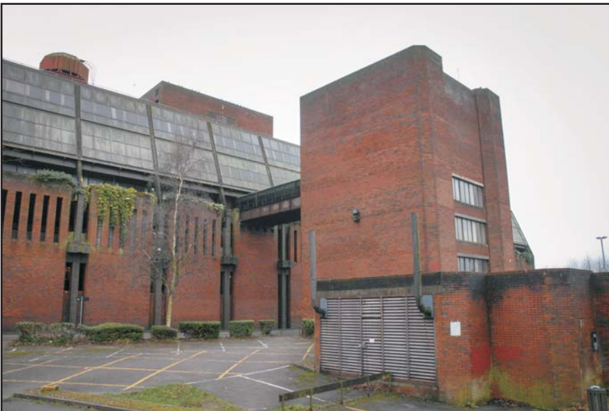
Access Tower, general view, looking south-west Fig 147
