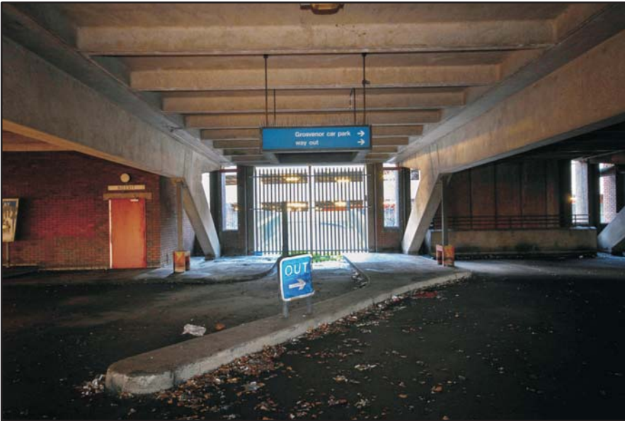
Car Park, entrance to the car park from the Grosvenor ramp, looking south Fig 79
