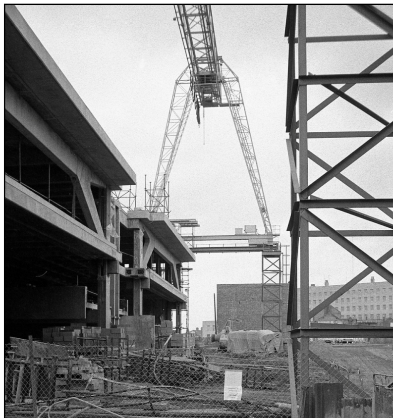
The east elevation under construction, looking north Fig 11
