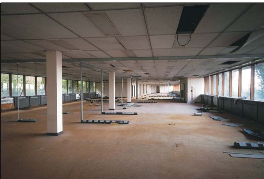
First Office Level, view of the office space, looking west Fig 101
