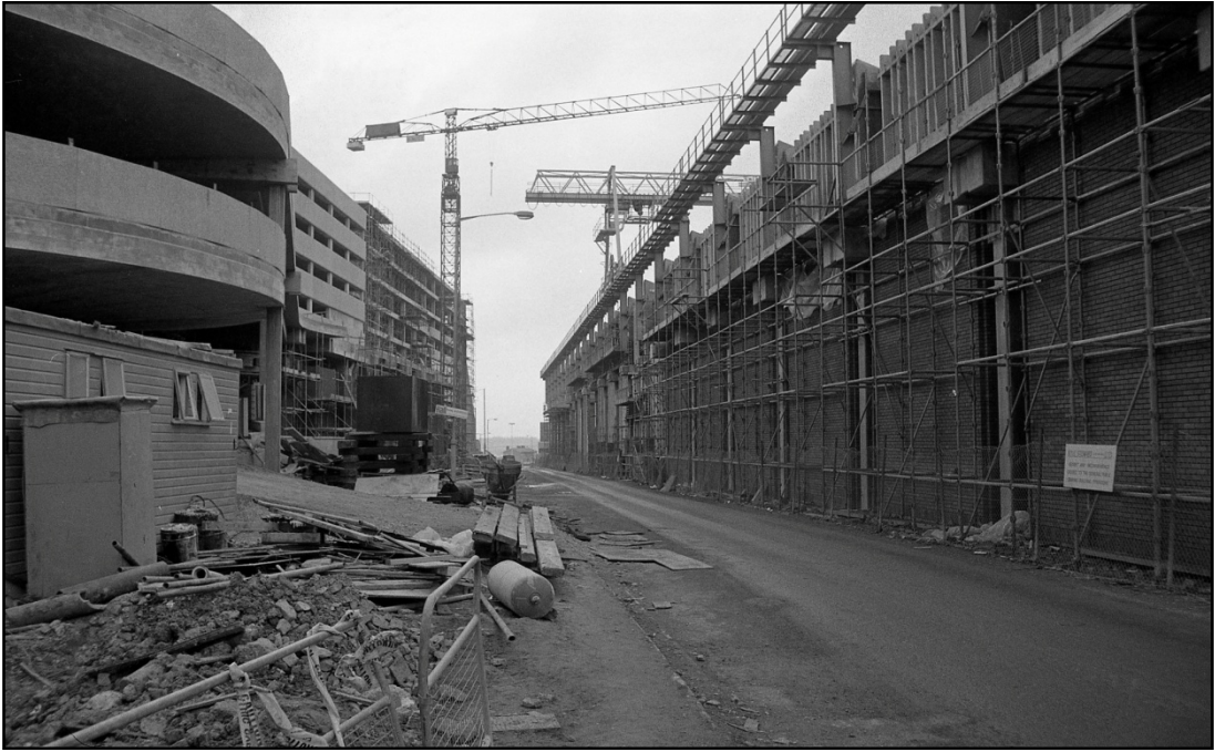
View of the Greyfriars elevation under construction, looking west Fig 8
