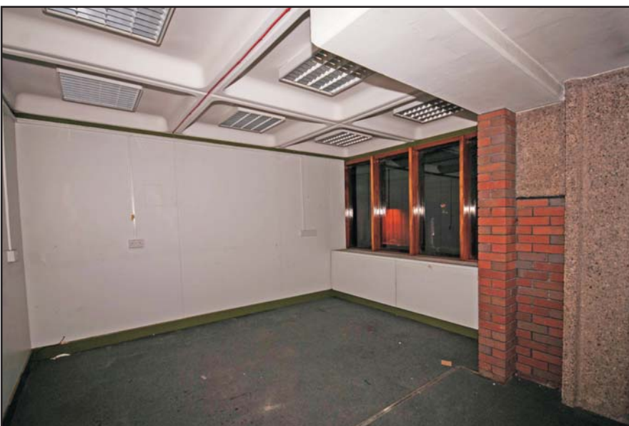
Mezzanine, general view of offices, looking west Fig 71
