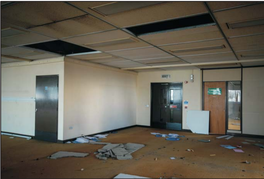
Second Office Level, doors to central access passage and exits Fig 108
