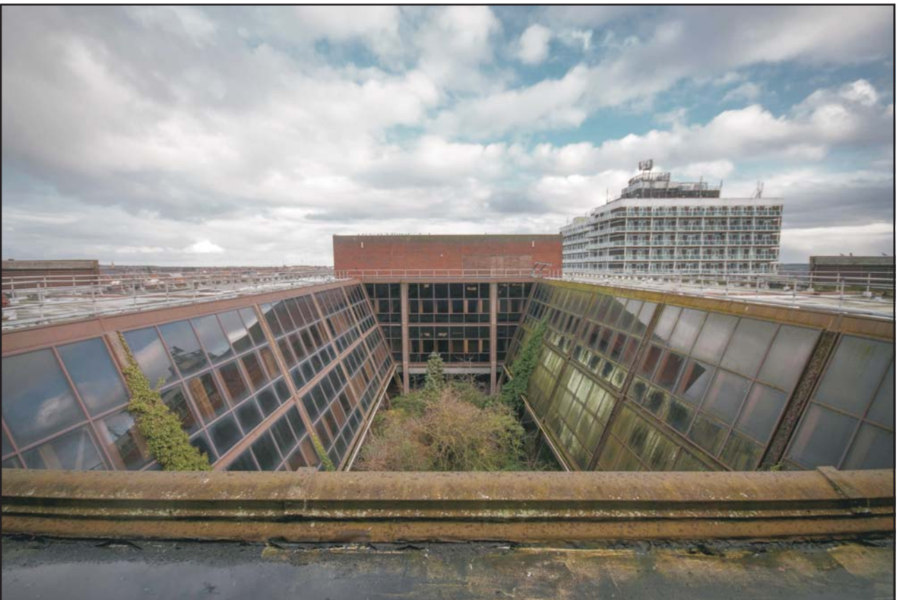
The Roof, the East Atrium, looking east Fig 135
