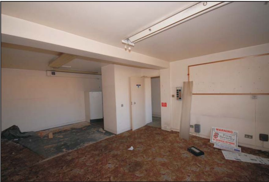
The Flat, the Kitchen and Living Room, looking south Fig 157
