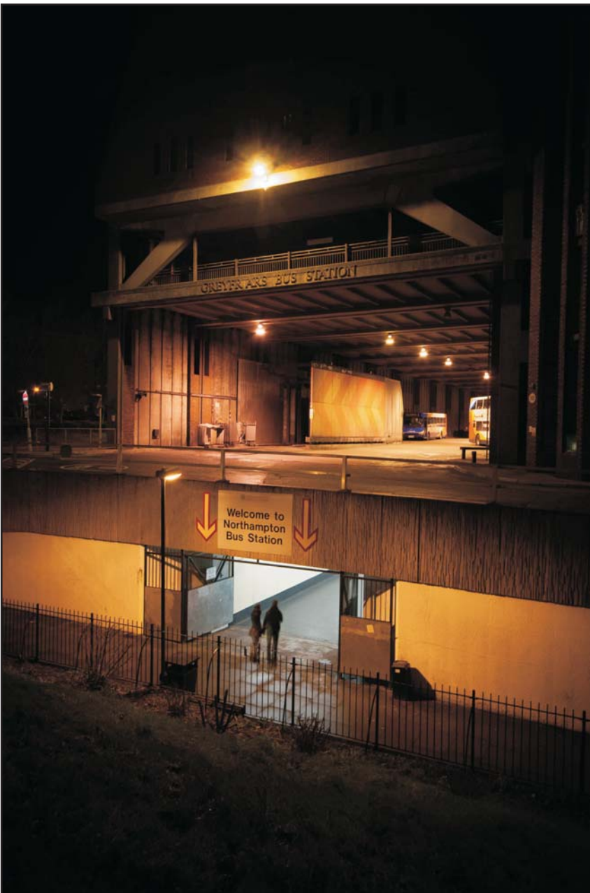
Exterior, the west elevation and subway entrance, night view Fig 24
