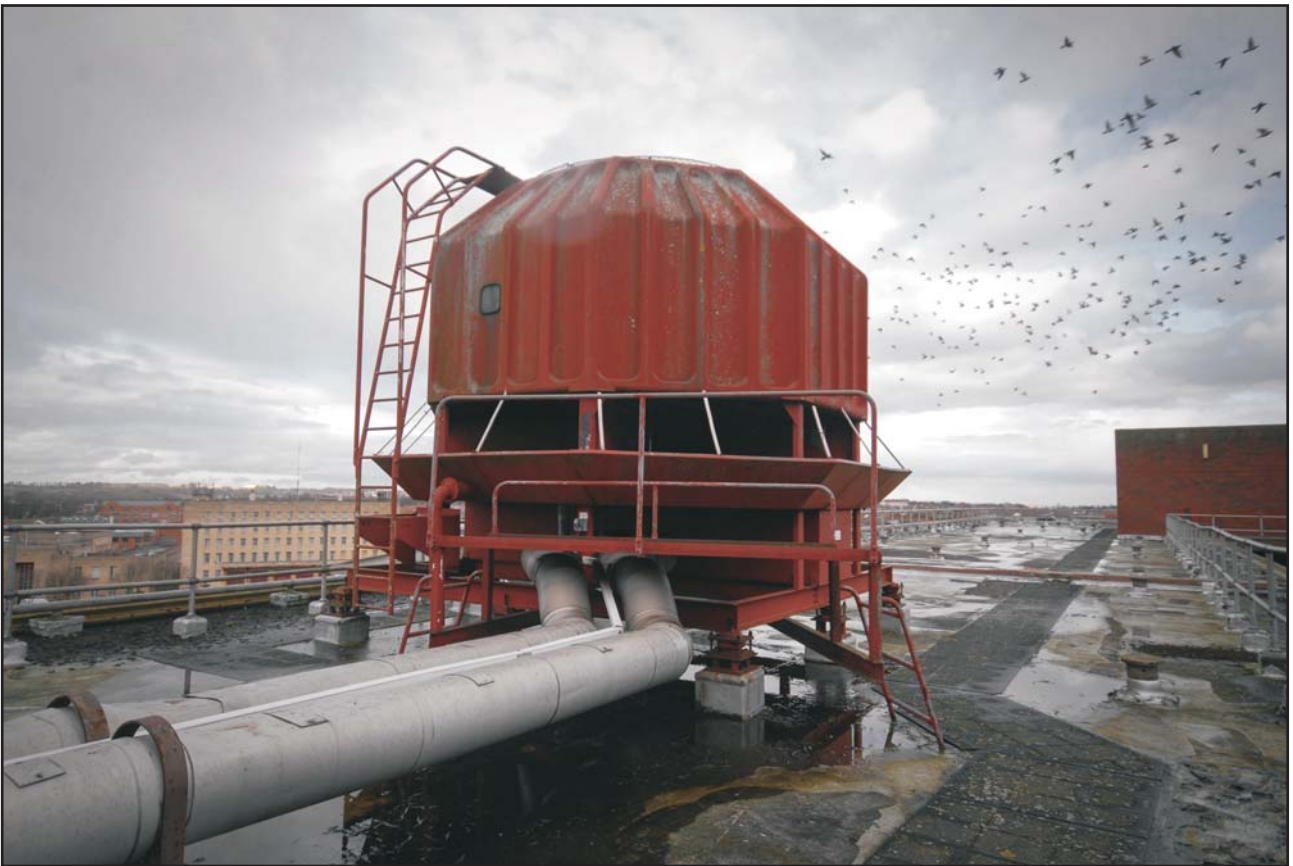
The Roof, the east cooling tower, looking east Fig 140
