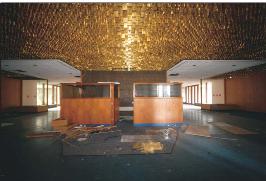
First Office Level, Reception and Lobby, looking south Fig 95
