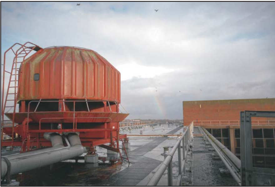
The Roof, general view, looking east, Fig 141
