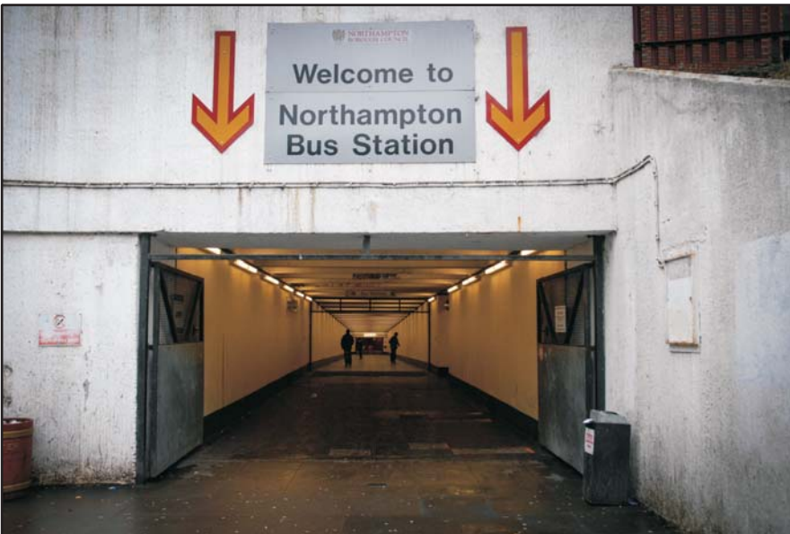
Concourse, view into the east subway Fig 29
