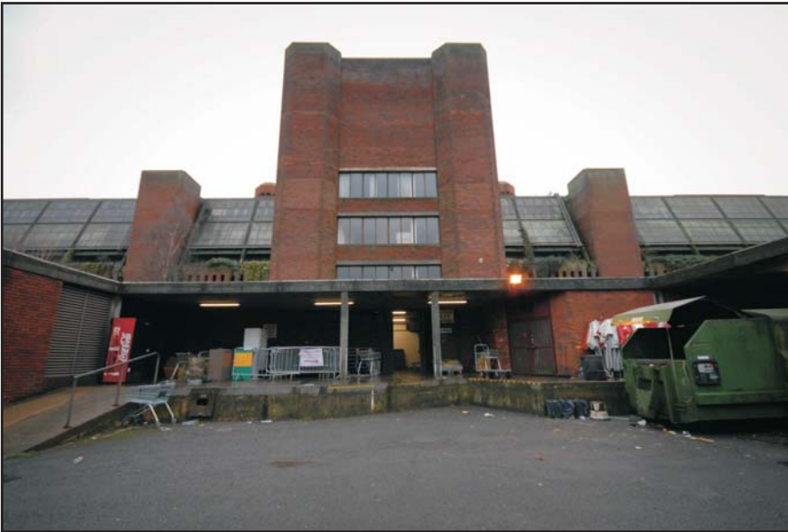
Access Tower, the rear loading bays, looking south Fig 146
