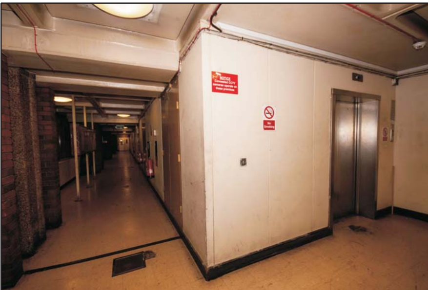
Mezzanine, the central lift and corridor, looking east Fig 64
