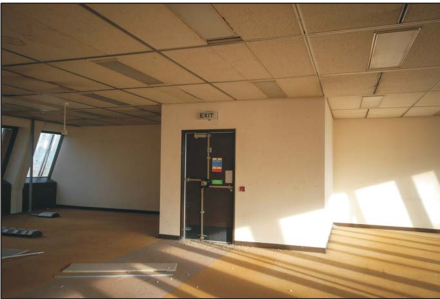
Third Office Level, the east emergency exit Fig 118
