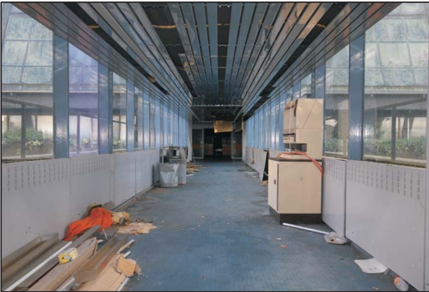
The Bridge, view toward the First Office Level Lobby Fig 93
