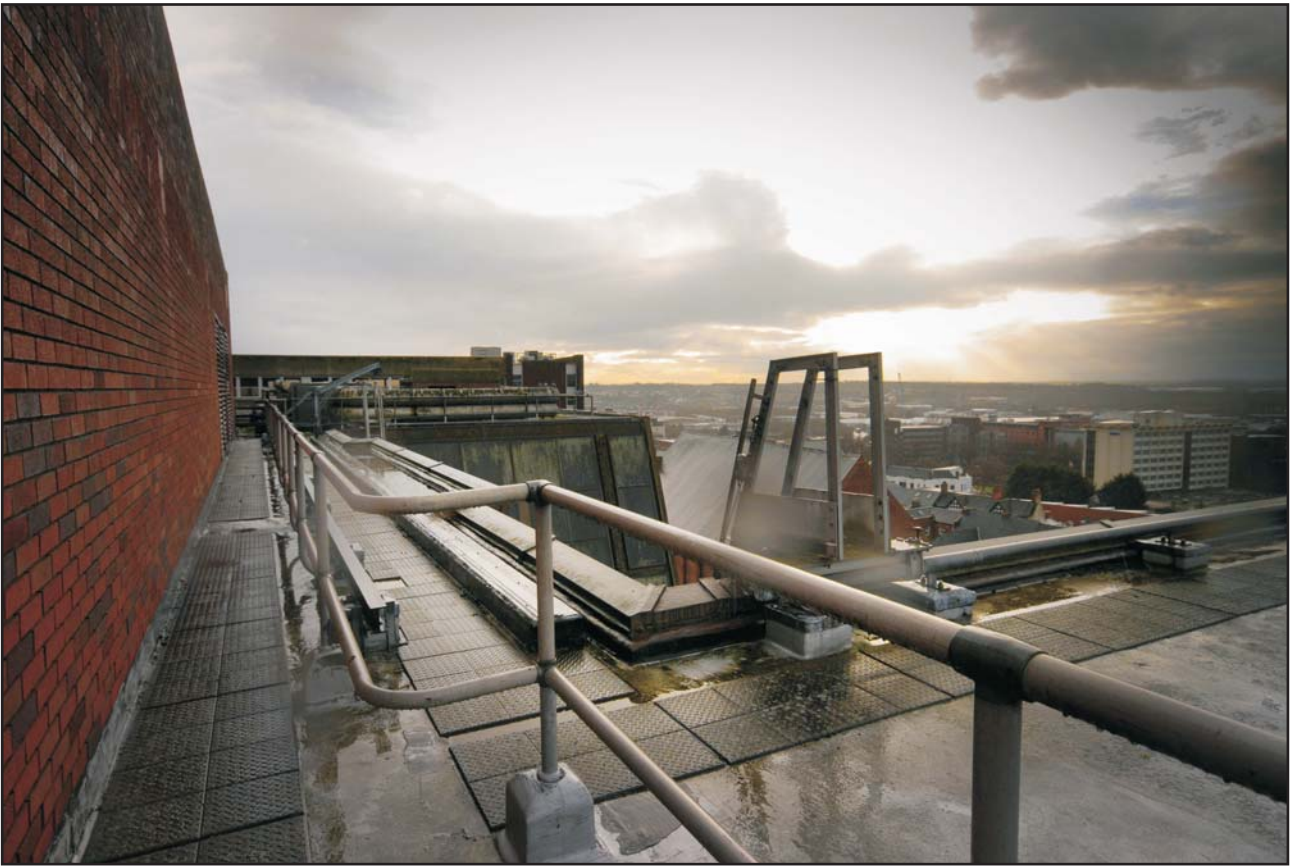
The Roof, the western end of the building, looking south-west Fig 139
