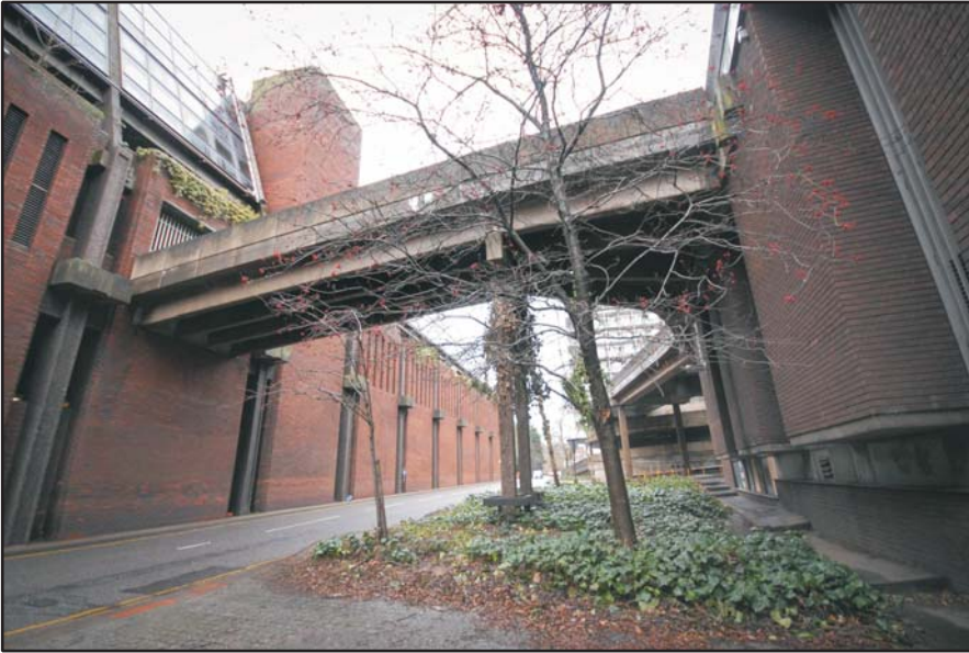
Car Park, the entrance bridge over Greyfriars, looking east Fig 78
