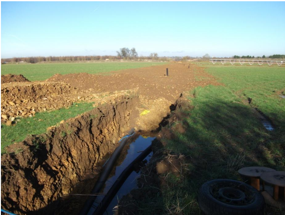
General view of pipe trench at southern end, looking north Fig 2
