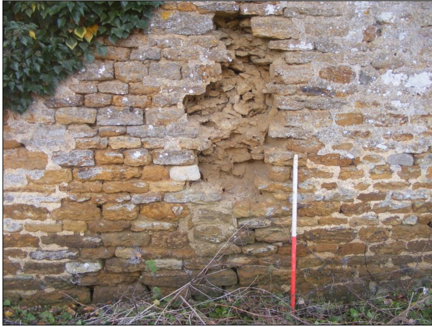
Wall of current barn, looking west
