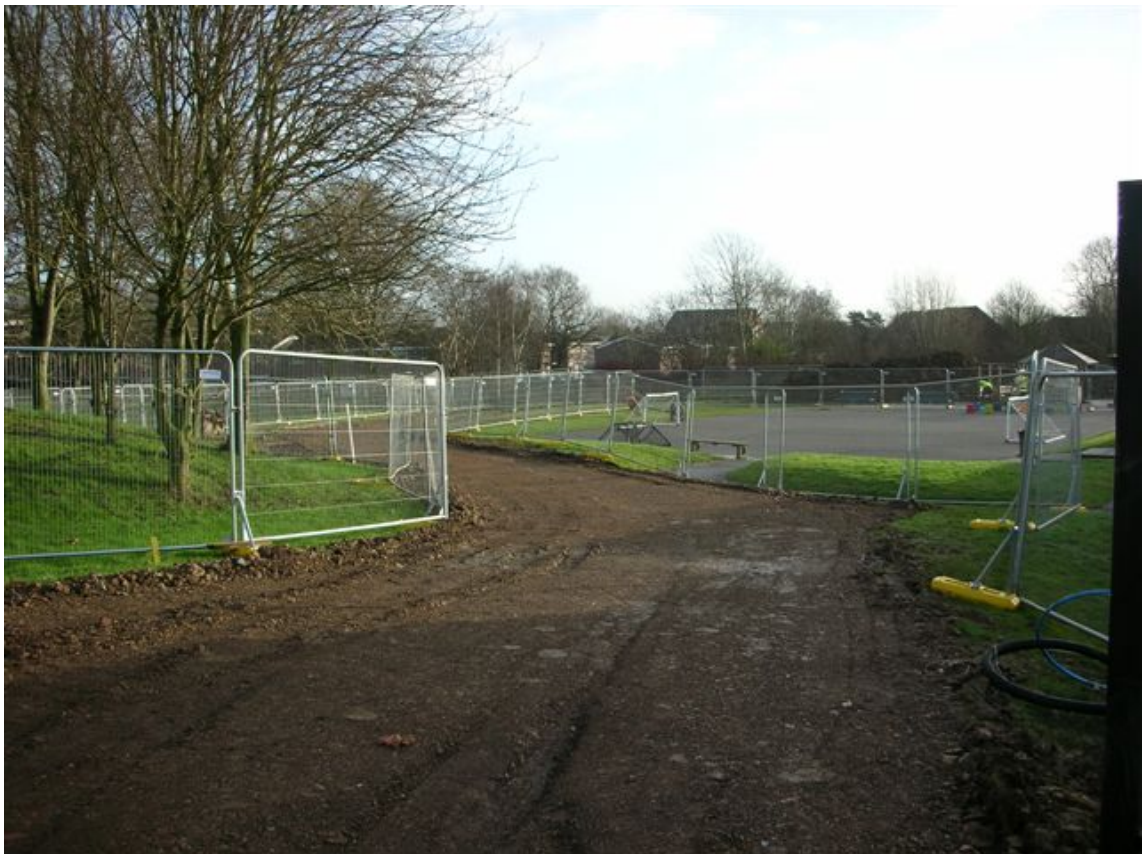
The temporary haul road, looking north-east Fig 4
