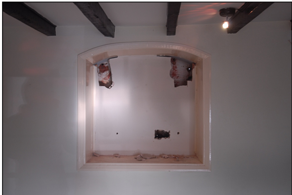
Former window opening in the north wall, level with new doorway Fig 14
