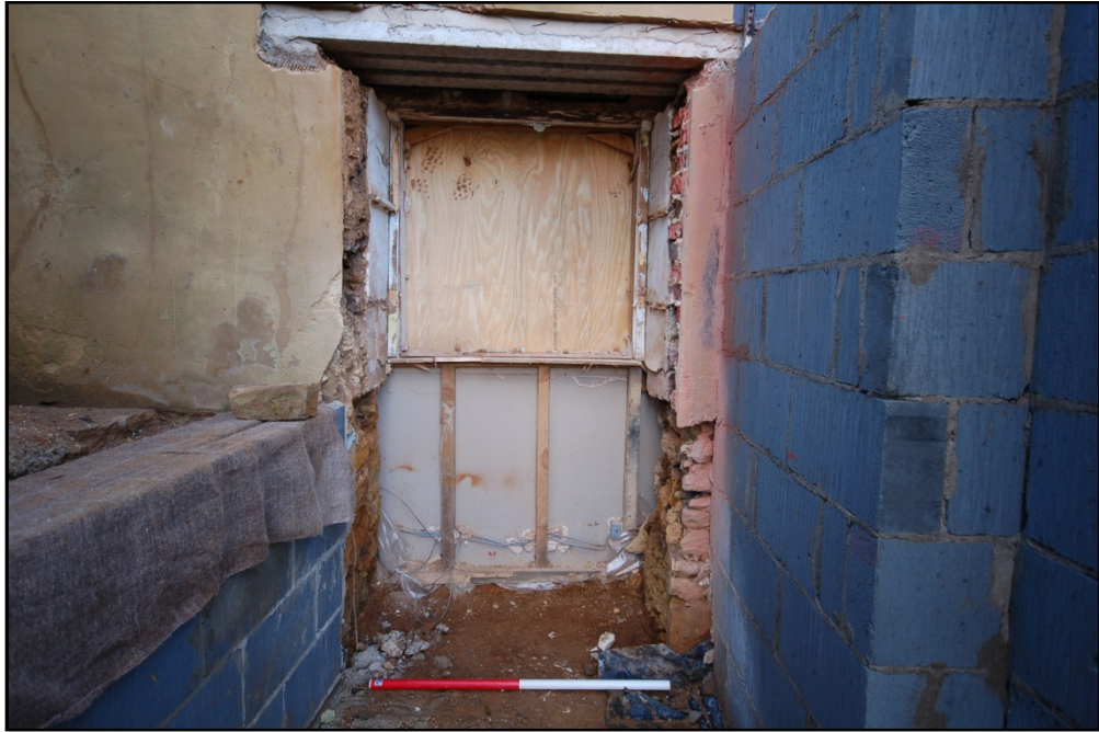
The new doorway after knocking through, looking south Fig 13
