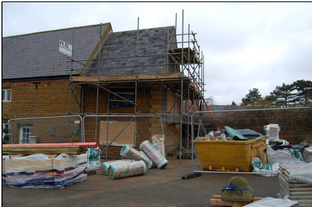
The new extension after completion of groundworks, looking north Fig 18
