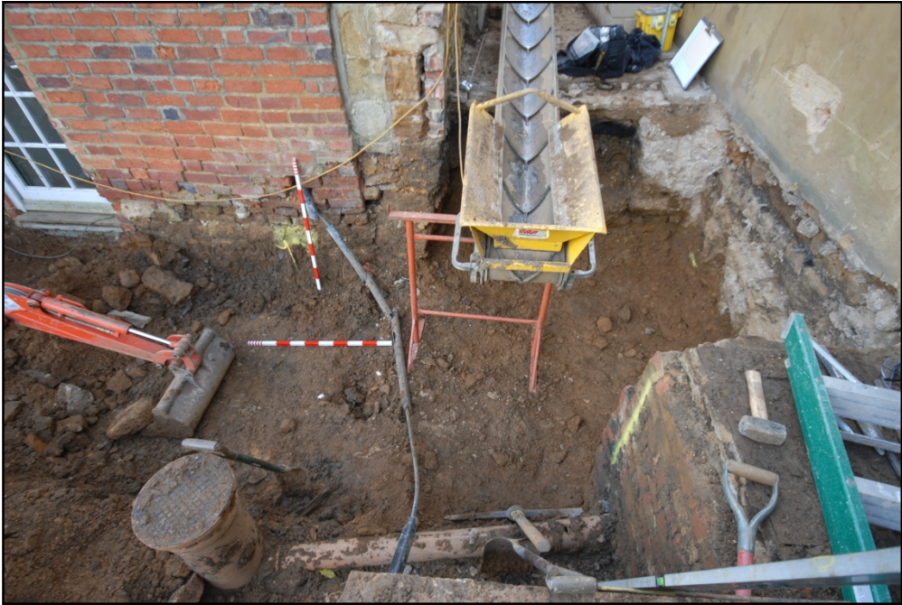
Area 1 during groundworks, looking east Fig 9
