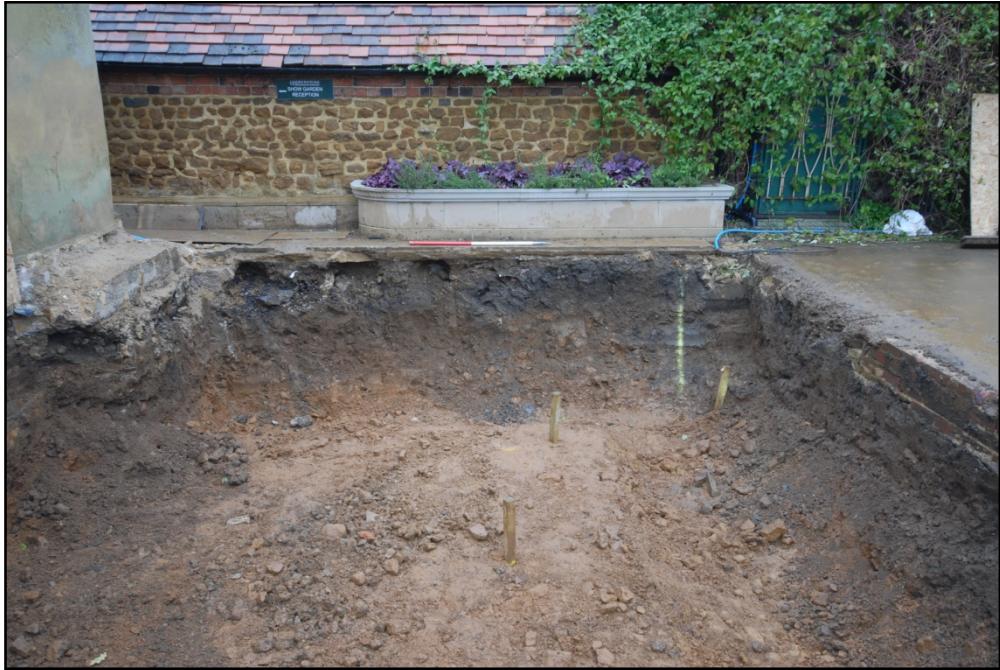
Area 2, during groundworks, looking north Fig 17
