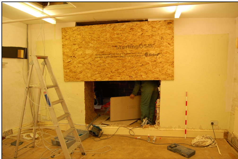
The first floor doorway, looking east Fig 22
