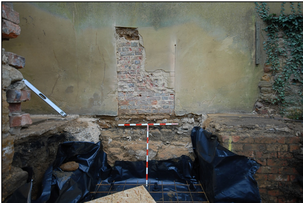
Section 3, new doorway prior to knocking through, looking south Fig 12
