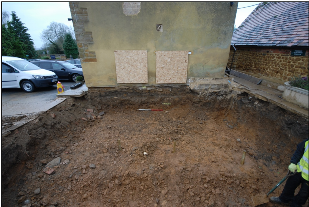
Area 2, during groundworks, looking west Fig 16
