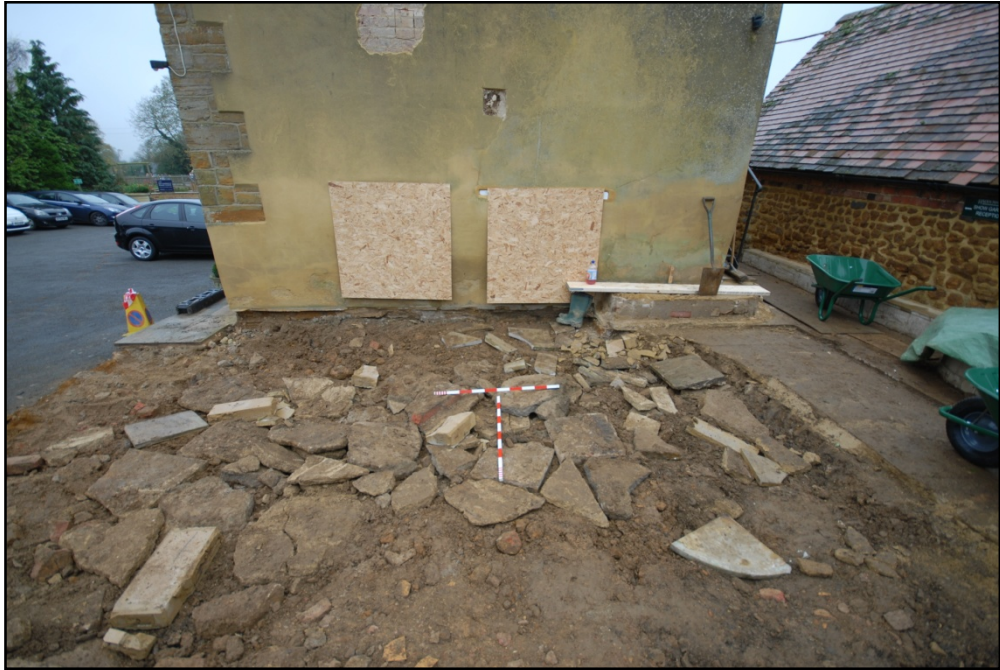
Area 2, general view at the start of groundworks, looking west Fig 15
