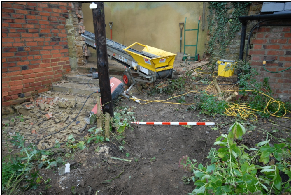
Area 1 at the beginning of groundworks, looking south Fig 8
