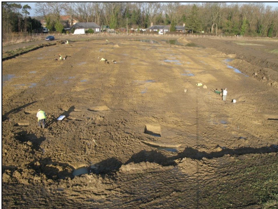
General view of site with work in progress, looking north Fig 3
