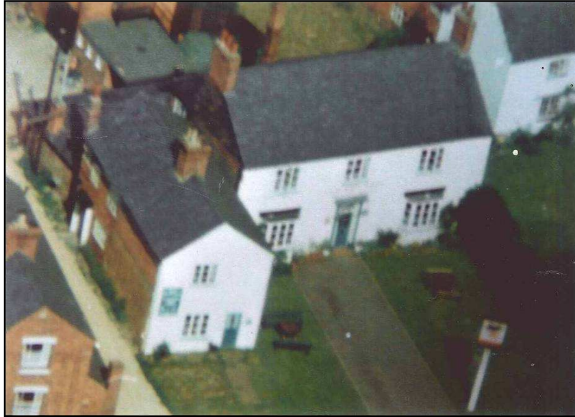
Aerial photo of pub with demolished buildings (possibly 1960s) Fig 5
