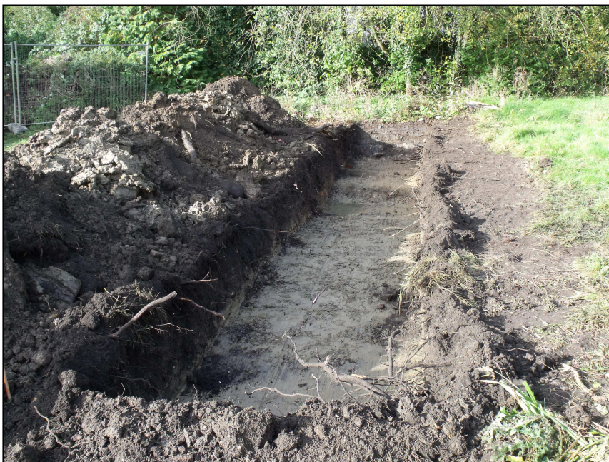
Trench 2, looking south-east Fig 11
