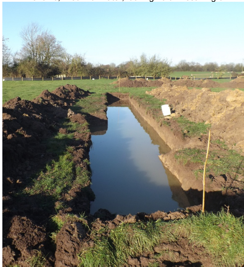
Trench 7, filled with water, looking north-west Fig 7
