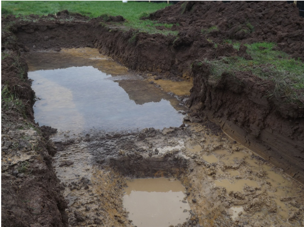
The excavated ditch section Trench 6, looking South Fig 4
