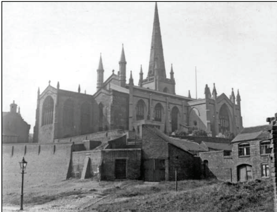
View of the church, looking south-west, showing 19th-century dwellings prior to demolition, photograph dated 1925 (aclickintime.co.uk) Fig 6
