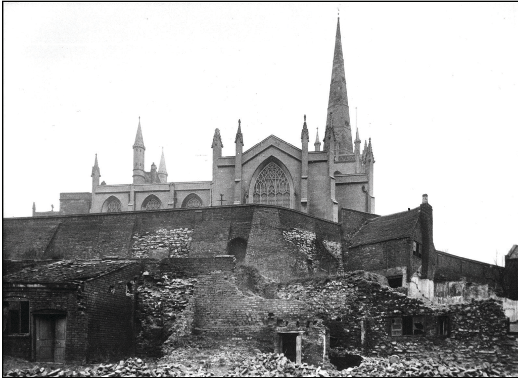
View of the former dwellings during demolition with the retaining wall exposed behind, photograph dated to 1930s (aclickintime.co.uk) Fig 9
