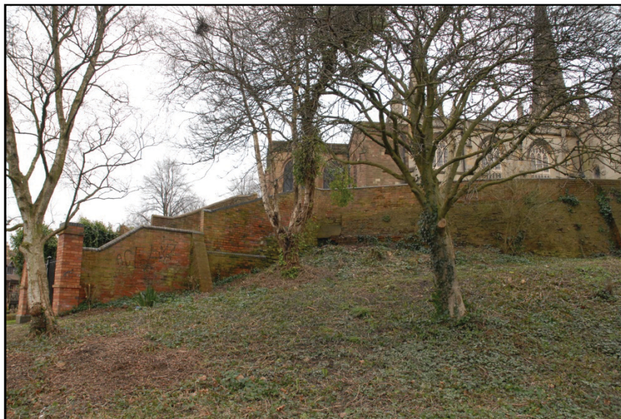
The eastern extent of the retaining wall, looking south-east Fig 16
