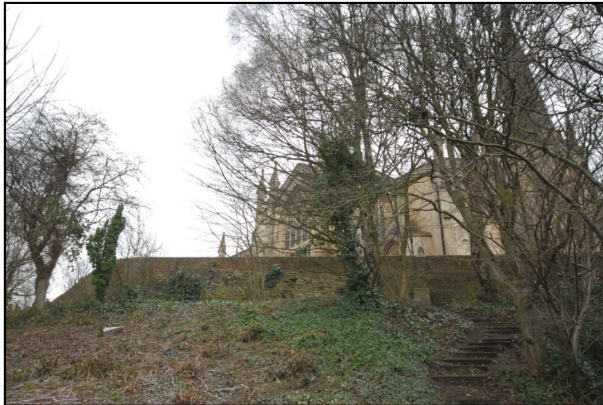
The western extent of the retaining wall, looking south-east Fig 18
