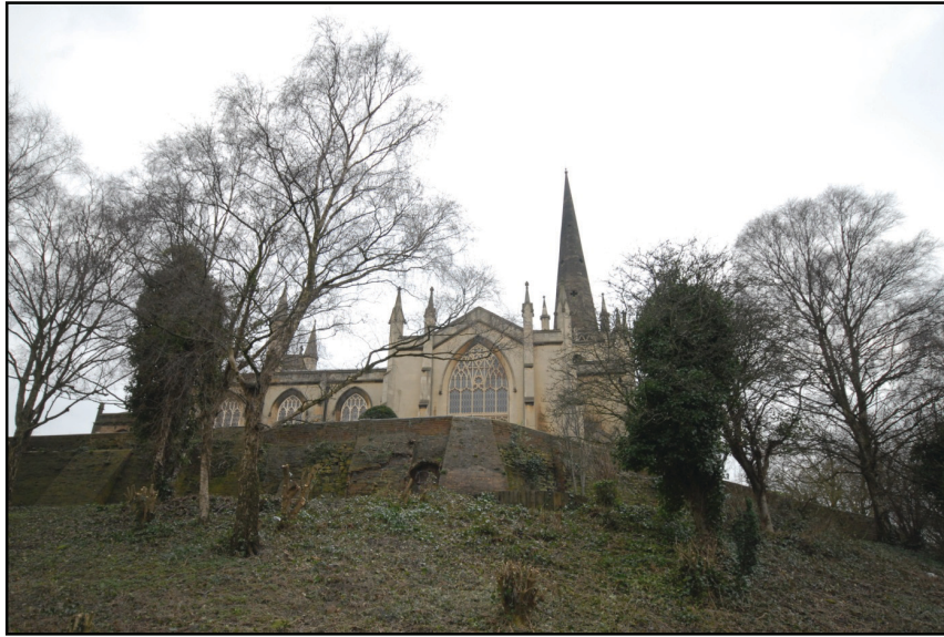
The central extent of the retaining wall, looking south Fig 17
