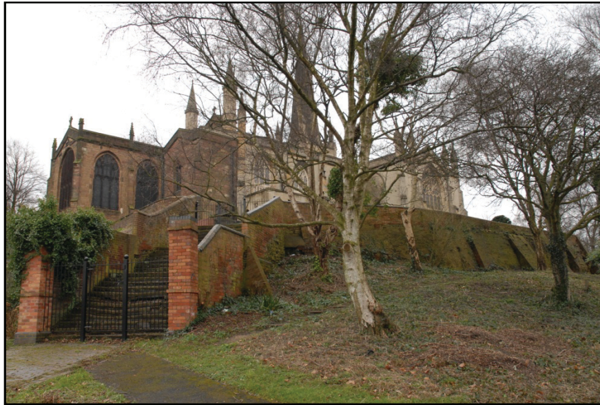
The eastern extent of the retaining wall, looking south-west Fig 15
