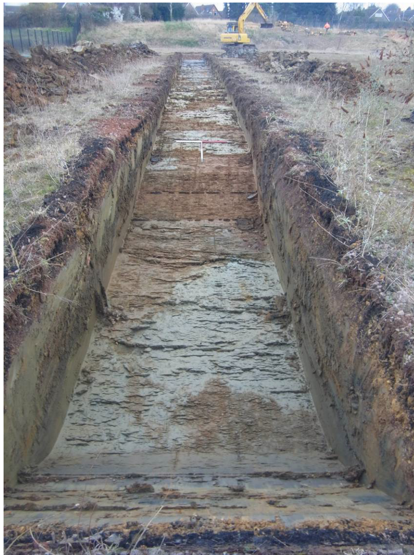
Trench 10, looking south-west
