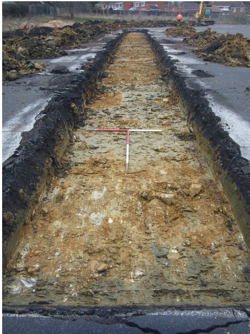
Trench 2, looking north-west Fig 9
