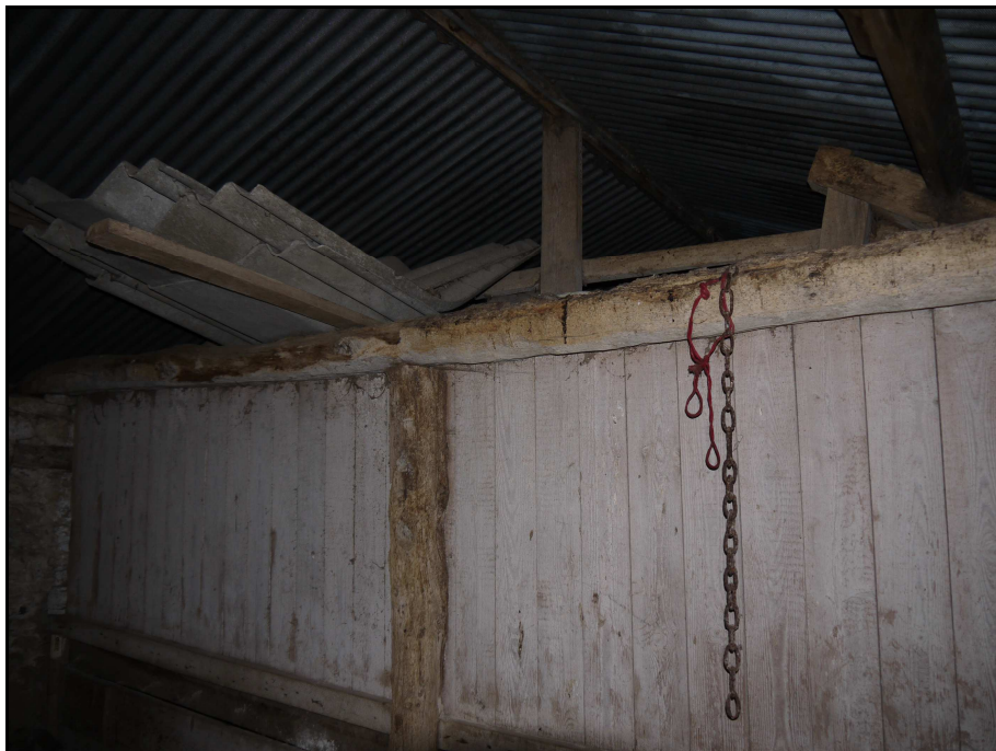
Original beam (C Middleditch) Fig 8
