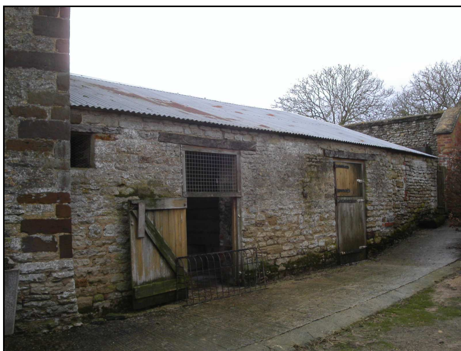
North-west elevation into courtyard (C Middleditch) Fig 3
