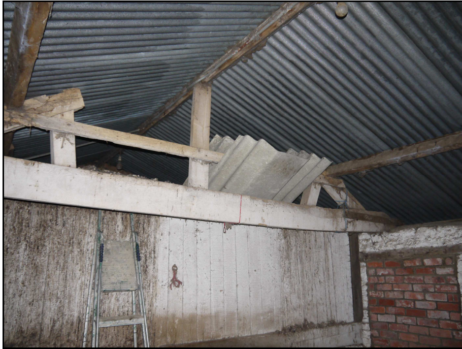
Remains of original truss and modern roof construction (C Middleditch) Fig 7
