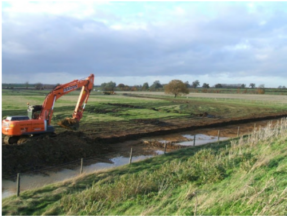
View of site during machine stripping, looking north-west
