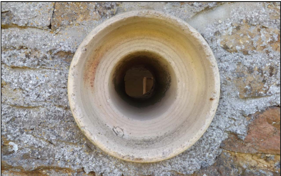
Detail of land drains used for ventilation throughout the ranges Fig 48
