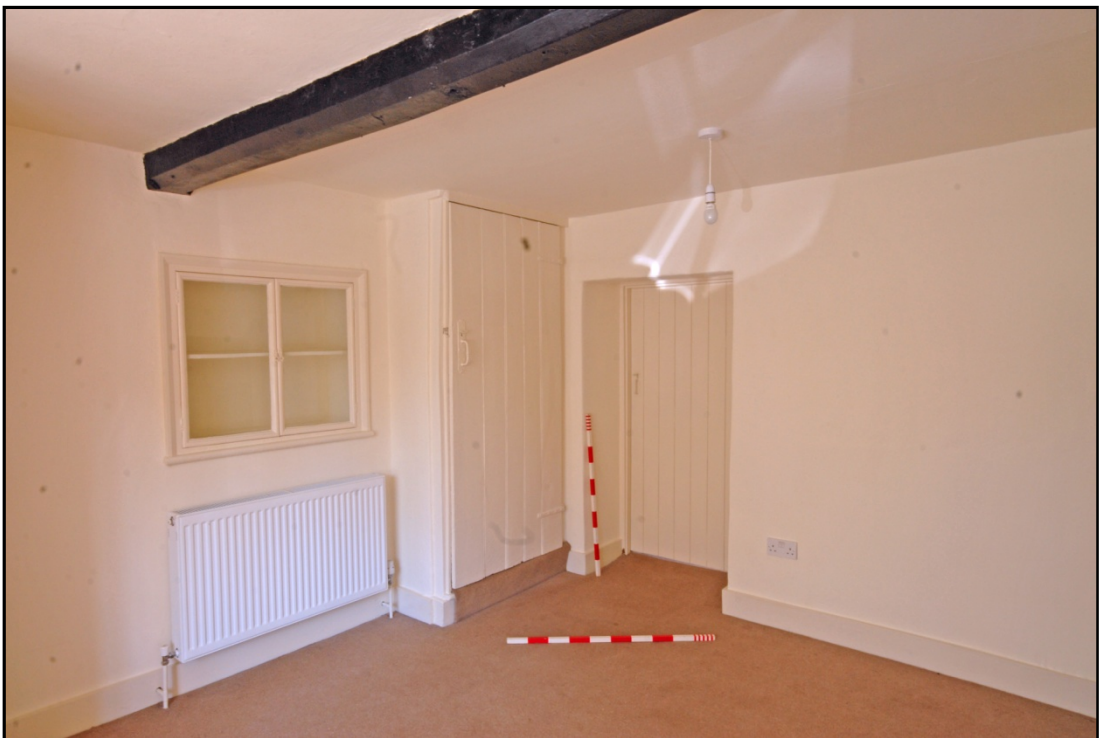
The Dining Room, with doors to the Bathroom and stairs, recessed cupboard to the left and beam with chamfered stops over Fig 24
