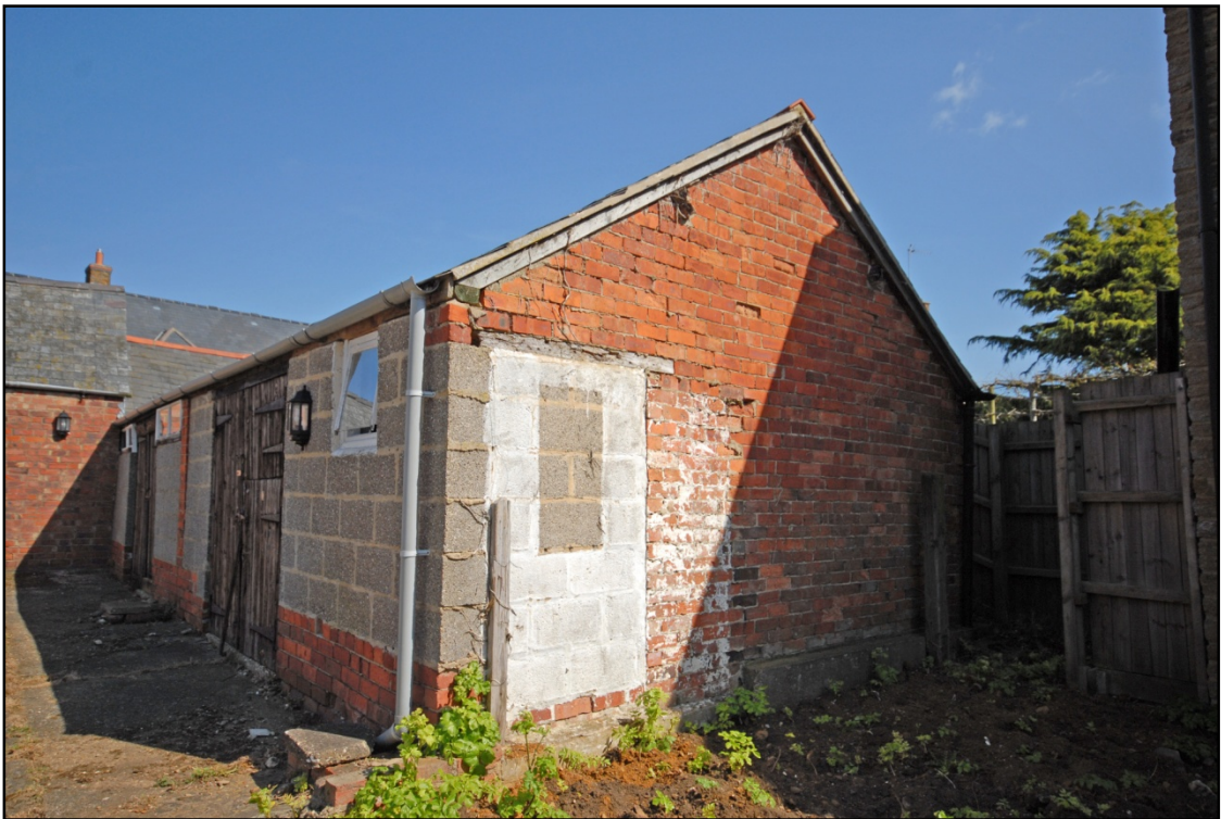
The east range, the south elevation, showing the blocked door Fig 60
