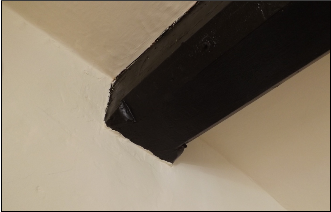
Detail of the Dining Room beam with chamfered stops Fig 25
