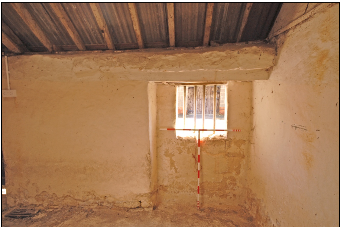
The blocked door in room G5, looking east. Note the beam over Fig 54
