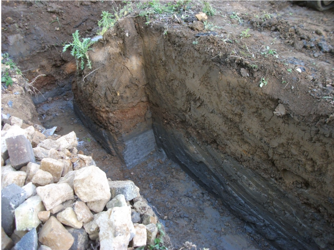
An excavated house foundation trench, showing the sequence of geological strata Fig 3
