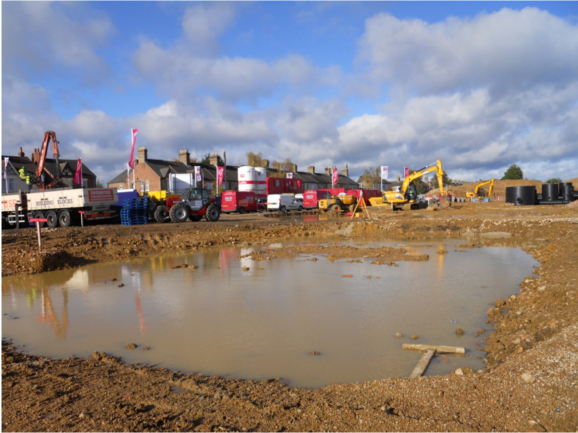
General view of the investigation area, looking west Fig 3
