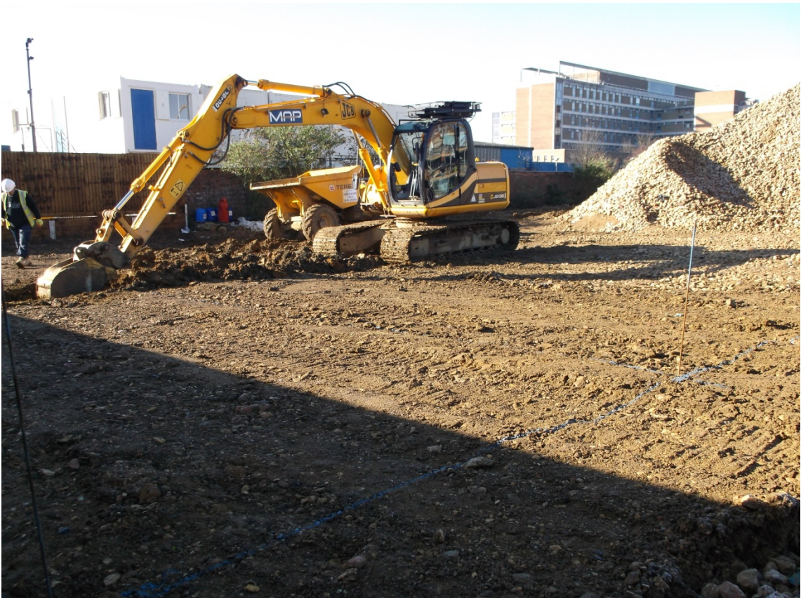
The groundworks in progress Fig 4
