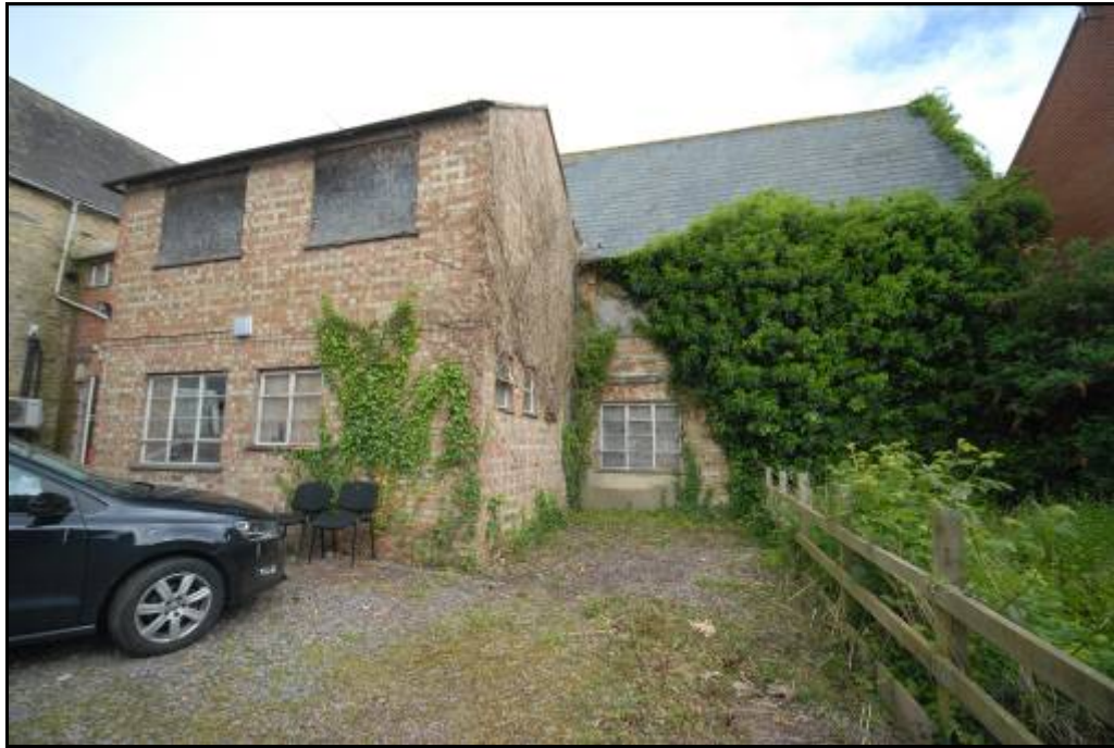
South elevation, looking north-west Fig 12
