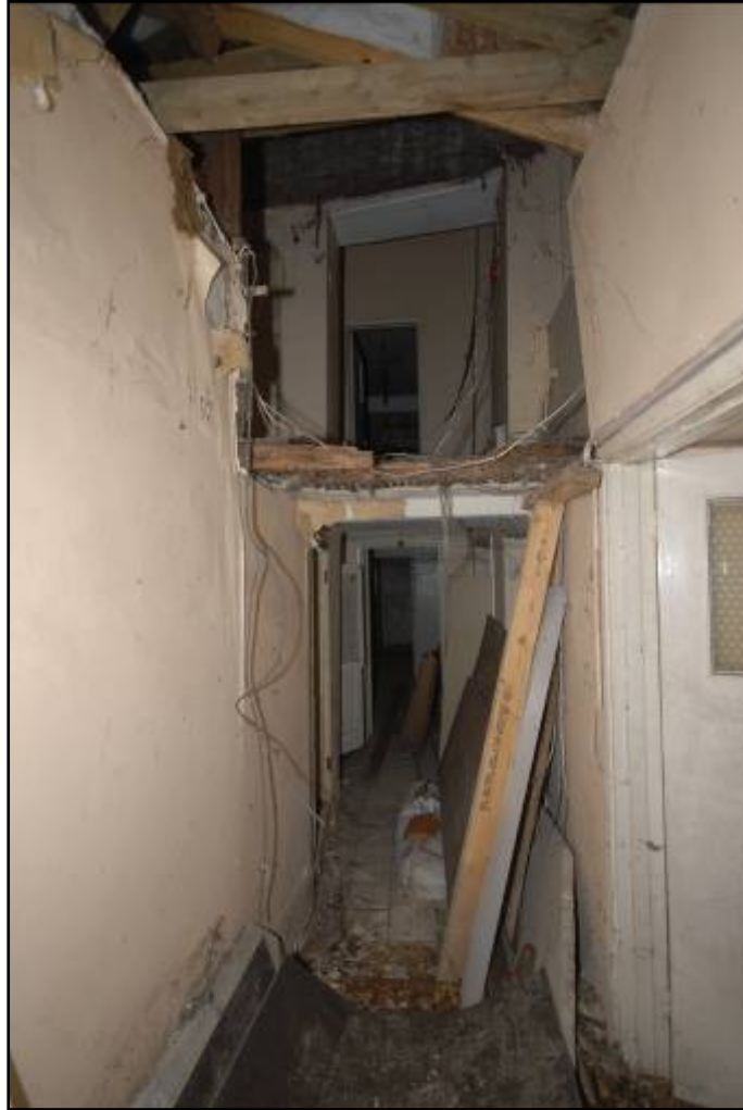
Hallway, looking east Fig 31
