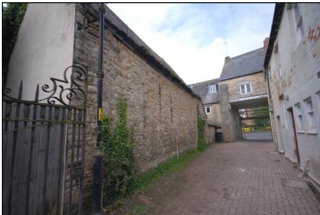
North elevation from Brewery Walk, looking south-west Fig 9
