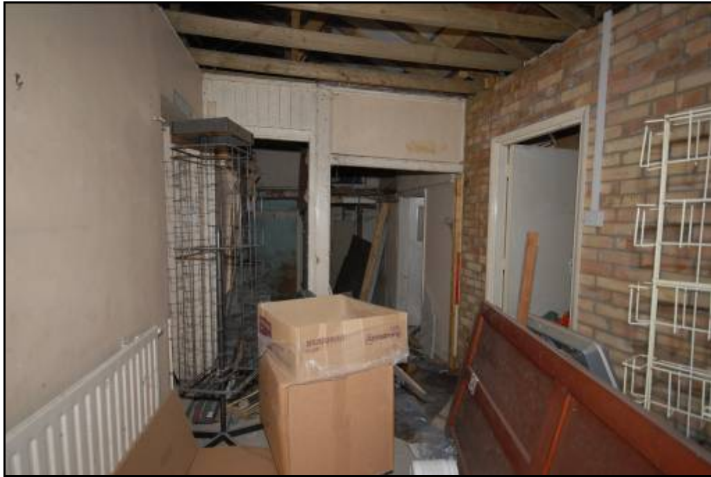
Room 2, looking east Fig 21
