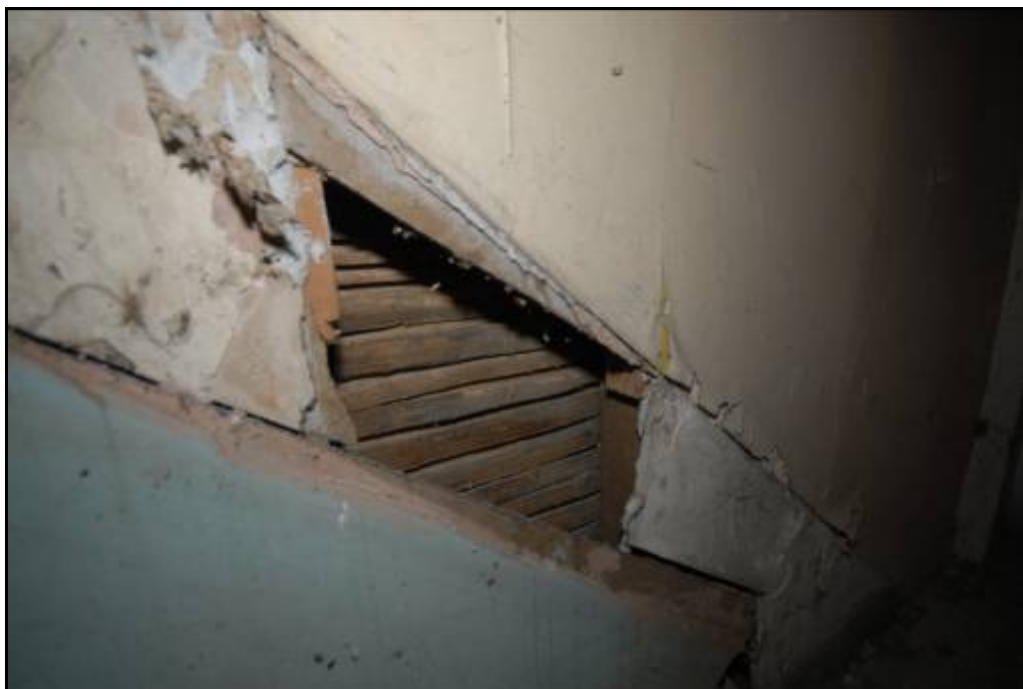
Lath and plaster showing in stud wall Fig 28
