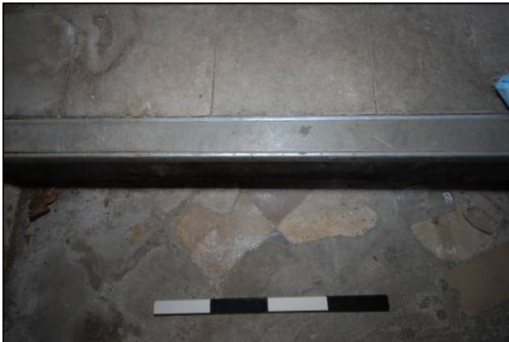
Original floor tiles showing underneath screed Fig 18
