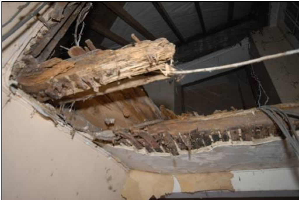
Lath and plaster construction of ceiling Fig 32
