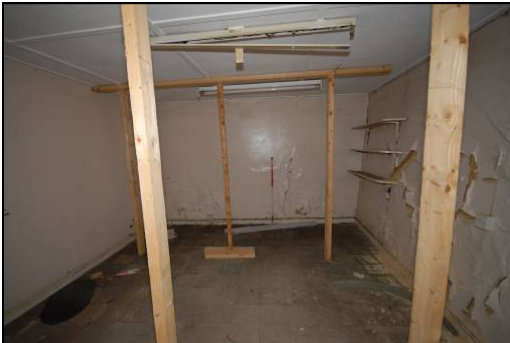
Room 11, looking north Fig 38
