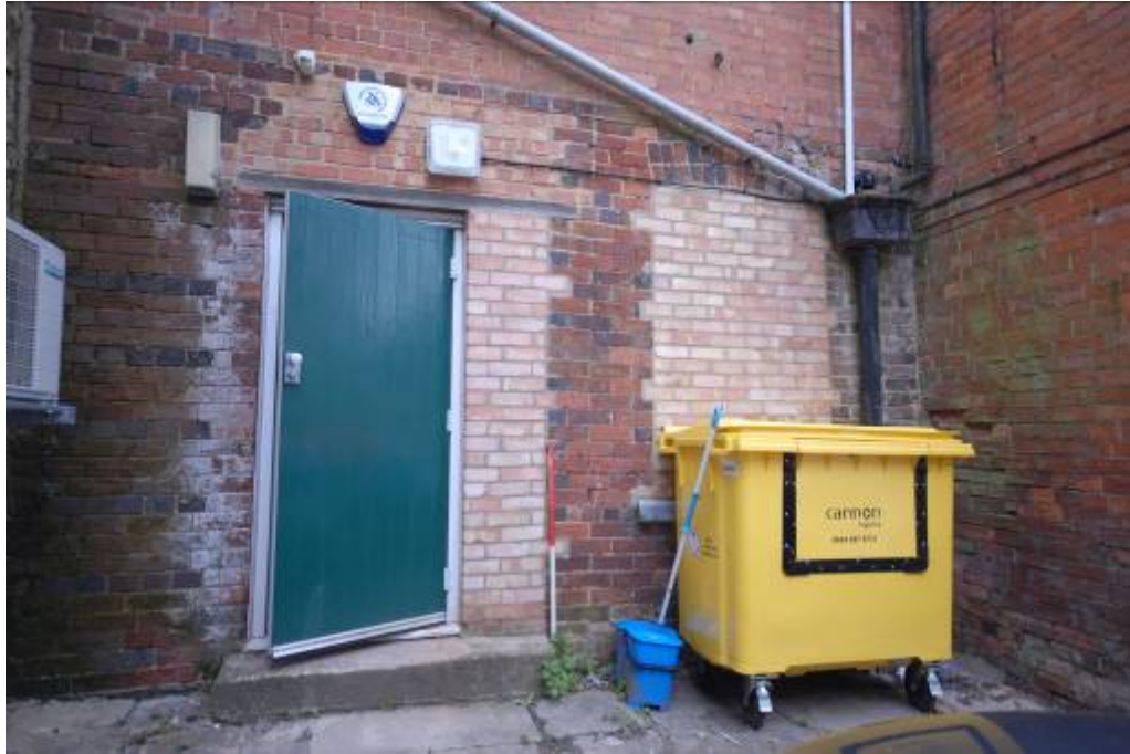
South elevation showing the door and window alterations, looking north Fig 14
