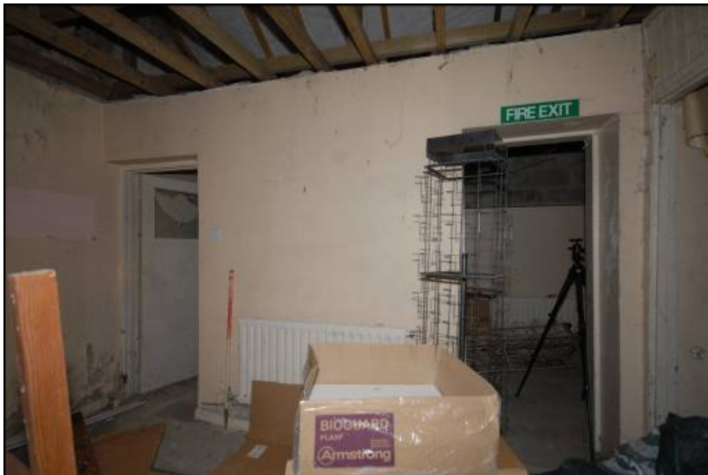
Room 2 with doors, looking north-west Fig 20
