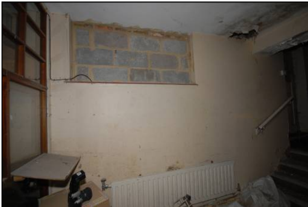
Blocked window in room 4 along northern wall Fig 24
