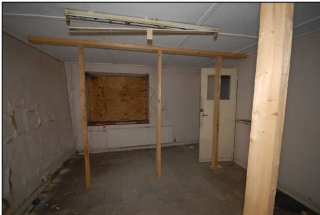
Room 11 with window, looking south Fig 40
