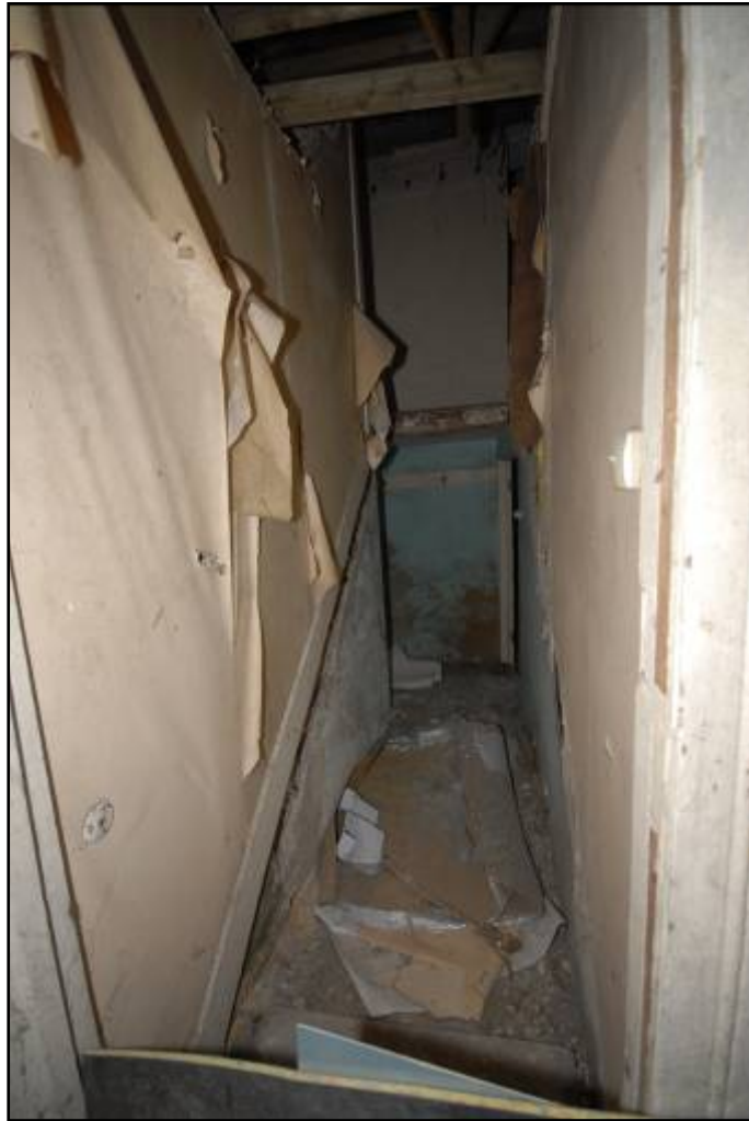
Stairwell after removal of stairs, looking east Fig 30
