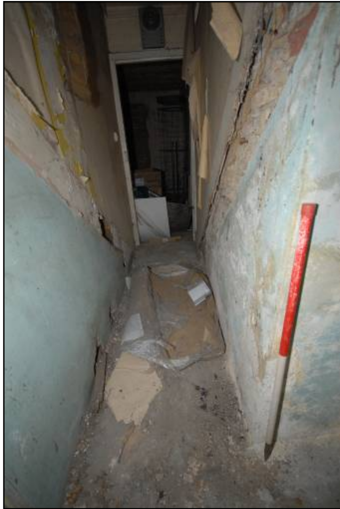
Cupboard under the stairs, looking west Fig 29
