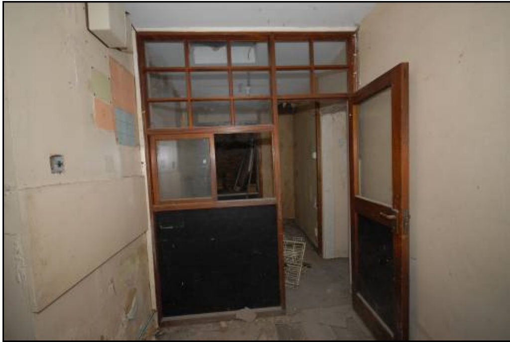
Wooden partition, looking east Fig 23
