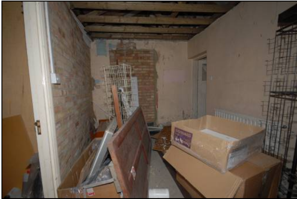
Room 2 with bricked-up door, looking west Fig 19
