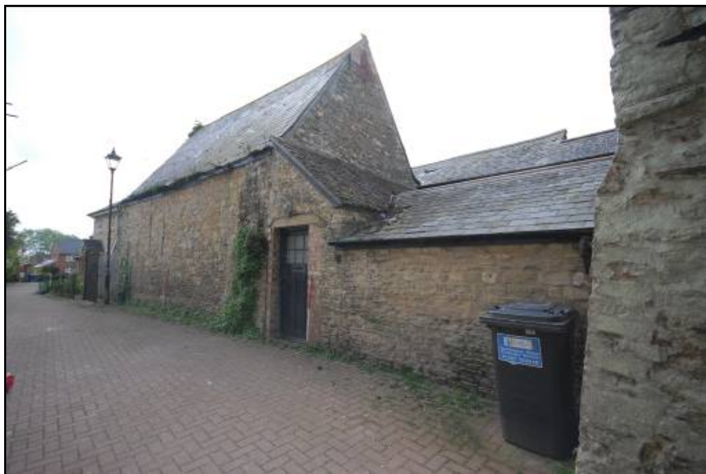
North elevation from Brewery Walk, looking south-east Fig 11
