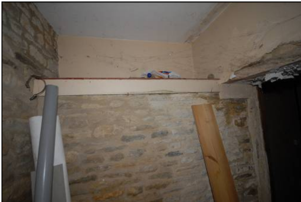
Exposed stonework with ledge, looking south Fig 26
