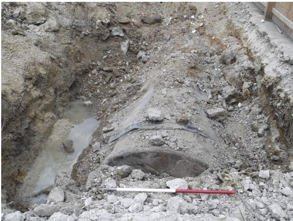
Fuel tank removal, looking north
